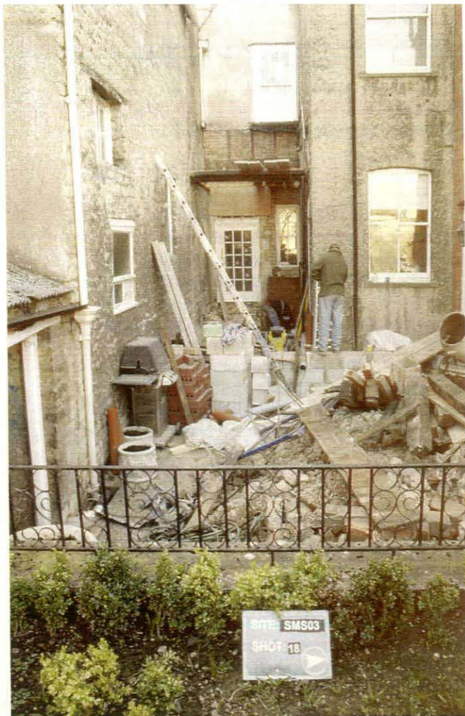
Plate 4 - General view following the removal of the porch, looking west
