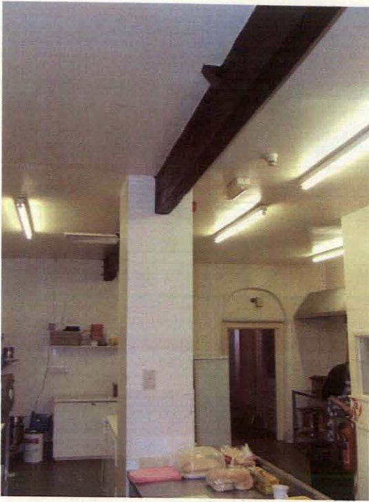
Plate 25 Former Drill Hall, Room B, looking
