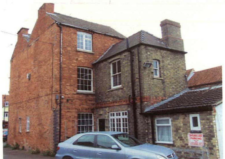
Plate 4 North and west elevations 26 Southgate, showing Phase 2 and 3 extensions, looking southeast
