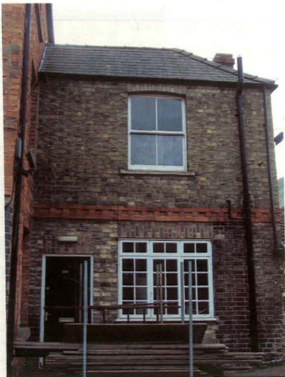
Plate 3 North elevation, 26 Southgate, Phase 2 addition, looking south
