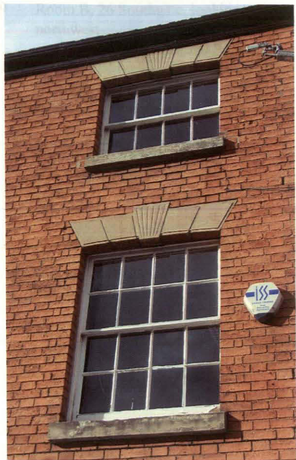
Plate 6 Upper storey windows, 26 Southgate, looking west
