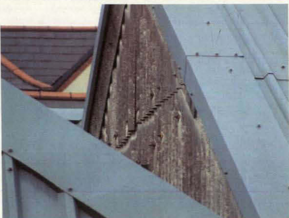
Plate 24 Former Drill Hall, west elevation above roofs, looking north
