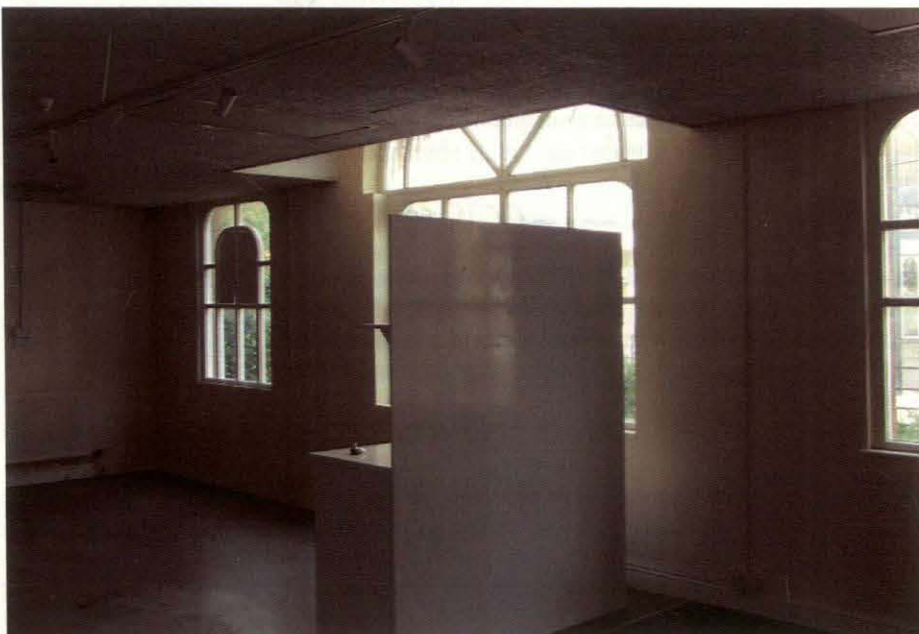
Plate 30 Former Drill Hall, Room G, windows, looking northwest
