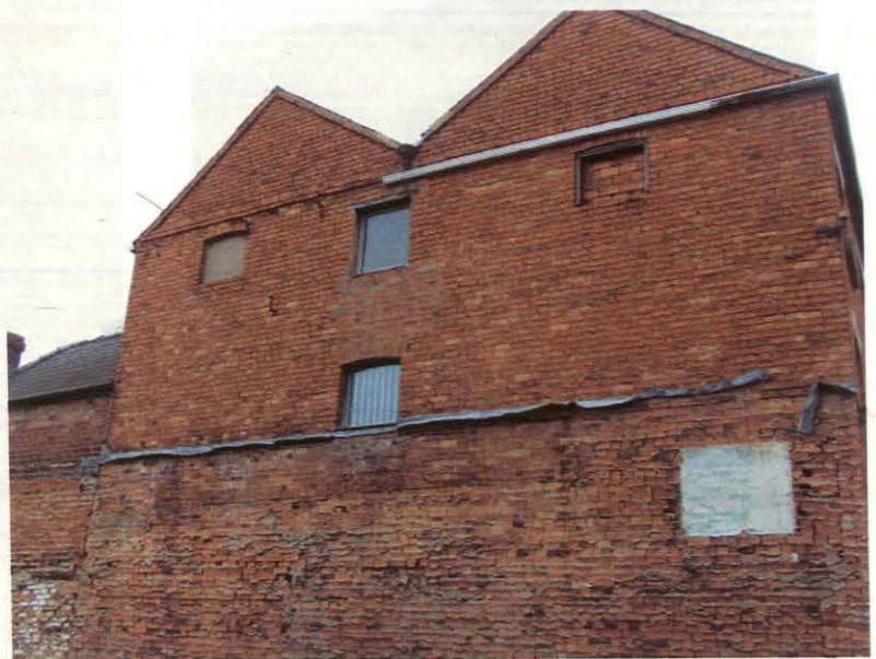
Plate 2 South elevation, 26 Southgate, looking northwest
