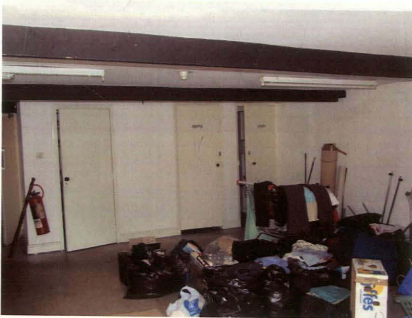
Plate 27 Former Drill Hall, Room F, looking northwest
