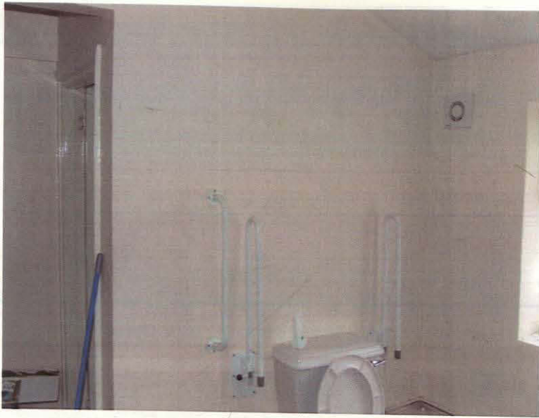
Plate 13 Room F, 26 Southgate, showing partition wall, looking northwest
