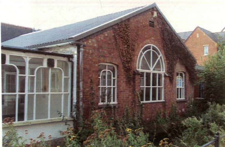
Plate 23 Former Drill Hall, north elevation, looking west
