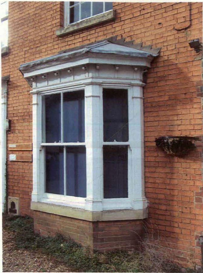
Plate 5 Bay window, 26 Southgate, looking southwest
