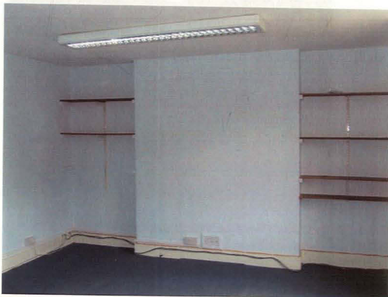
Plate 16 Room H, chimney breast, 26 Southgate, looking north
