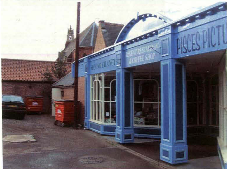
Plate 22 Former Drill Hall, east façade, looking southwest
