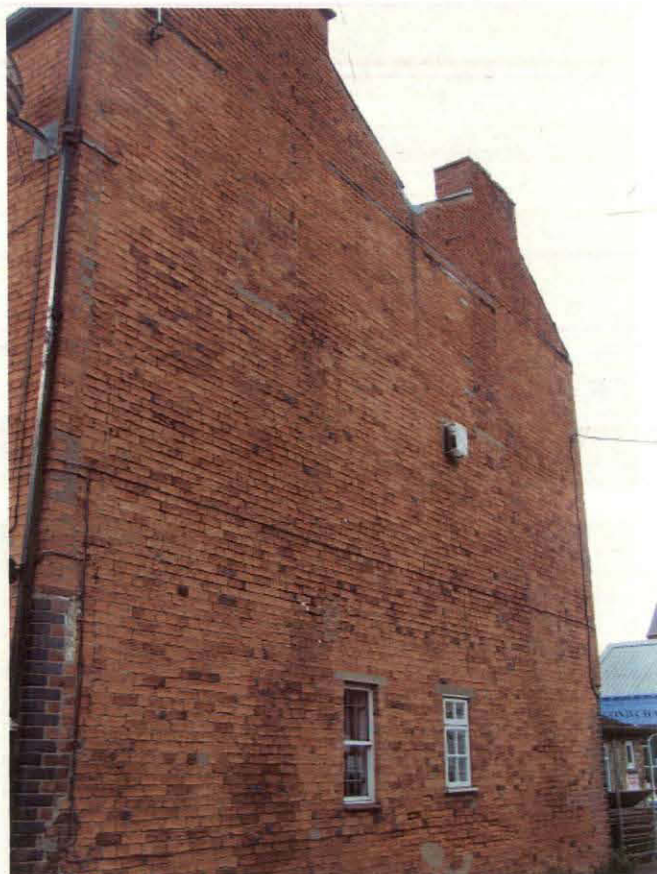
Plate 7 North elevation, 26 Southgate, looking southwest
