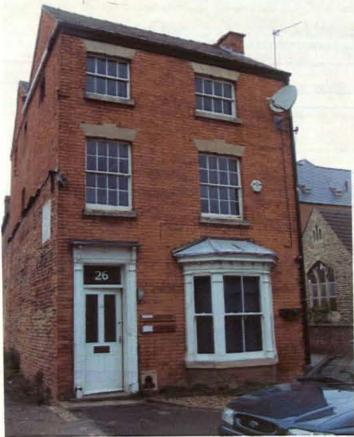
Plate 1 General view, 26 Southgate, showing east elevation, looking west
