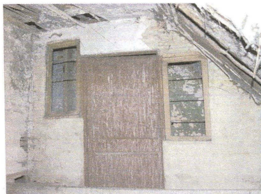
Plate 5 Stud partition between Rooms S1 and S2
