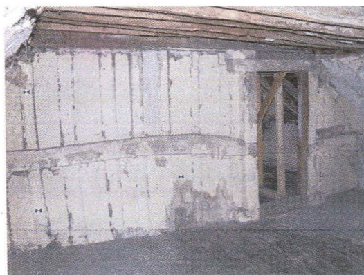
Plate 9 Tie-beam partition between Rooms S4 and S5
