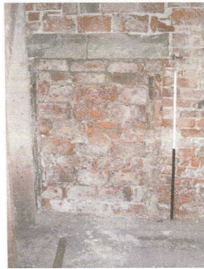
Plate 1 Blocked fireplace in Room G2 (scale 1.0m)
