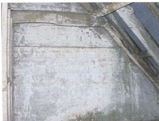
Plate 4 Stringcourse in internal wall of Room S2
