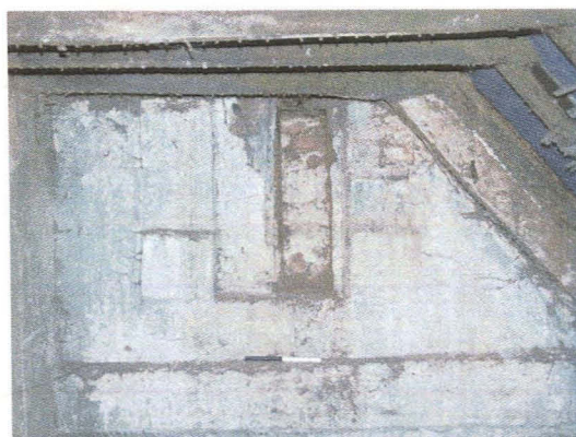
Plate 6 Blocked window in Room S3 (Scale 0.20m)
