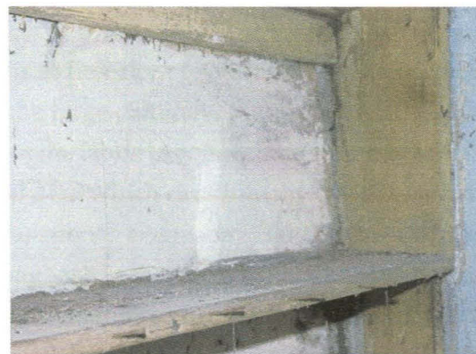
Plate 12 Continuation of stringcourse in Room G6
