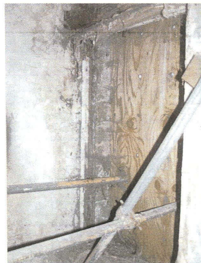
Plate 3 Window cut by internal wall in Room F2
