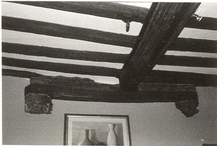
Plate 13 Bracket Supporting Beam, Bar North of Archway
