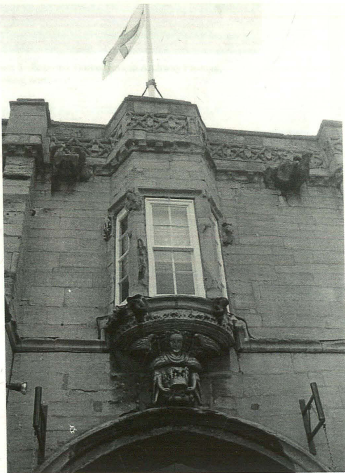
Plate 3 Central Oriel Window and Angel Corbel, Hotel Frontage, looking east
