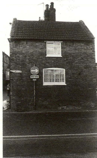
Plate 26 Eastern Elevation of East End Store Room, North Wing, looking west
