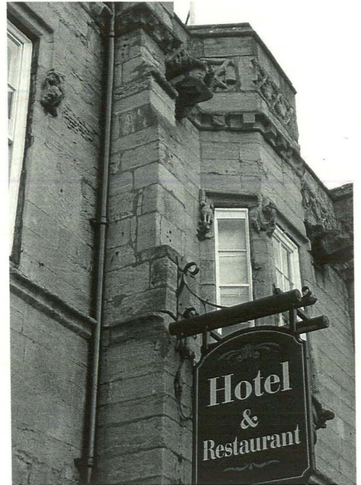
Plate 2 Gargoyles and Decoration, Hotel Frontage, looking southeast
