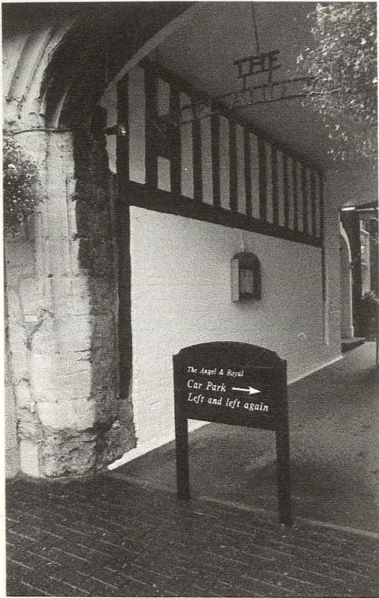
Plate 5 Exposed Timberwork in Archway Passage, looking northeast
