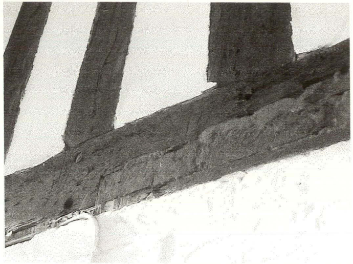
Plate 6 Joiner's Marks on Exposed Timbers in Archway Passage, looking northwest
