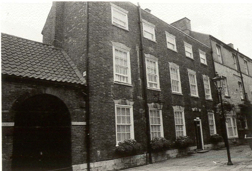
Plate 43 North Side of Three-storey Brick House, South Wing, looking southwest
