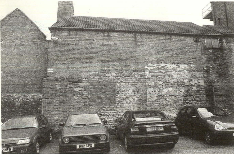
Plate 28 Two Storey House, North Side of North Wing, looking south
