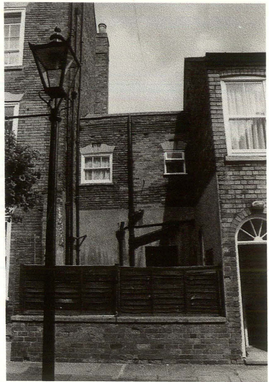
Plate 23 Narrow 2-Storey Building, North Wing, looking north
