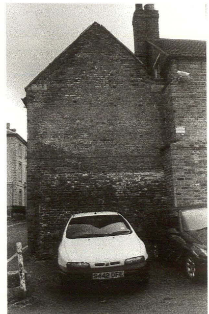
Plate 27 North Side of East End Store Room, North Wing, looking south
