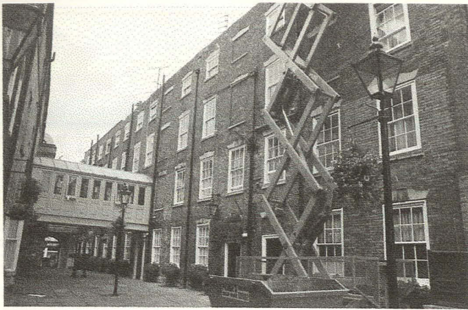
Plate 22 General View of North Wing, South Elevation, looking northwest
