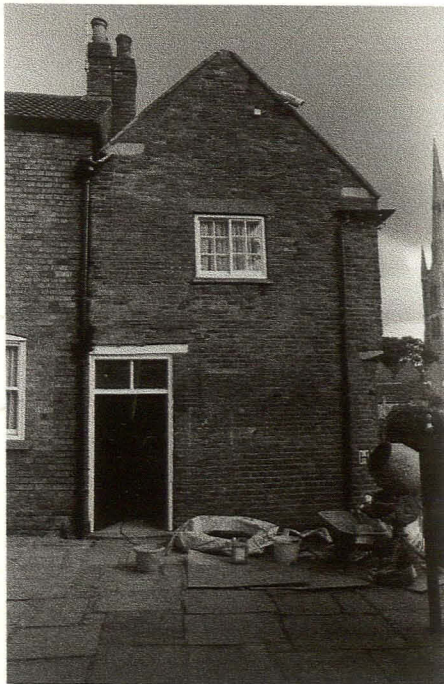
Plate 25 East End Store Room, North Wing, looking north
