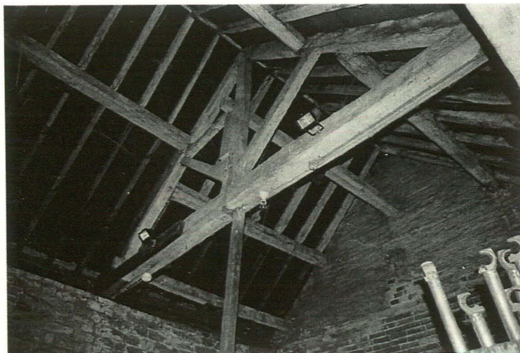
Plate 46 King Post Roof Truss in Stable Range, South Wing
