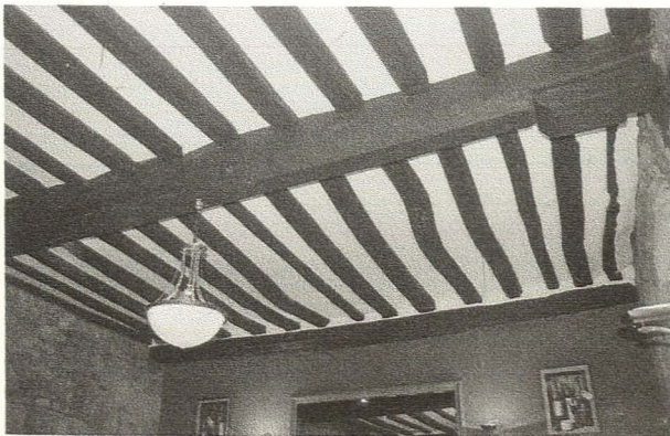
Plate 9 Roof Timbering, Bar South of Archway
