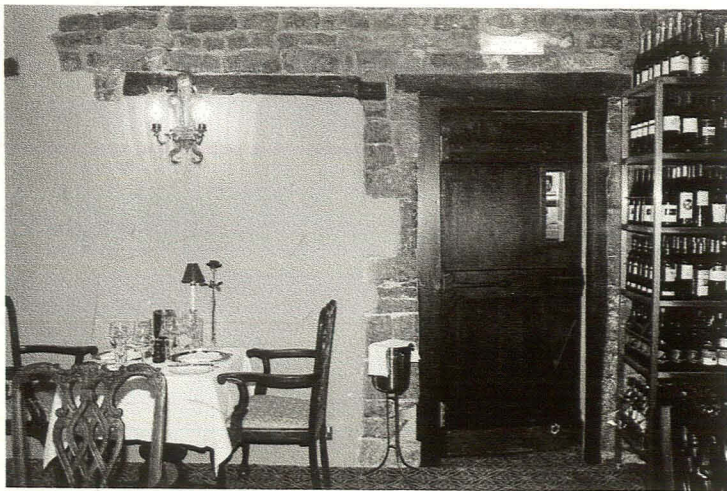
Plate 20 Timber Lintel Marking Possible Blocked Doorway, First Floor Restaurant
