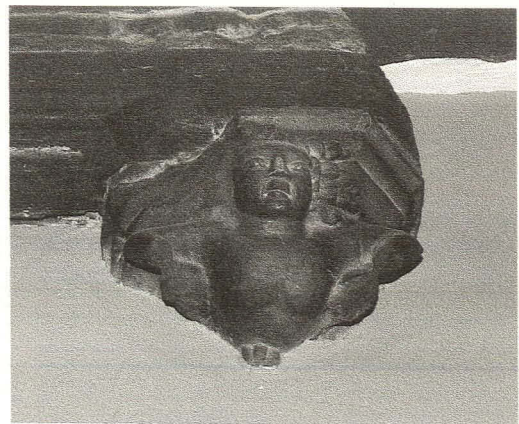
Plate 14 Corbel Supporting Bracket, Probable Reused Misericord
