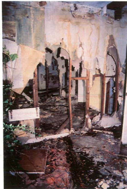
Plate 14 – View of the first floor, looking southwest
