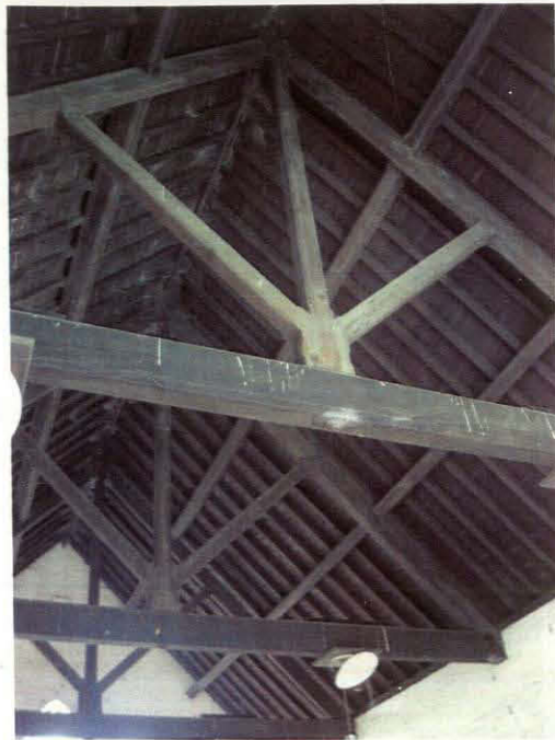
Plate 4 – Roof detail in the chapel
