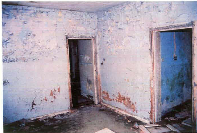
Plate 8 – Room A, looking southwest
