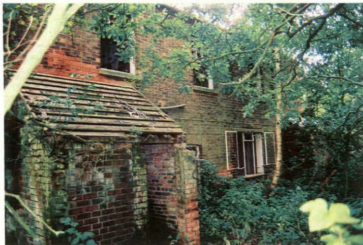
Plate 6 – The west façade of Rowan House
