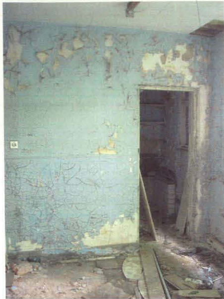
Plate 10 – Rooms B and D, looking west
