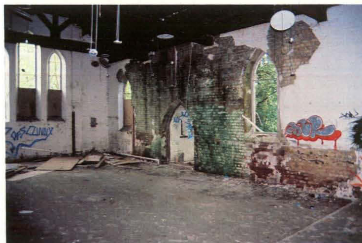
Plate 3 – Interior view of the chapel, looking northwest
