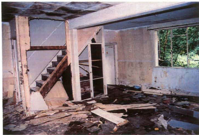
Plate 11 – Room E, looking south
