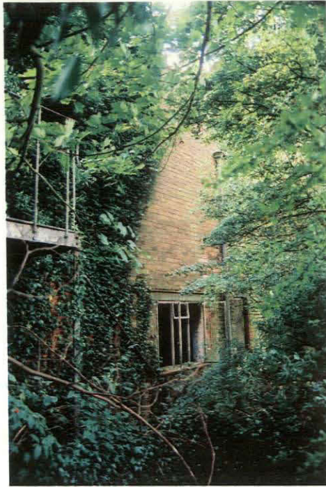
Plate 7 – The north façade of Rowan House
