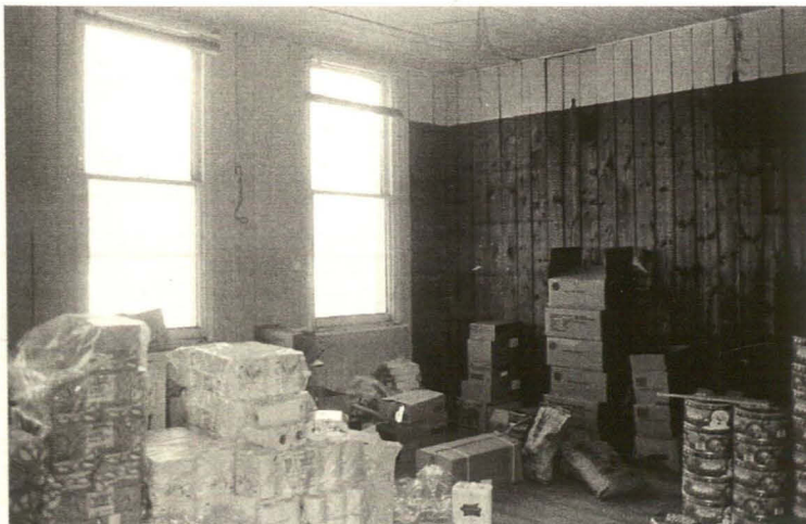
Plate 15 Co-Operative Store, Upper Floor, main storeroom showing panelling, looking northeast
