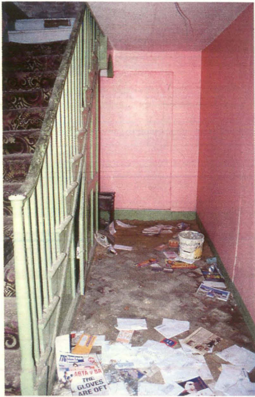
Plate 5 Central Stairwell, looking south
