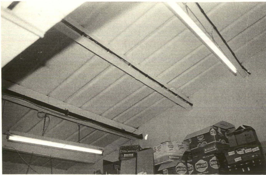
Plate 13 Sheet Steel Roof of Recent Extension to Store, ground floor, looking southwest
