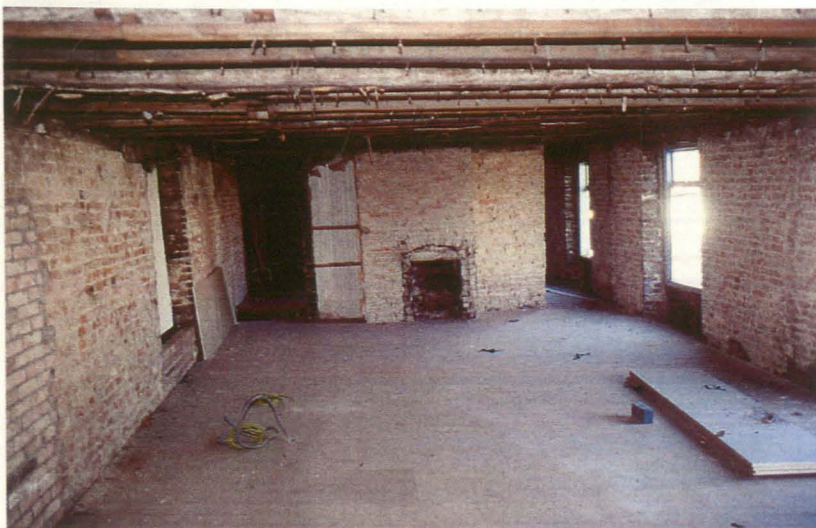
Plate 8 Upper Floor, area of eastern section of housing terrace, looking west
