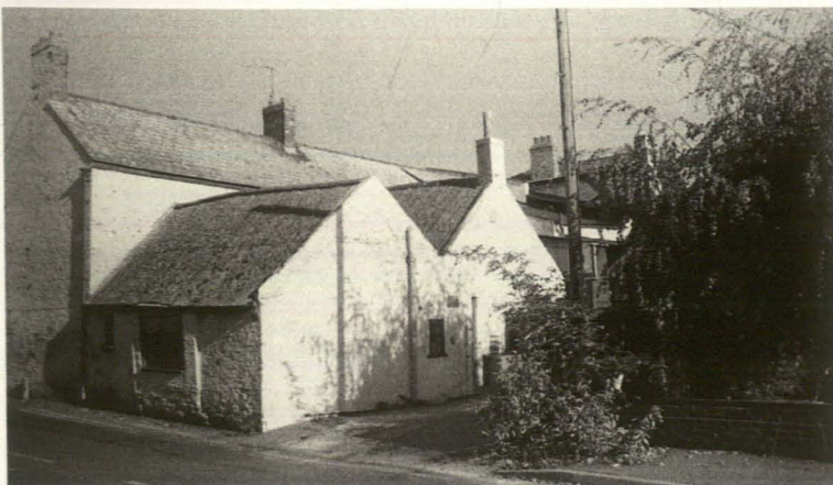
Plate 4 Single Storey Buildings to rear of West End Shop and Stairwell, looking northeast
