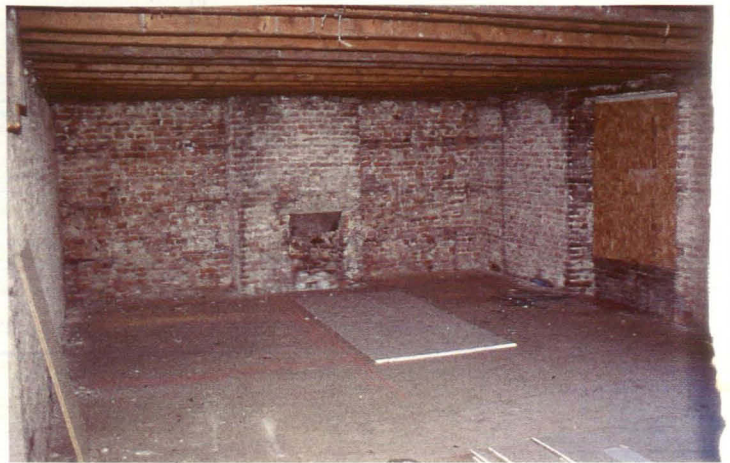
Plate 6 Upper Floor, area of West End Shop and Stairwell, showing fireplace and scars of removed shelving, looking west
