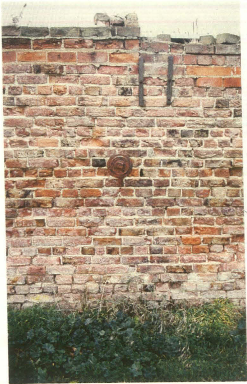
Plate 9 RSJ in southeastern wing
