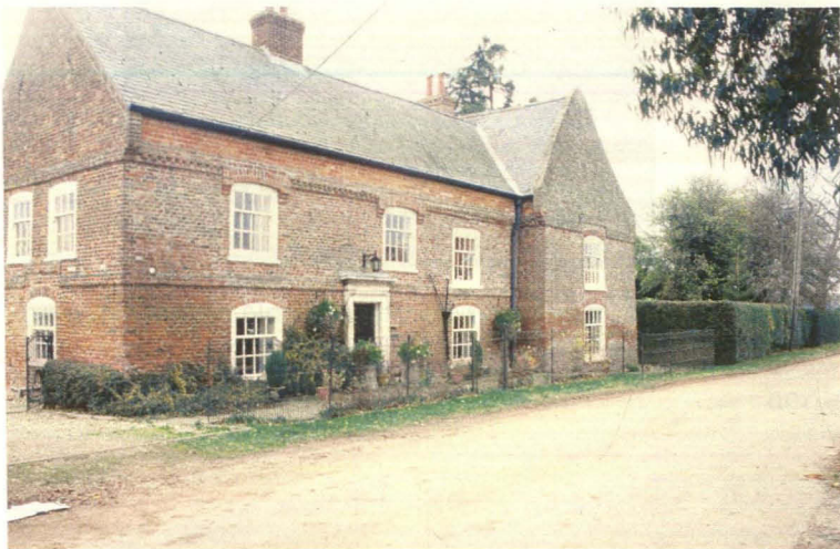
Plate 2 Ivy House, looking west
