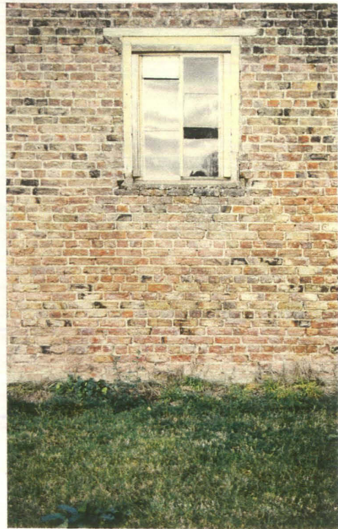
Plate 6 Window in southeastern gable of main barn, looking northwest
