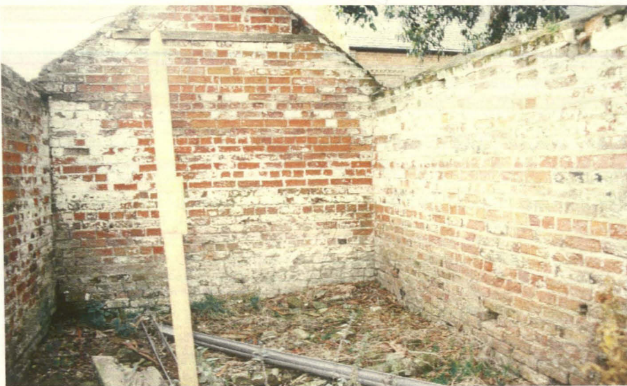
Plate 26 Interior of southwestern room in northwestern wing, looking southwest
