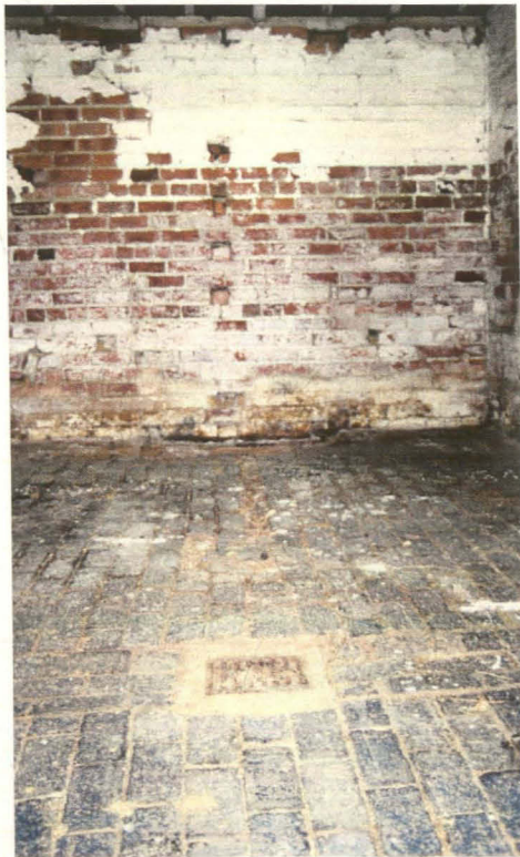
Plate 16 Brick flooring in northeastern stable compartment
