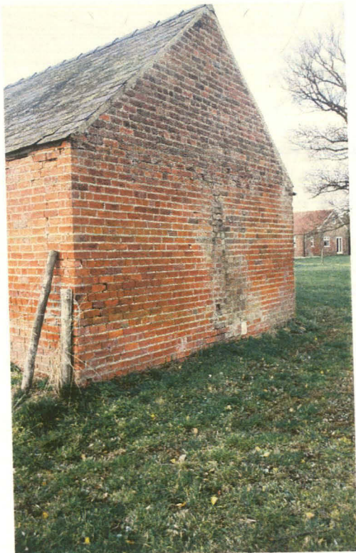
Plate 11 Northeastern gable of stable block, looking southwest
