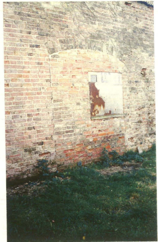
Plate 20 Blocked arch and boarded window-main barn-northeastern elevation, looking southwest
