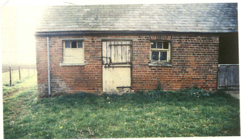
Plate 13 Northeastern compartment of stable block, looking southeast
