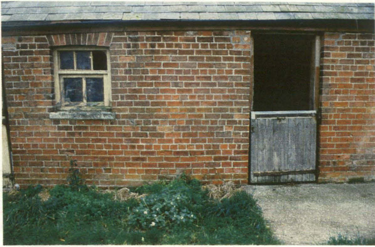
Plate 14 Central compartment of stable block, looking southeast
