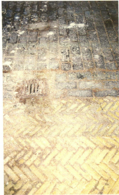
Plate 17 Brick flooring in central stable compartment
