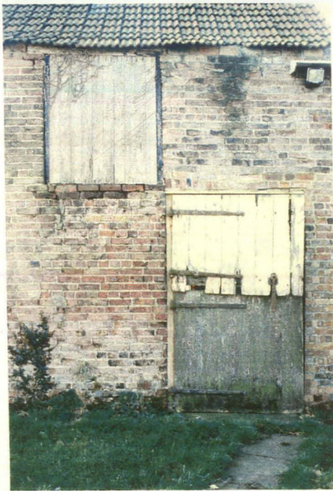
Plate 19 Dutch door and boarded window- main barn, looking southwest
