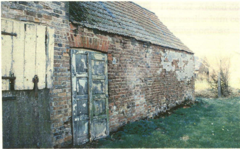
Plate 18 Northeast elevation of northeastern wing, looking west
