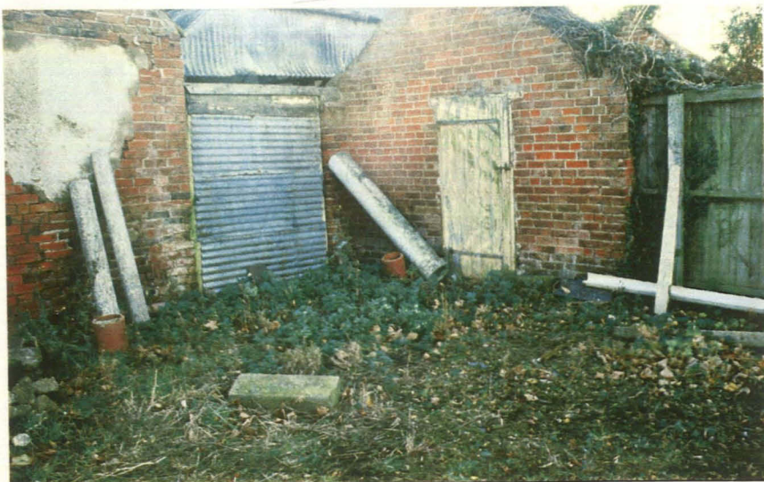
Plate 24 Northeast gable of northwestern wing, looking south
