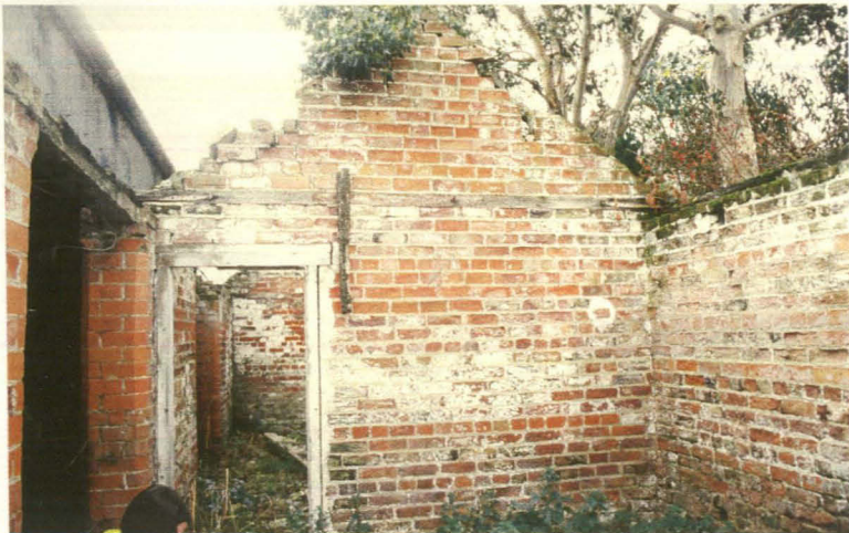
Plate 27 Internal divide in northwestern wing, looking southwest
