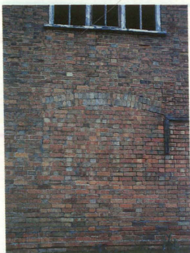
Plate 5 Northern elevation, blocked ground floor window, looking south
