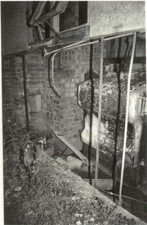
Plate 20 Chimneys, showing straight joins, looking northeast
