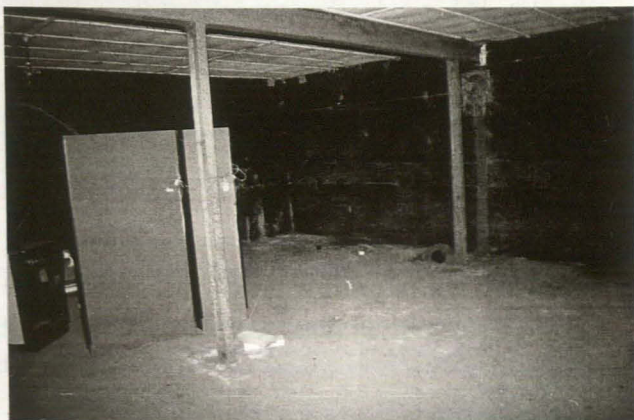
Plate 14 Interior, west room, showing RSJ beam and supports, looking southwest
