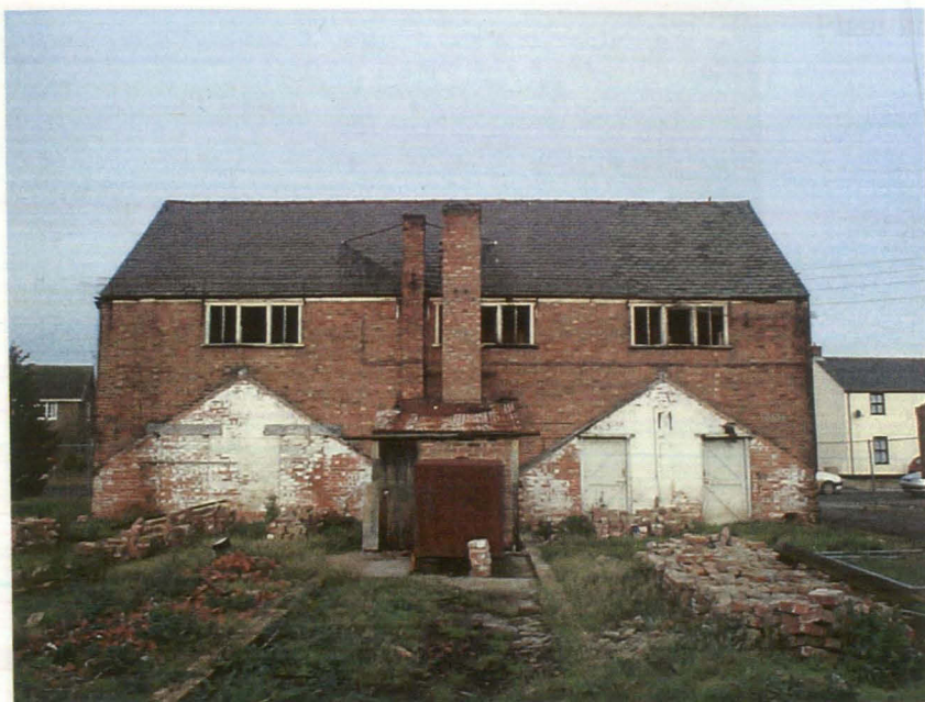
Plate 8 South side of building, showing scars of removed glasshouses, looking northeast
