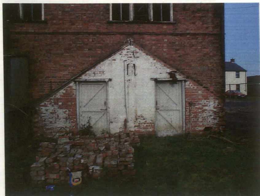
Plate 10 Southern elevation, east side, showing doors and glasshouse scar, looking north
