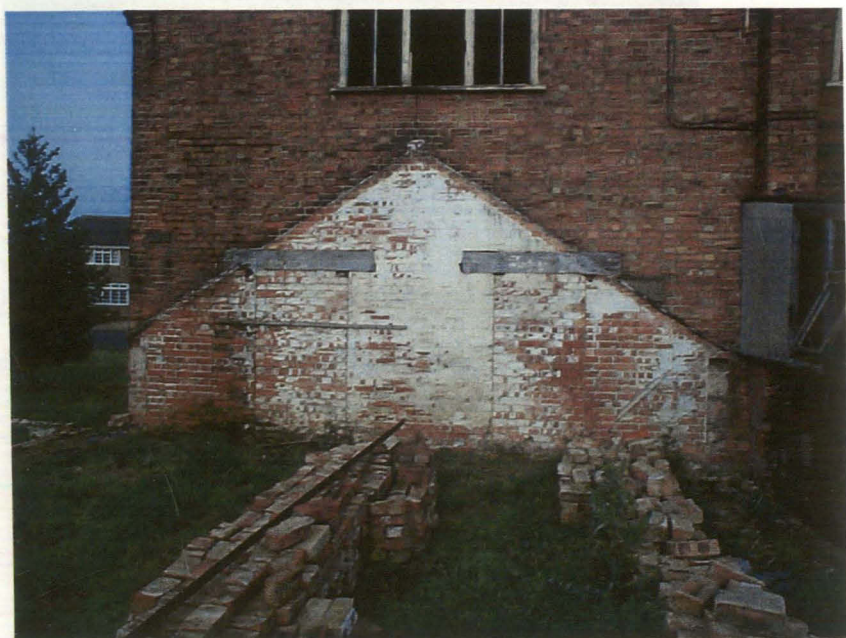
Plate 9 Southern elevation, west side, showing blocked doors and glasshouse scar, looking north
