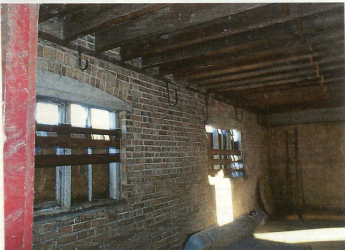
Plate 13 Interior, east room, north side, showing pipe suspension hooks, looking east
