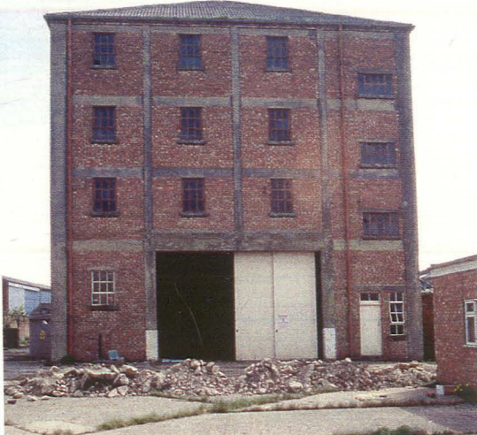
Plate 2 North elevation of Warehouse 1, showing loading access
