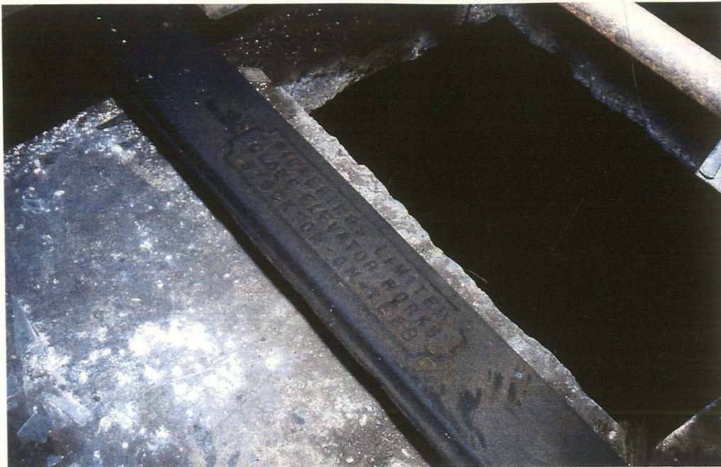
Plate 23 Metal plate of sack hoist with 'PICKERING LTD GLOBE ELEVATOR WORKS STOCKTON-ON-TEES embossed, Warehouse 2
