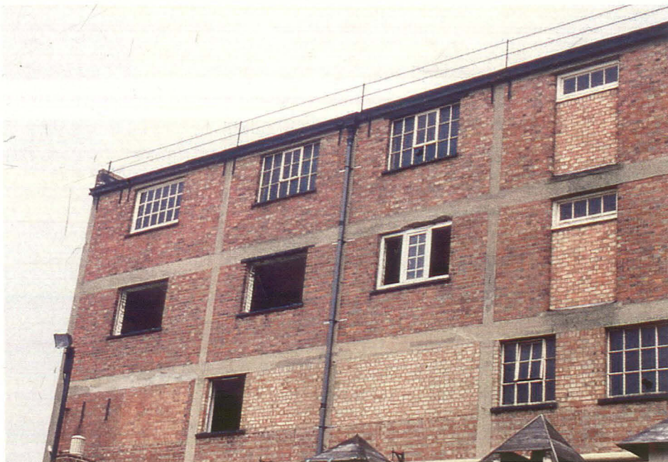
Plate 19 Brick blocking on third storey and metal railing around roof, Warehouse 2
