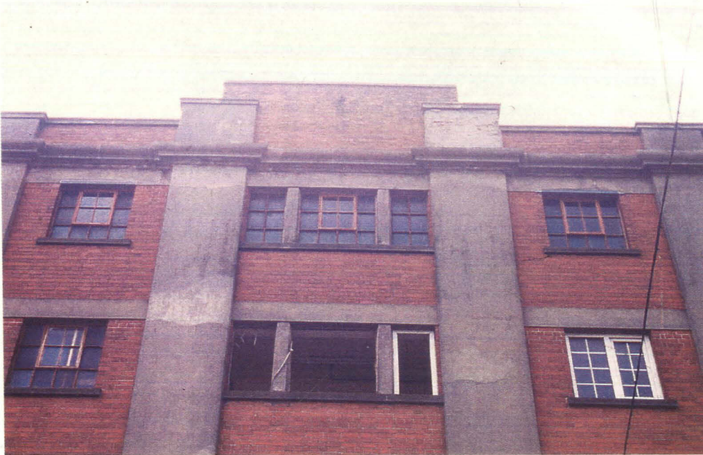
Plate 20 Brick architrave, and top of central bay in northern elevation, Warehouse 2
