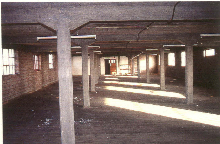
Plate 25 General view of third floor, Warehouse 2
