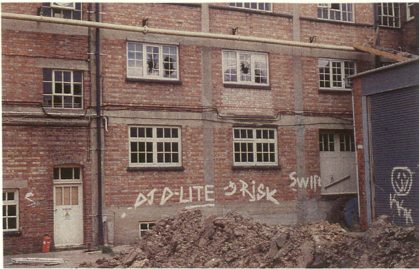
Plate 17 Detail of windows and wooden doors in south elevation, Warehouse 2
