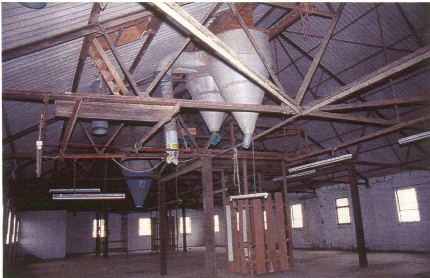
Plate 12 Third floor, showing silos and metal roof trusses, Warehouse 1
