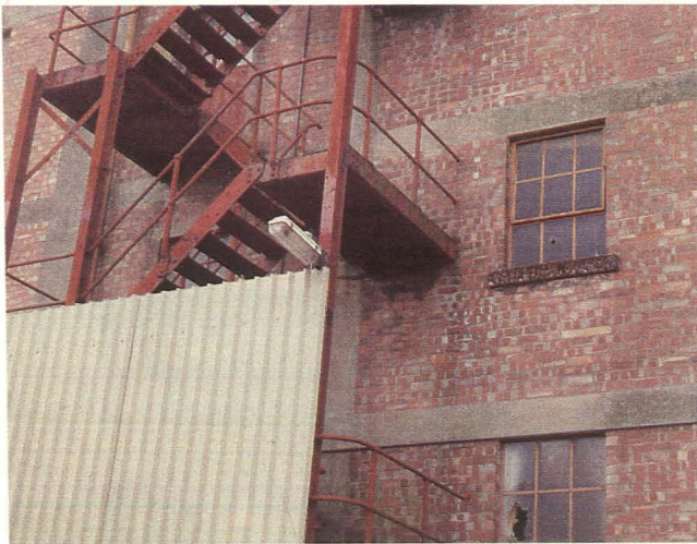
Plate 6 Detailed view of corrugated steel around base of external staircase, Warehouse 1
