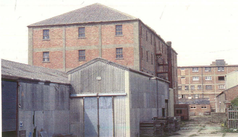
Plate 4 South elevation of Warehouse 1
