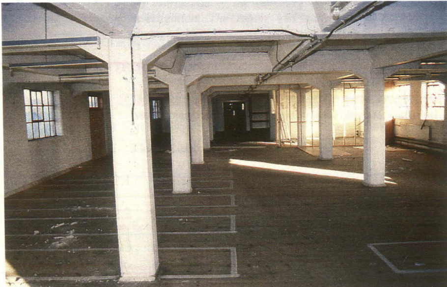
Plate 24 General view of second floor, Warehouse 2
