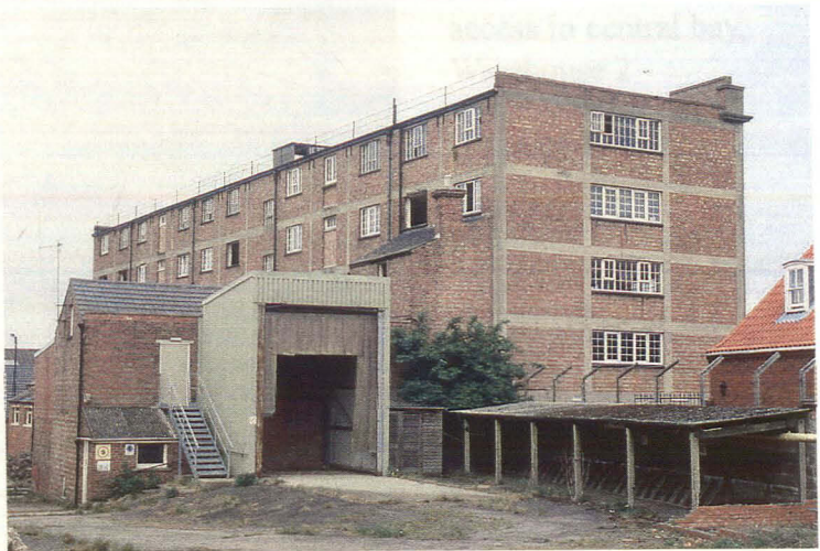
Plate 15 Eastern elevation of Warehouse 2/Stells Lane
