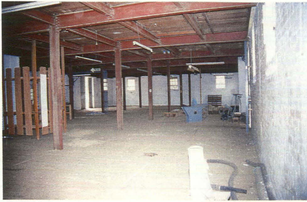
Plate 9 Interior of ground floor, Warehouse 1
