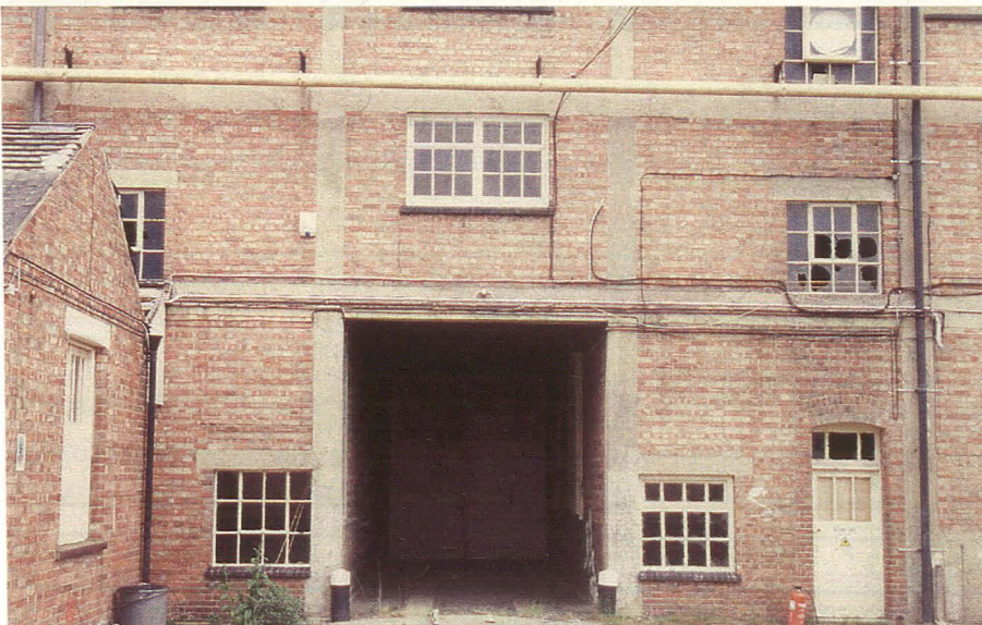
Plate 18 Drive-in access in central bay, Warehouse 2
