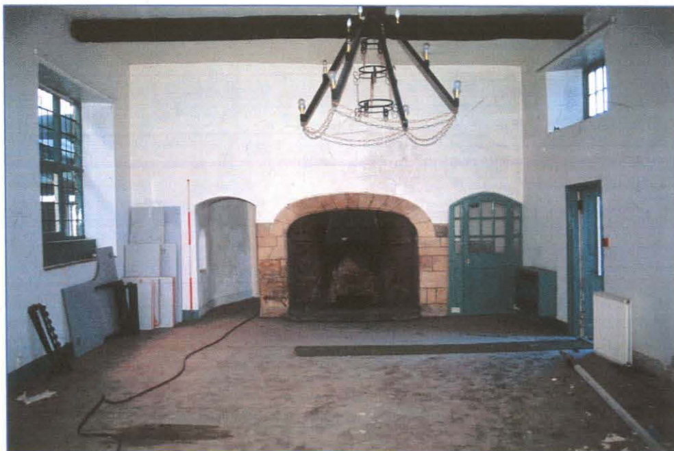
Plate 24: (038) Room 2. In the north wall is a large 18 th century basket arched fireplace with integral moulded stone surround and buttresses over an integral stone slab. There is an arched recess to the east of the fireplace with a half glazed nine pane door flanked by narrow three light sashes. The arch to the west passes through a former oven set into the corner of the building with an external curved wall. Looking north.
