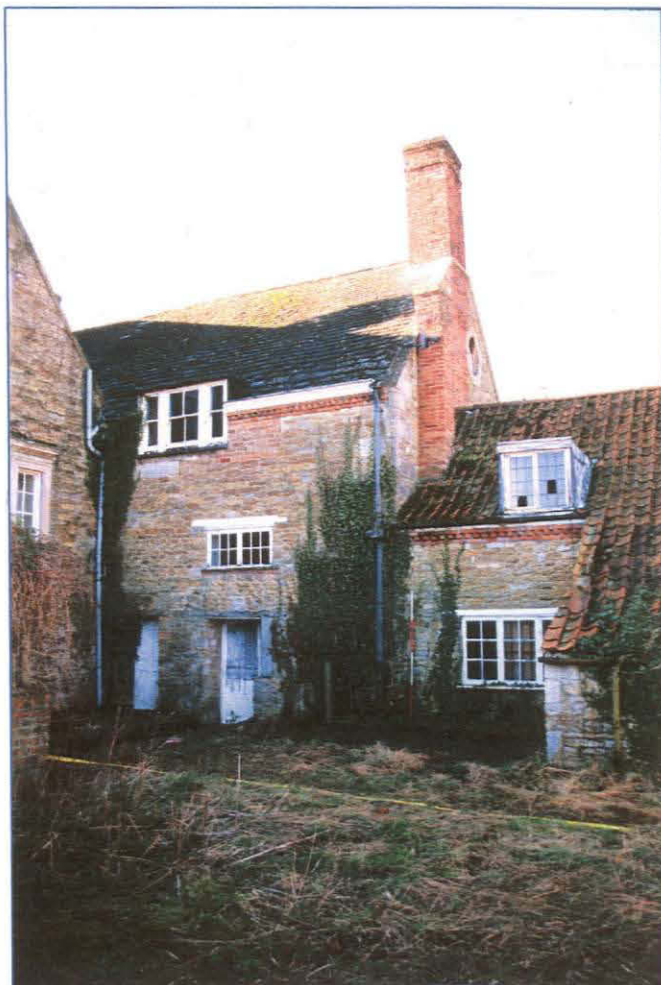
Plate 4: (013) The eastern elevations of the Eastern Range, detailing remodelling at the eaves and the insertion of dormers into the roof. Looking south-west.
