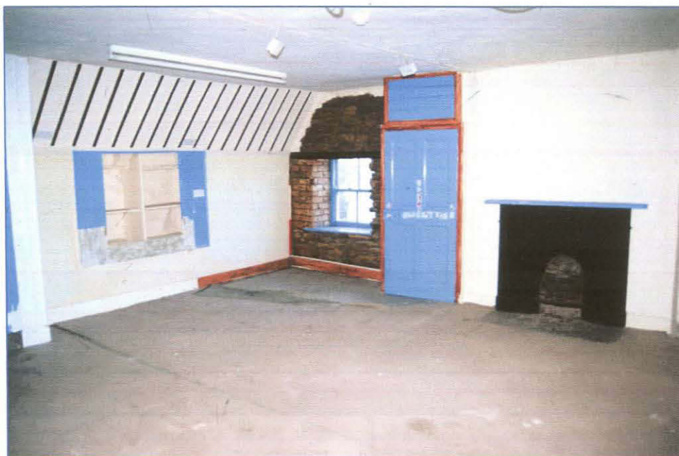
Plate 22: (079) Room 13, on the first floor of the Eastern Range. Set into the chimney breast on the northern wall is a 19 th century cast iron arched bath grate with a plain stone mantel and pillars. The door leads to Room 14 down a short flight of stairs. Looking north-west.
