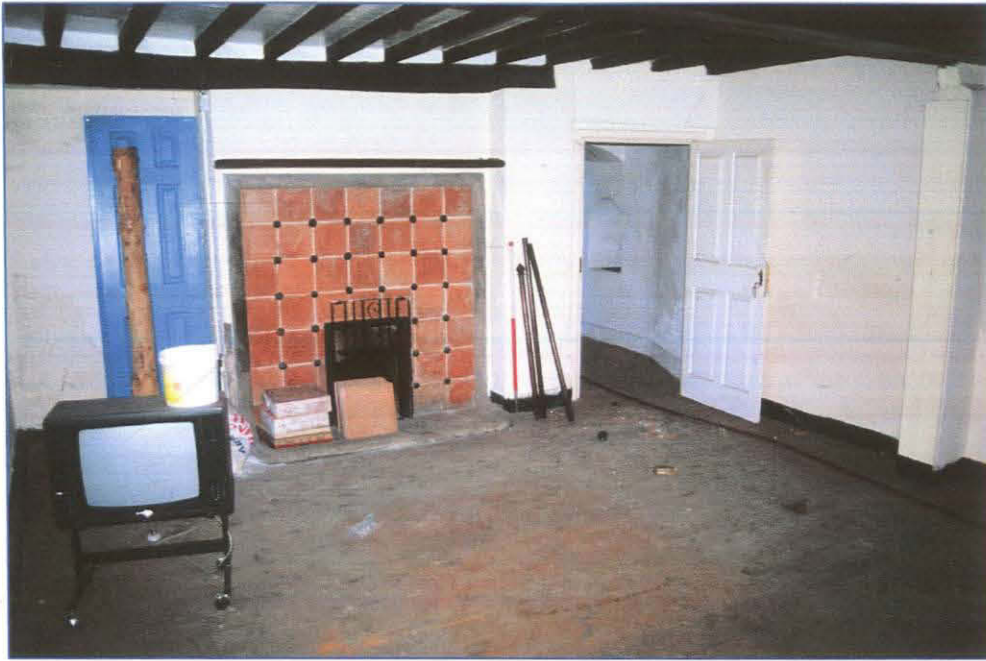
Plate 25: (041) Room 3 has a beamed ceiling with a large cross beam supporting squared timber joists, with a further beam set into the chimney breast crossing a recess on its eastern side. There is a tile backed modern retro fireplace incorporating iron studs and a small grate fitted to the chimney breast on the south wall. The floorboards are also a relatively recent addition to the building and the internal doors are modern replacements. Looking south-east.
