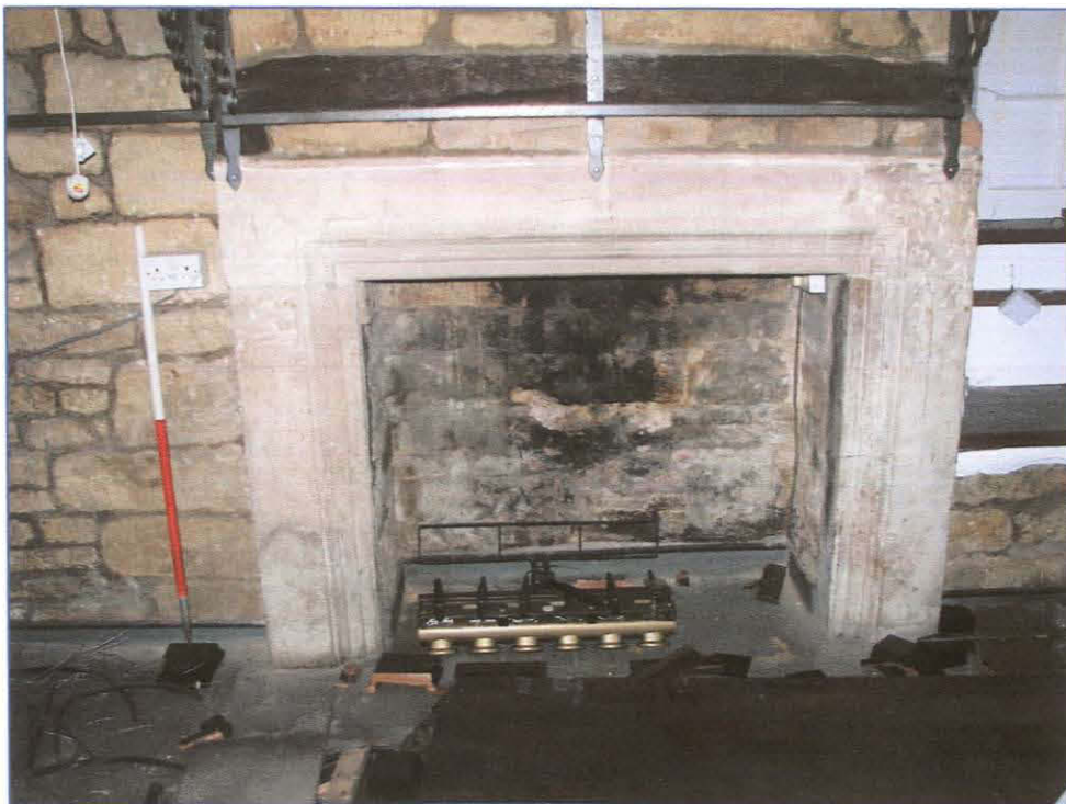
Plate 18: (056) Room 6 in the Western Range, 17 th century open fireplace with a stone surround. Looking west.
