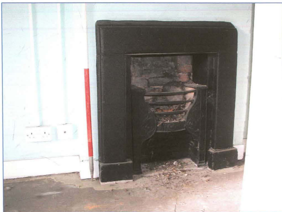
Plate 10: (123) Room 18 retains a late 18 th early 19 th century cast iron hob grate with a plain stone surround. The same style of fireplace has been retained in rooms 19, 20 and 21. Looking north-north-west.
