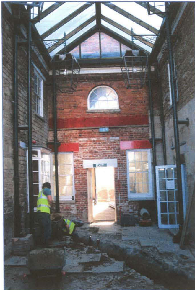
Plate 8: (027) Northern elevation of the carriageway arch with 19 th century infilling on the ground floor. Note the offset of the ashlar blockwork facia, in the right hand corner, necessary to correct the alignment between the Southern and Western Ranges. Looking south.
