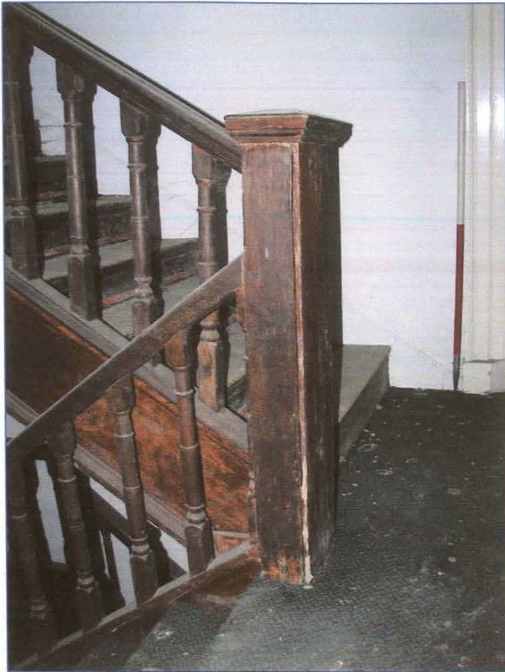
Plate 17: (167) The Western Range staircase, later 17 th /early 18 th century style, closed string construction with simple turned balusters, heavy plain handrail and balusters. Looking north.
