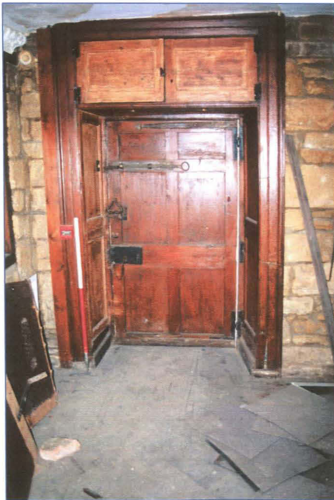
Plate 20: (055) Room 6, mid 18 th century style six panelled door with L shaped hinge and contemporary iron work. The door is set within panelled jambs below a built in cupboard. Looking east.
