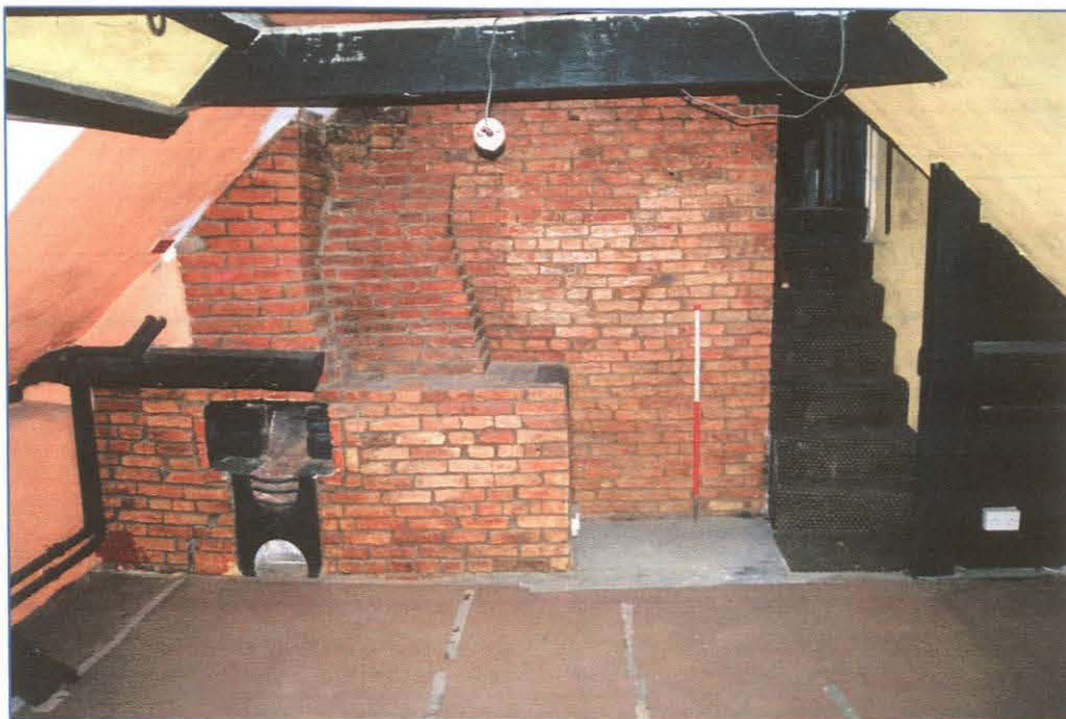
Plate 23: (083) Room 14. The southern wall is dominated by a large brick chimney breast that has a small hob grate built onto its eastern side. This structure also supports the stub end of a cross beam that has been cut to accommodate the insertion of stairs from Room 13. A timber stanchion at the foot of the stairs supports the opposing beam stub. Looking south.
