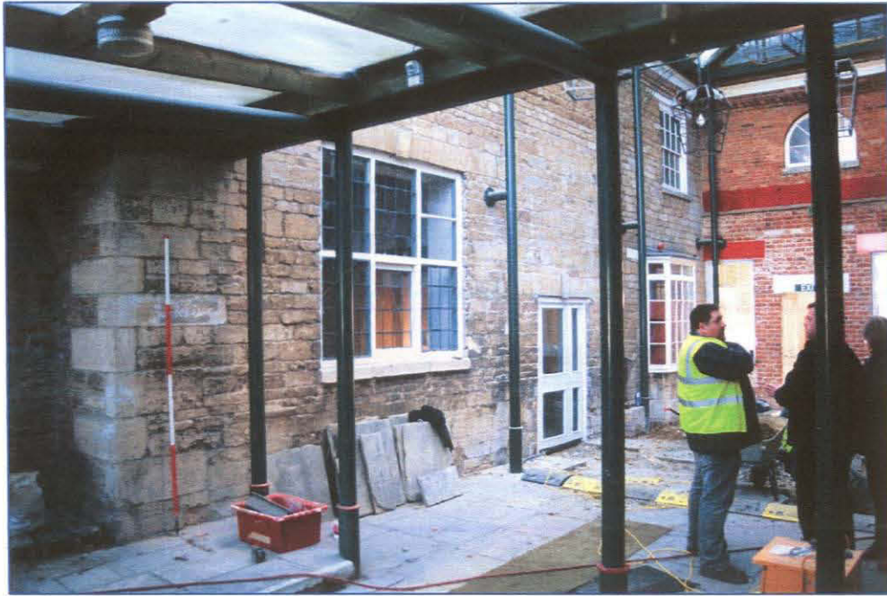
Plate 7: (021) Western (internal) elevation of the East Range (South Block). Looking east.
