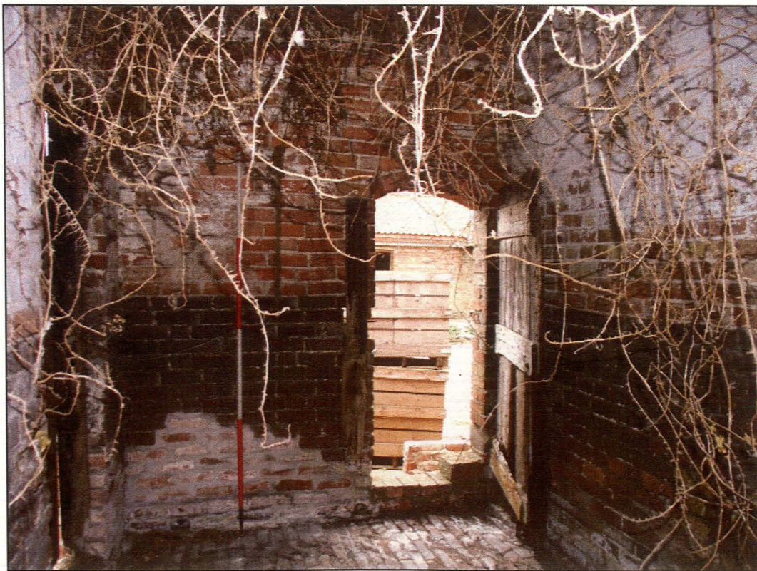
Plate 42 (Shot 79): Interior shot of store B9 showing two accesses and the original brick floor. Looking west-north-west
