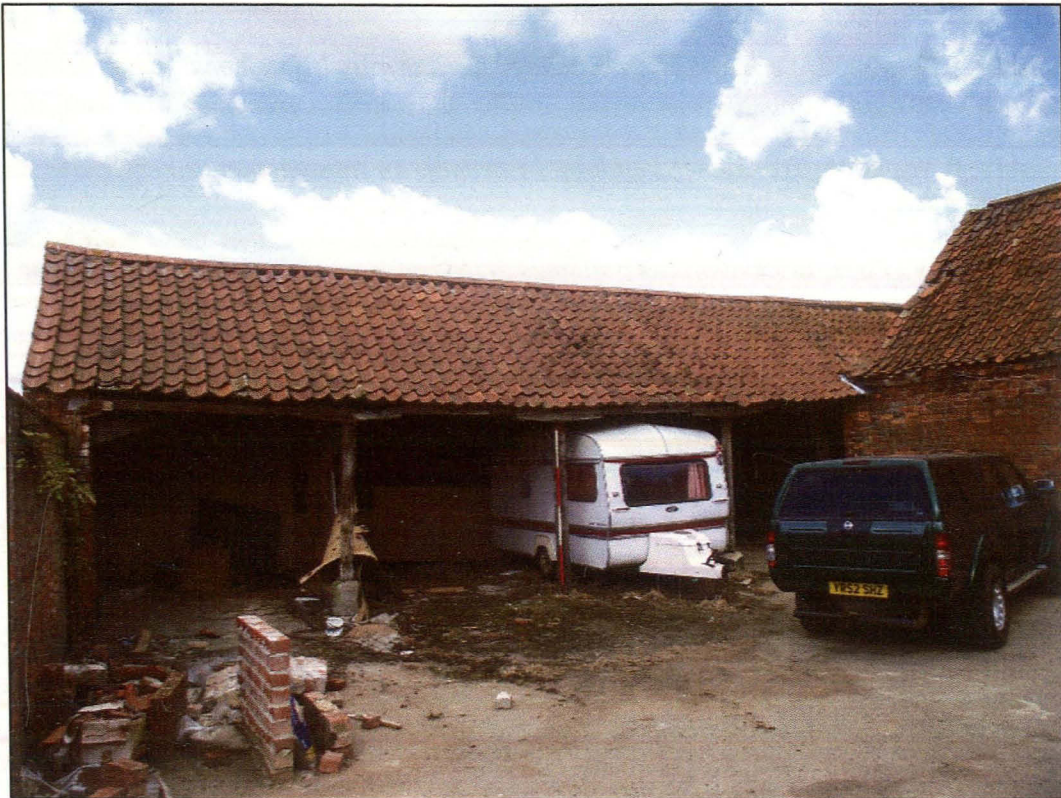
Plate 1 (Shot 11): East-north-east facing elevation of animal shelter A1, looking north-west
