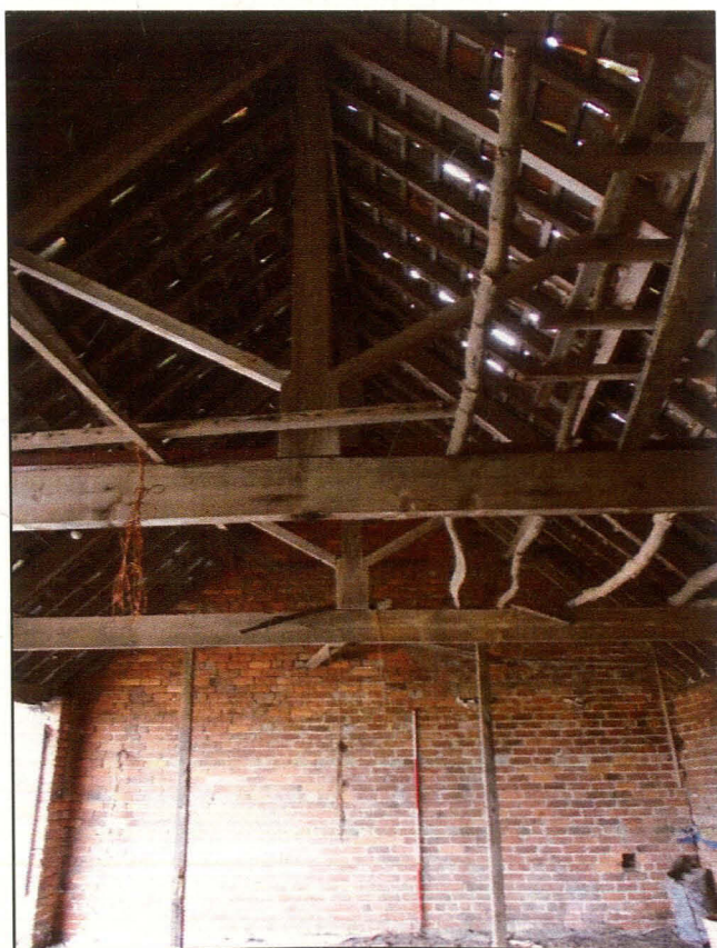
Plate 12 (Shot 32): Kingpost roof structure in cart shed A1, looking east-north-east
