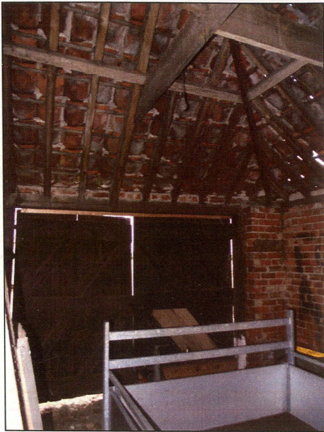
Plate 9 (Shot 18): Store A3 interior, looking north-west
