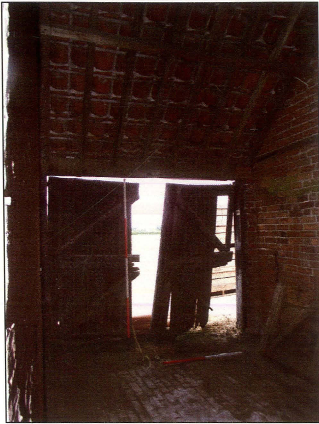
Plate 7 (Shot 15): General shot of store A2 interior. Looking north-west
