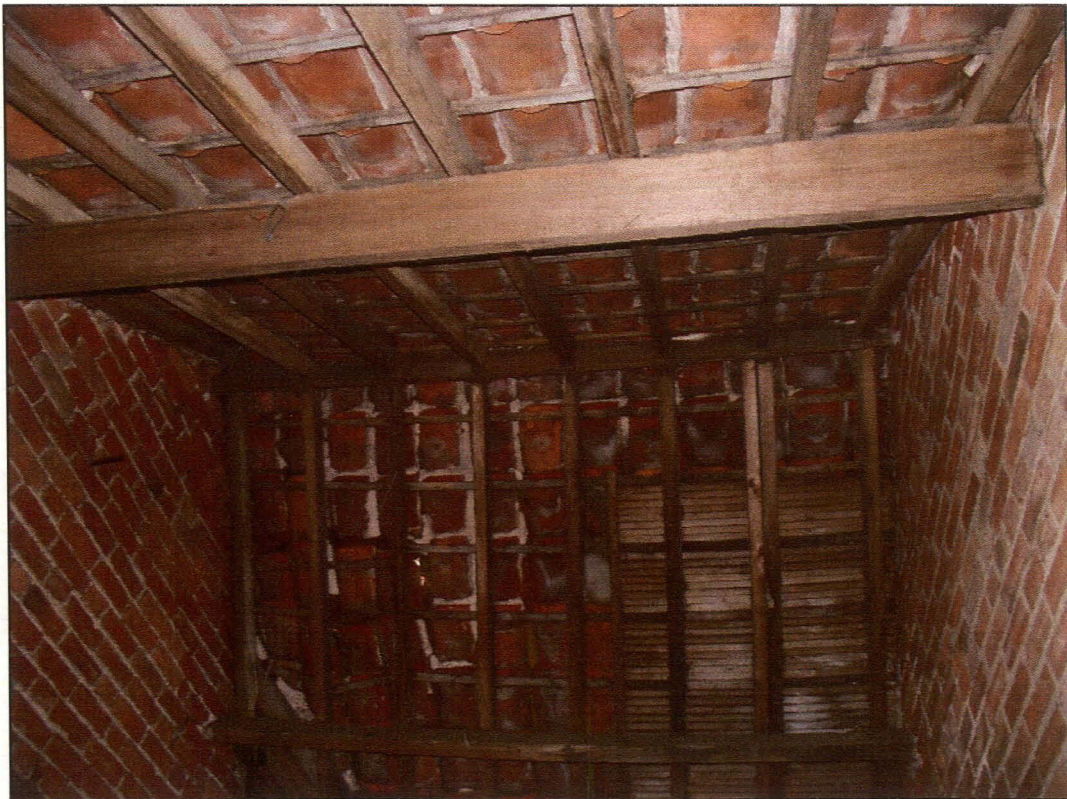
Plate 8 (Shot 17): Roof structure of store A2, looking north-east
