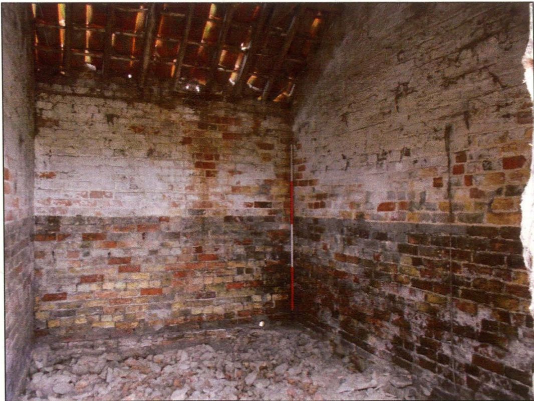
Plate 44 (Shot 84): General interior shot of store B11. Looking north-west
