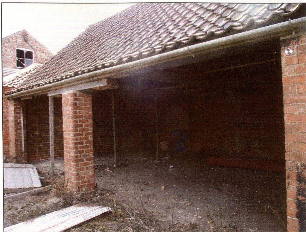
Plate 11 (Shot 36): Cart shed A1 showing central column of bullnose bricks and dirt floor, looking east-south-east
