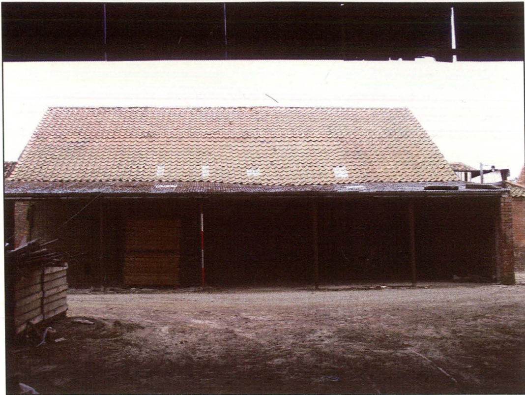
Plate 27 (Shot 26): North-north-east elevation of Block B. Looking south-south-east
