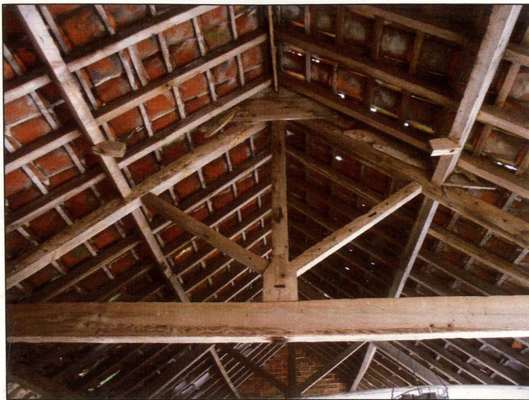
Plate 5 (Shot 13): Roof structure of animal shelter A1, looking north-north-west
