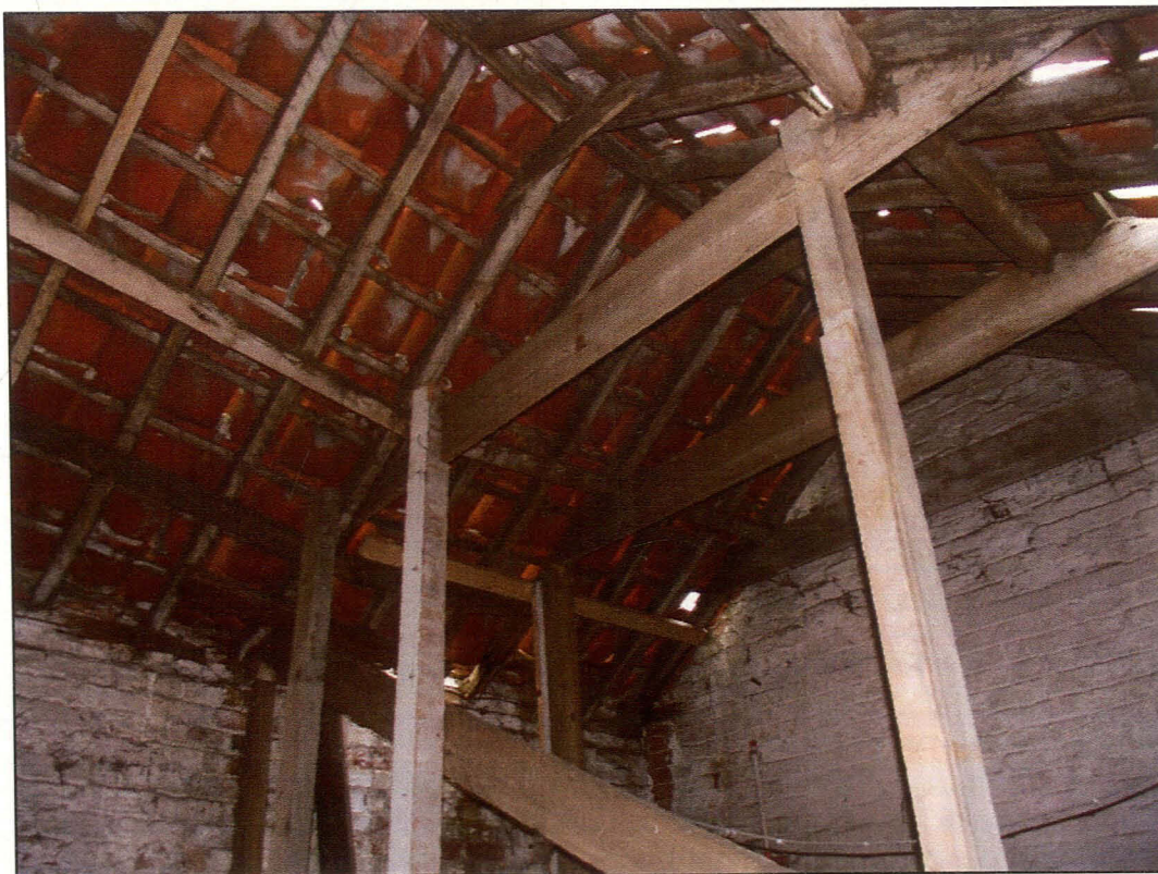
Plate 40 (Shot 76): Roof structure of barn B8. Looking south-east
