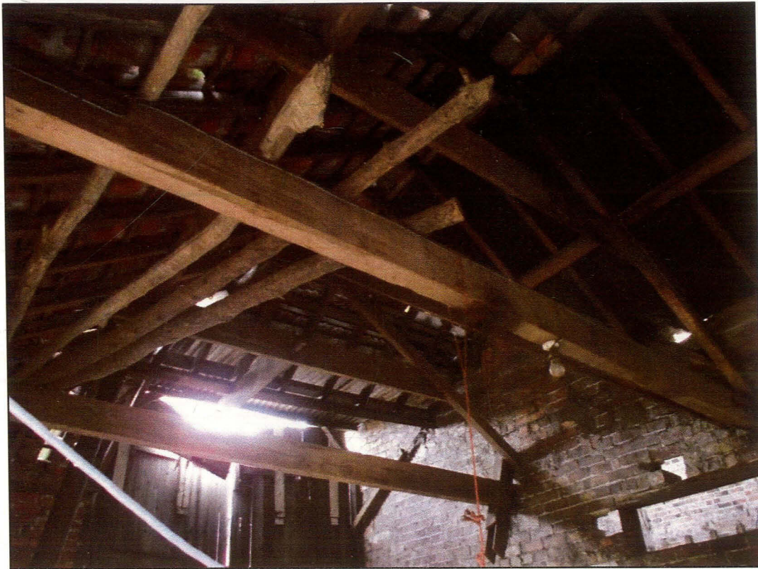
Plate 23 (Shot 52): Roof structure of barn B4, looking north
