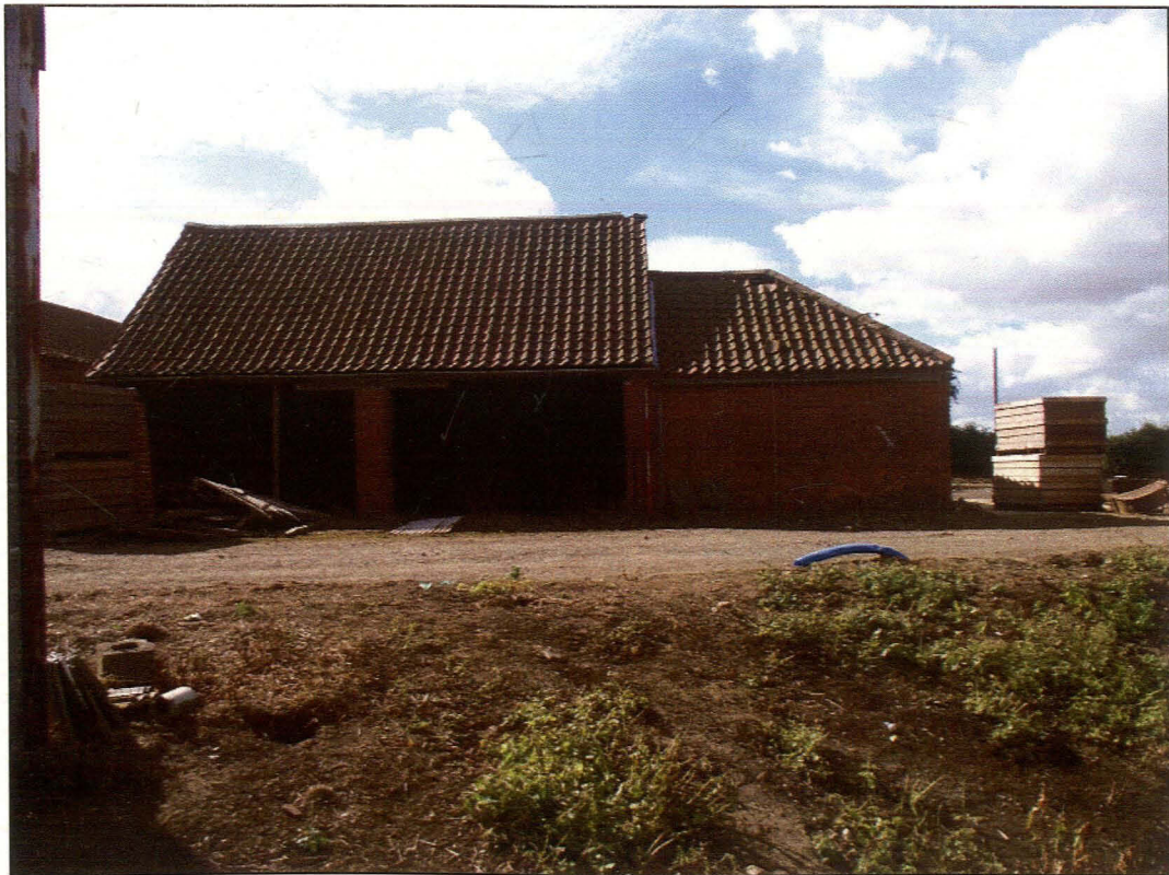
Plate 4 (Shot 10): North-north-west facing elevation of Block A, looking south-south-east
