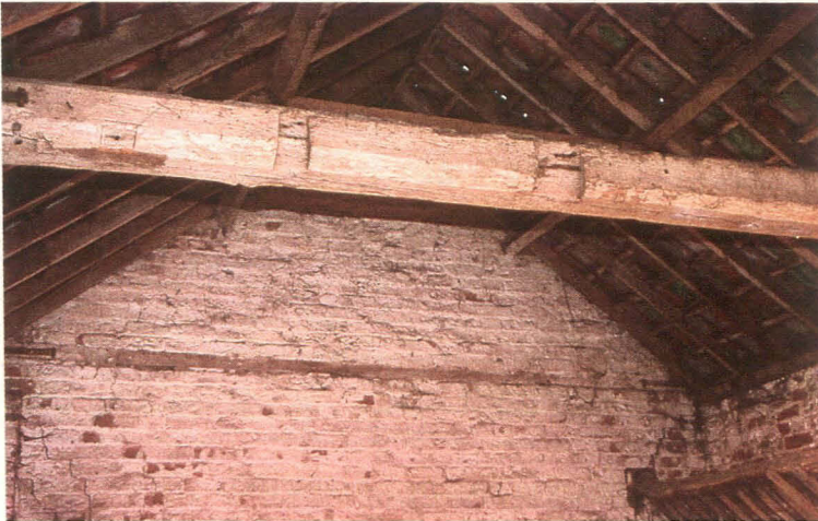
Plate 15 Centrally located reused overhead beam in cattle stall
