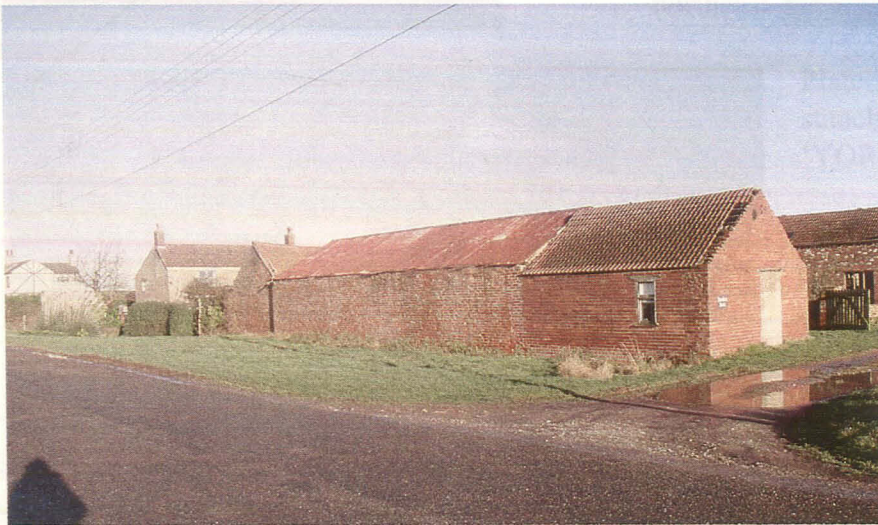
Plate 7 Western elevation of east-west block showing diaper pattern ventilation, looking east
