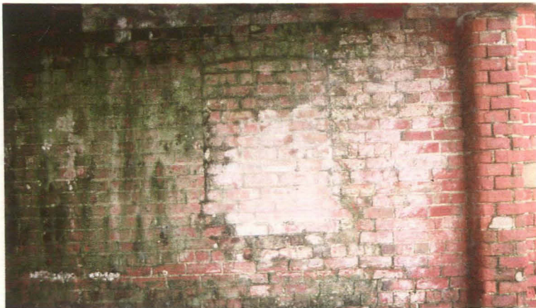
Plate 13 Blocked window in southern elevation, looking north
