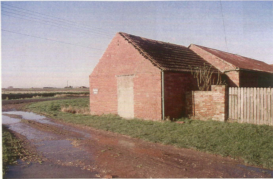
Plate 5 Southern elevation, showing blocked doorway, looking northwest
