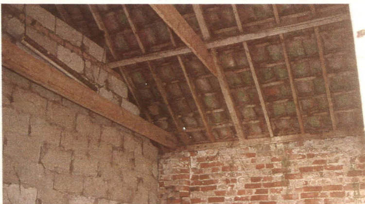
Plate 17 False internal wall divide, dividing space in east-west buildings, looking northeast
