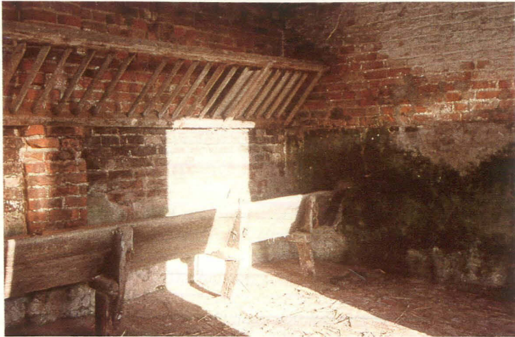
Plate 14 Cattle trough and overhead hay rack in cattle stall, looking northwest
