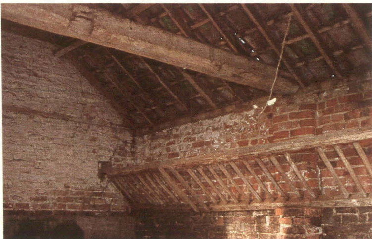
Plate 16 Hay rack and overhead beam, also showing roof detail
