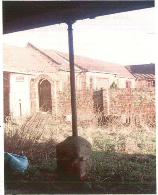
Plate 11 Detailed view of iron stanchion, embossed with 'YORKSTONE BOSTON'
