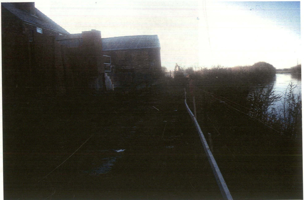
Plate 1 General Site View, looking south towards former mill
