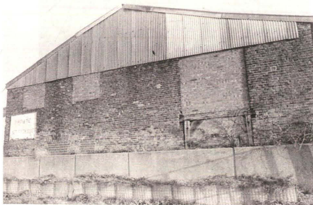
Plate 6 West Side of Former Mill, showing blocked entries, looking northeast
