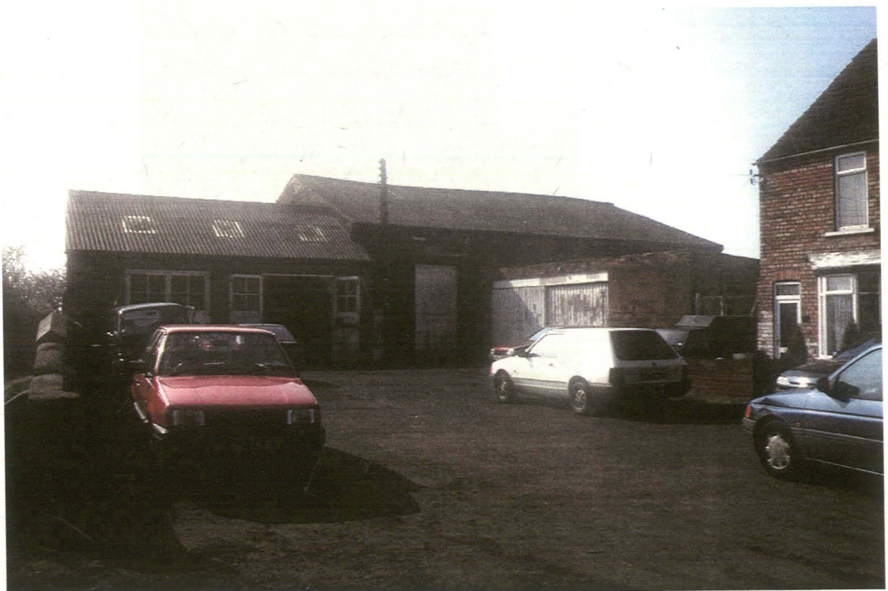
Plate 2 General View, north side of former mill, looking southwest
