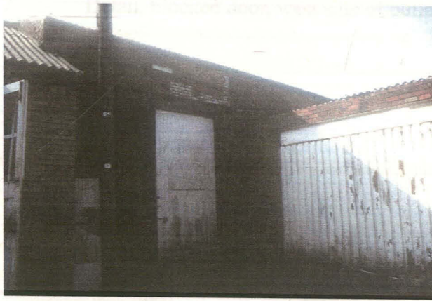
Plate 4 North Side of Former Mill, showing main entry and extension, looking southwest
