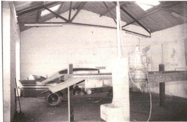
Plate 13 Interior of Eastern Extension, looking east
