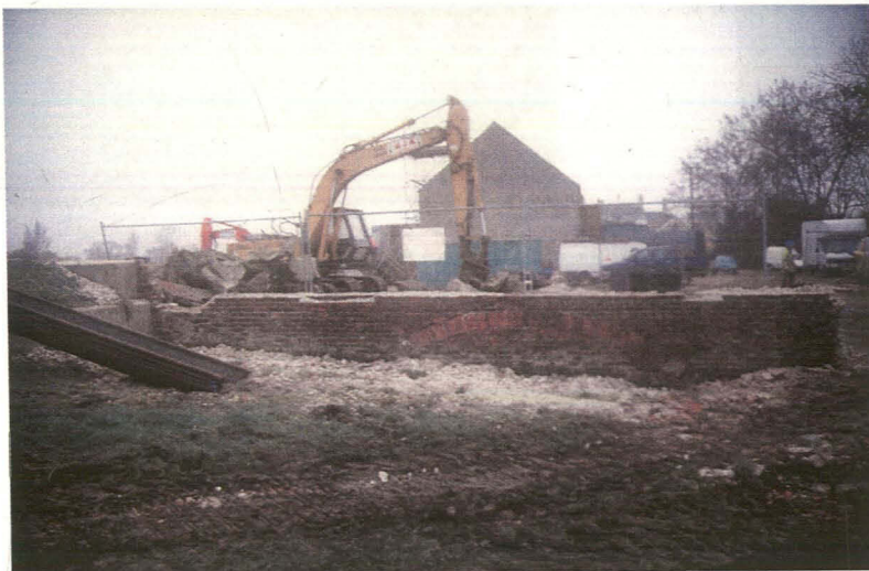
Plate 17 Partially demolished mill building, showing retained brick arch, looking northwest
