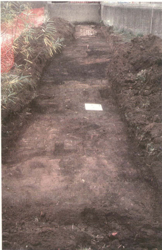
Plate 20 Stripped Area, northern end of site, looking north
