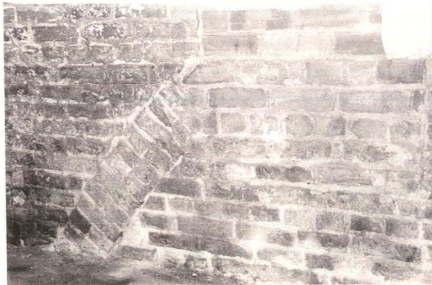
Plate 12 Detail, truncated brick arch, looking northwest
