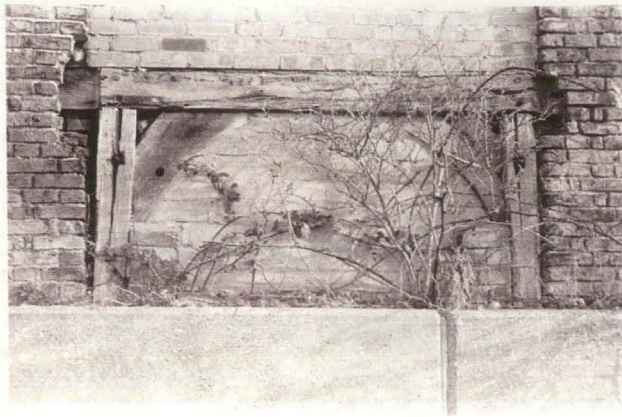
Plate 7 Detail, blocked door, west side of building, looking east
