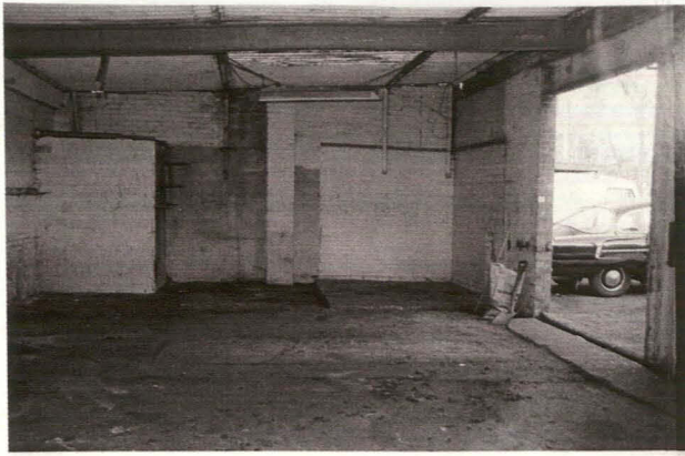
Plate 11 Interior Main Mill Building, east end, showing blocked entries, looking east
