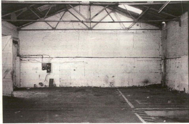
Plate 15 Interior of Northern Extension, looking north
