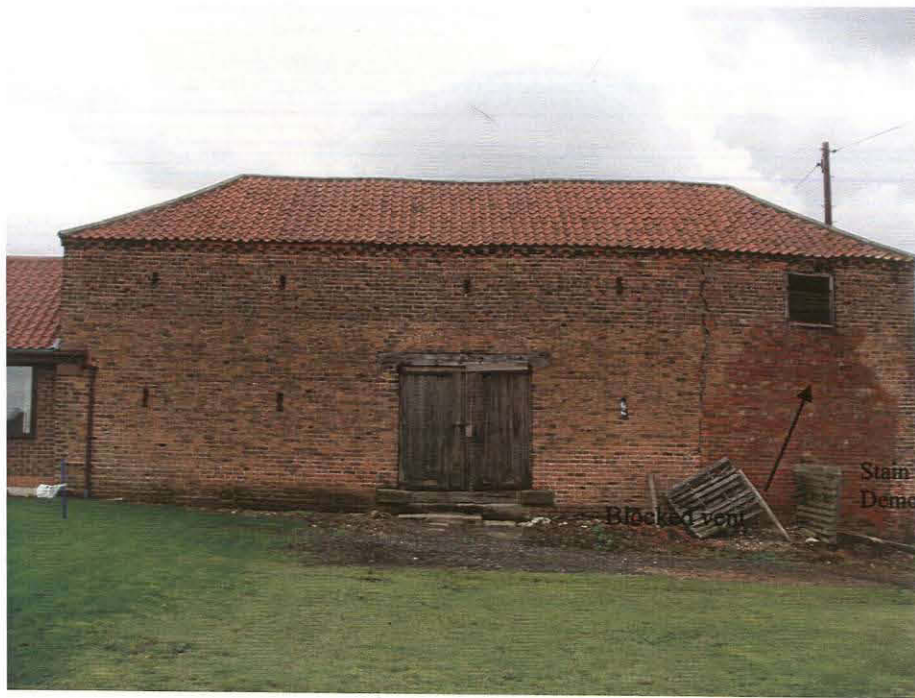
Pl. 13 Barn, east elevation showing two rows of vents, vertical crack, upper window at north end of building and stain marking position of demolished building
