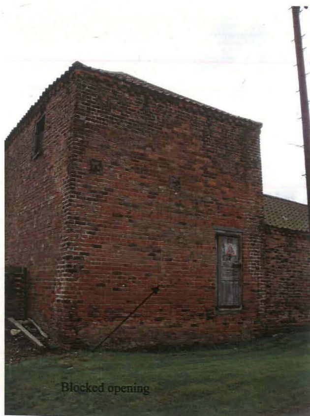
Pl. 13 Barn, east elevation showing two rows of vents, vertical crack, upper window at north end of building and stain marking position of demolished building
