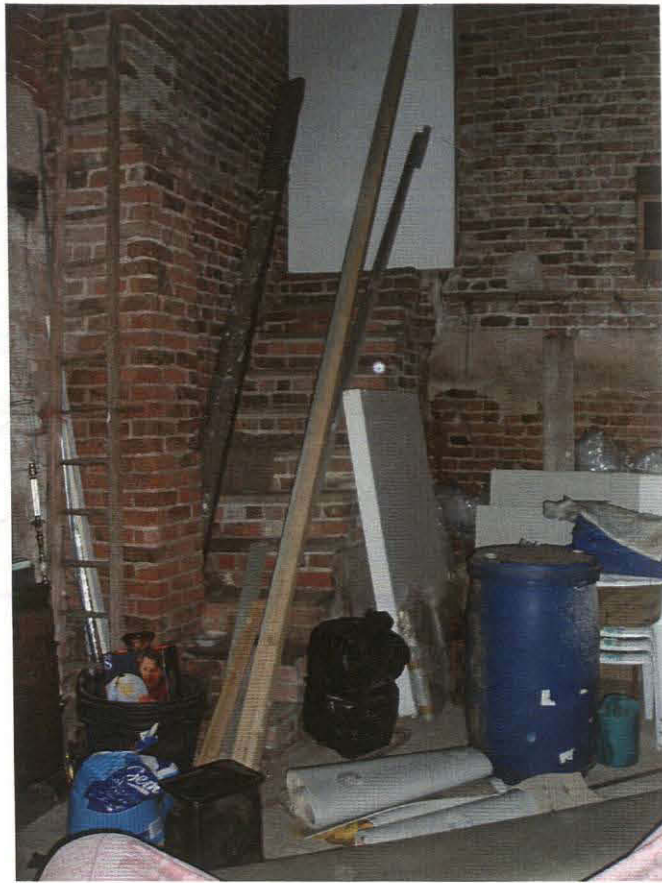
Pl. 19 Steps to north bay of the barn
