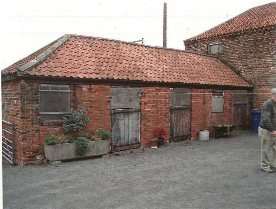
Pl. 26 The stable, south elevation, looking north
