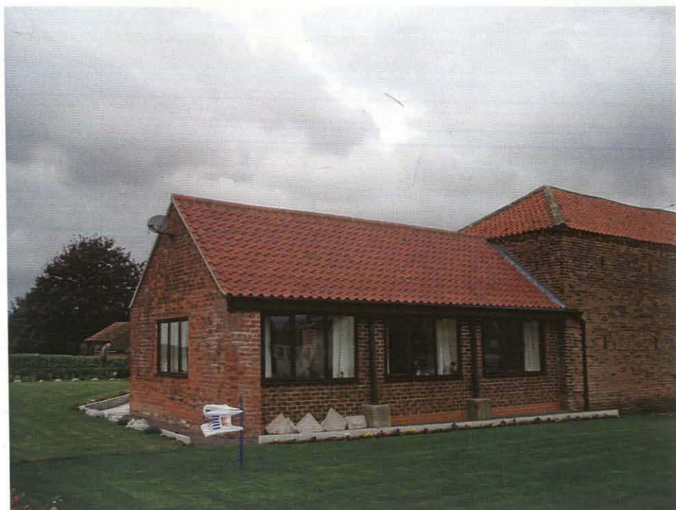
Pl. 21 The cart shed south of the barn, after conversion, looking west
