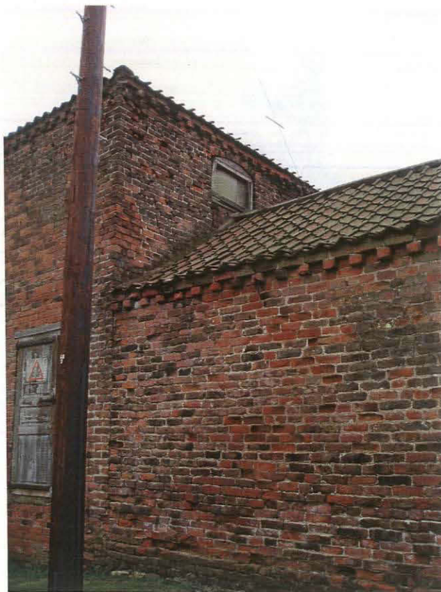
Pl. 3 Junction of the barn and the north boundary wall.
