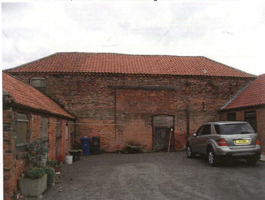
Pl. 15 Barn, north elevation showing detail of inserted door.
