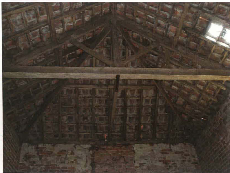
Pl. 20 Barn roof, south end, showing roof truss and hip.
