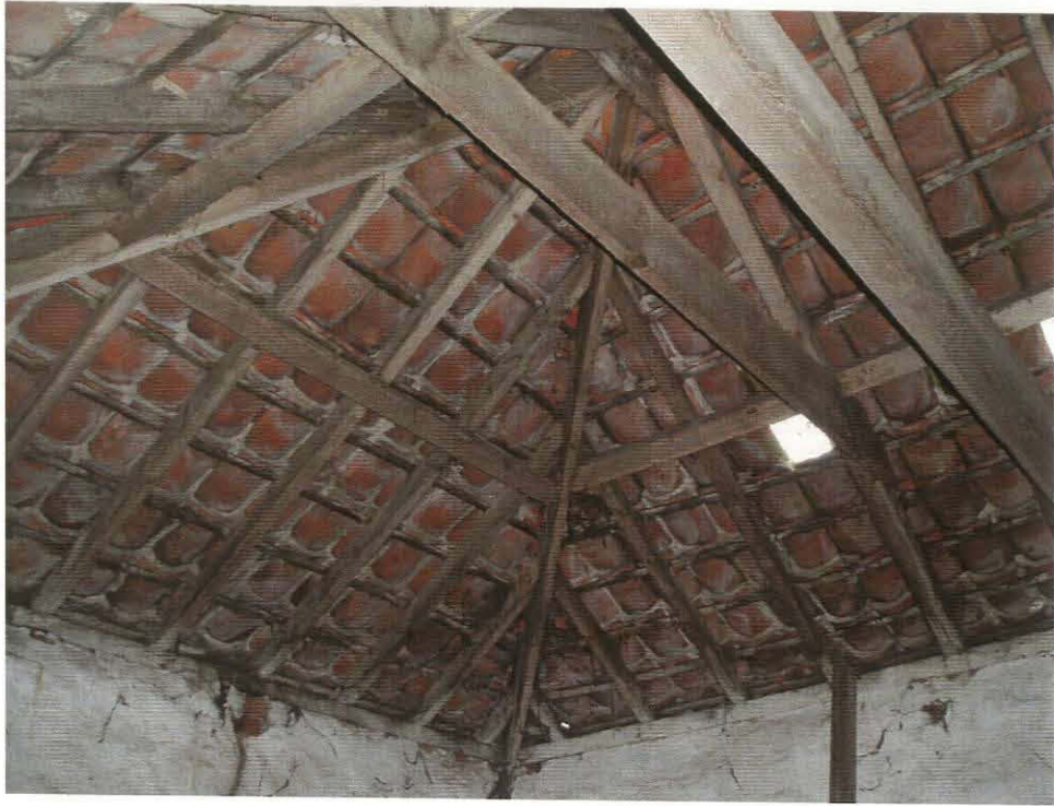
Pl. 29 The stable roof, hip at west end.
