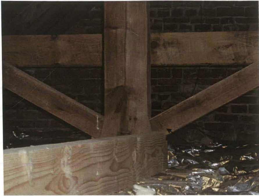
Pl. 25 The cart shed. Detail of Truss 1, showing truss number
