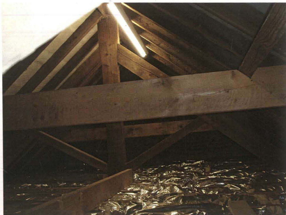
Pl. 24 The cart shed roof trusses, looking south
