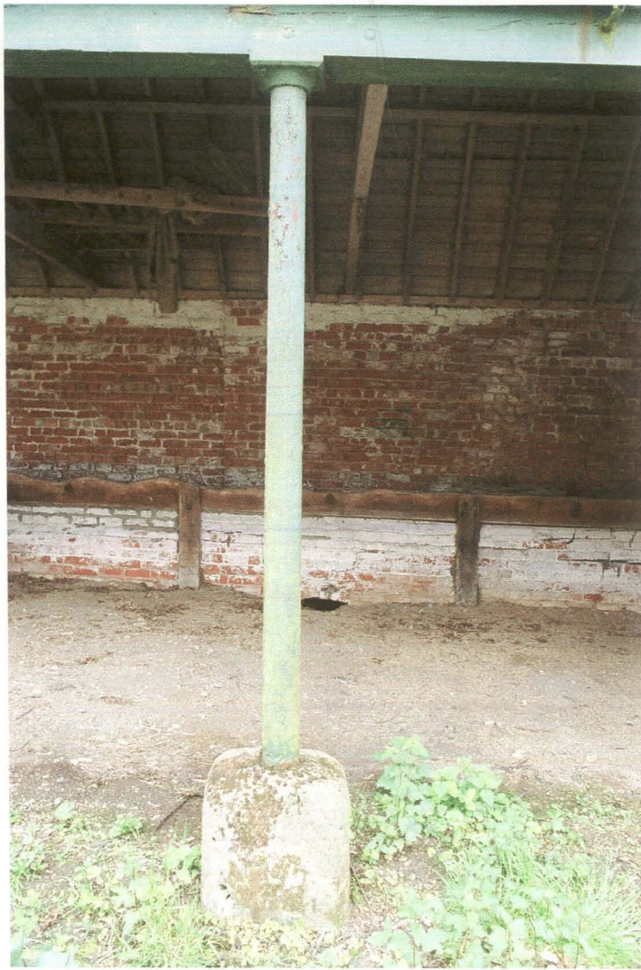
Pl. 33 Building 6, cast iron column with concrete base.
