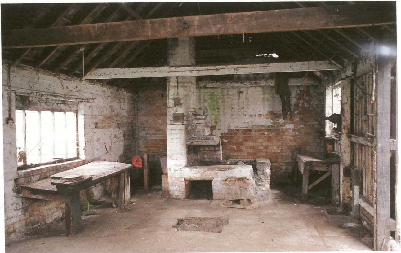
Pl. 13, Building 3, blacksmith's workshop interior looking north showing forge and work benches. Hole in flagged floor marks original position of anvil base which sits in front of forge.
