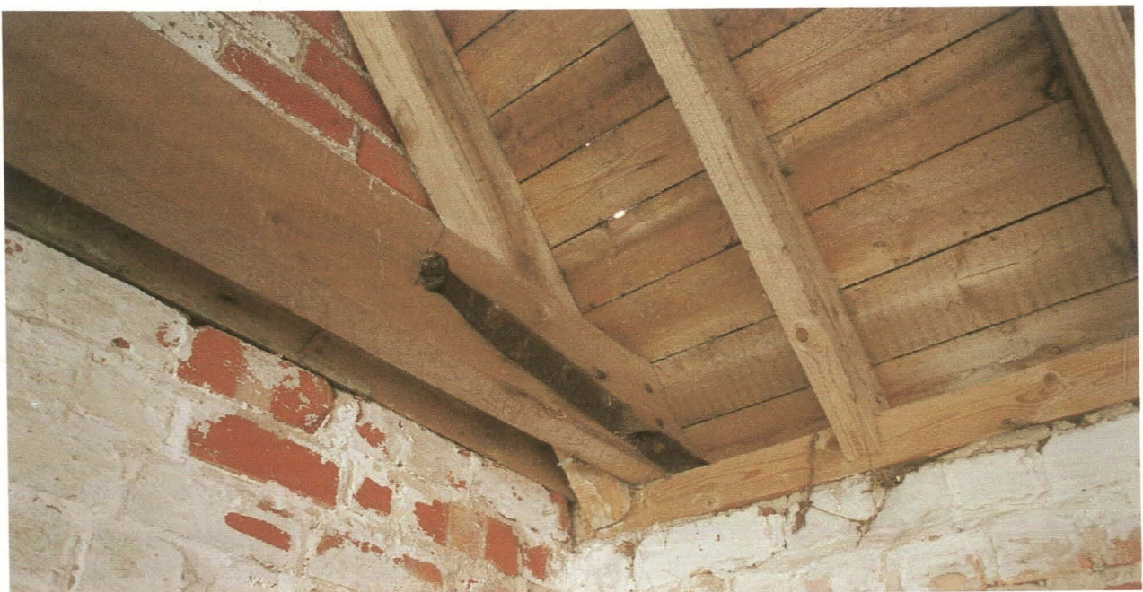
Pl. 37 Building 6. general view looking east showing roof construction, note internal boarding on south (right) side of roof only.
