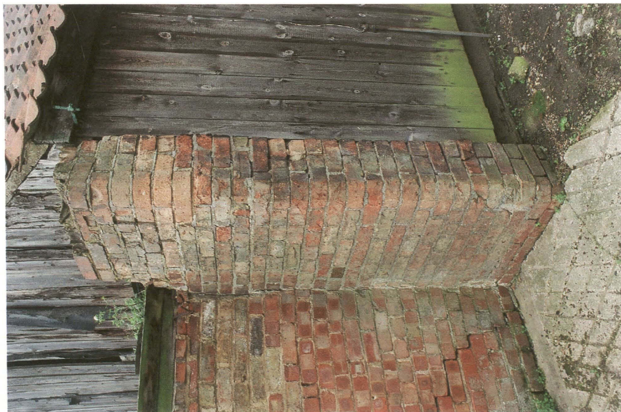
Pl. 25 Building 4. Chamfered pilaster at north east corner.
