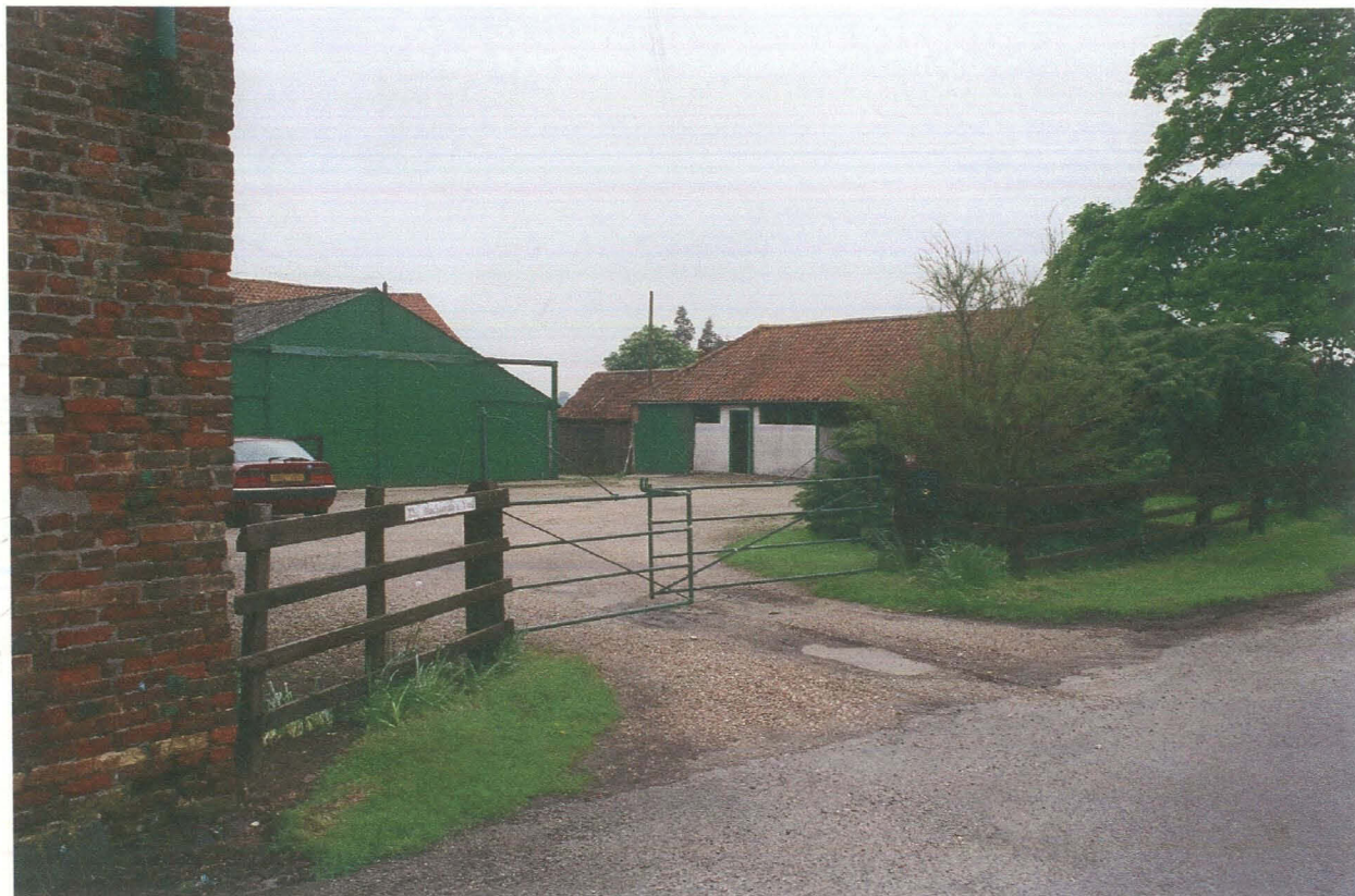
Pl. 3 General view of Blacksmith's Yard looking south-west.
