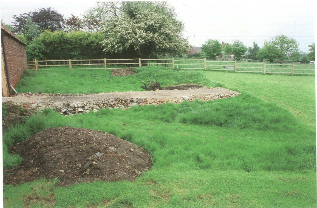
Pl. 36 Partially filled-in ditch behind Building 6, which runs east into adjacent property. View east.
