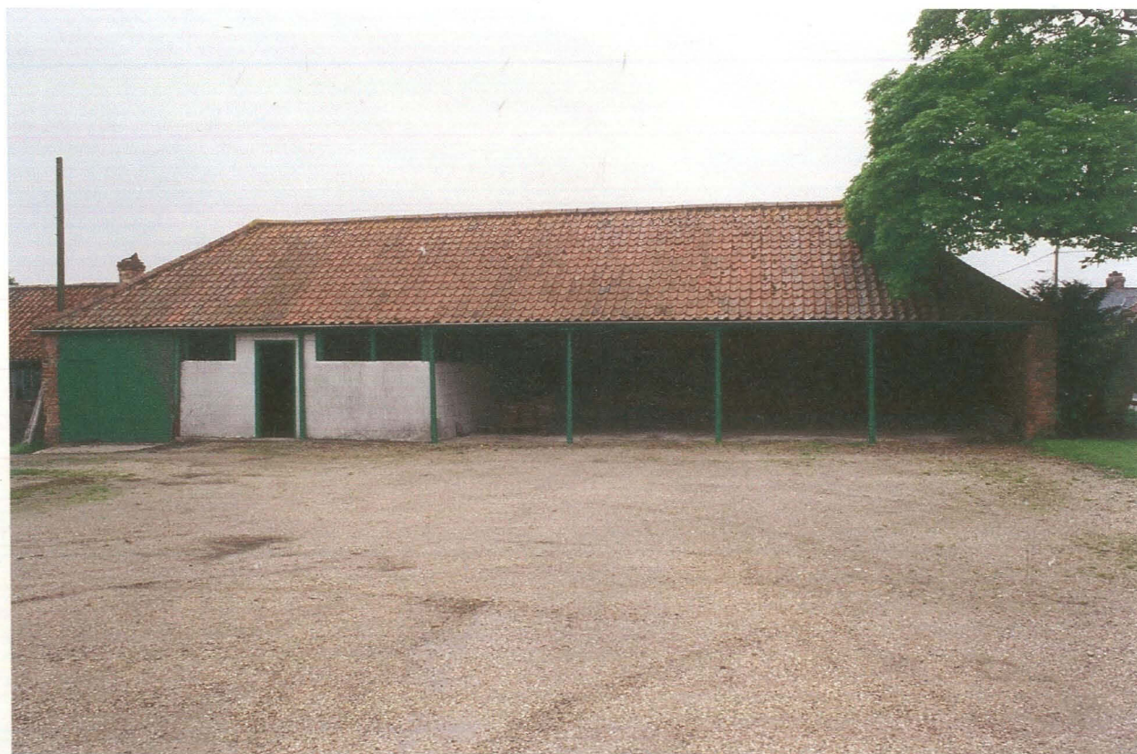
Pl. 4 Cart shed, Buildings 1 and 2 on west side of Blacksmith's Yard
