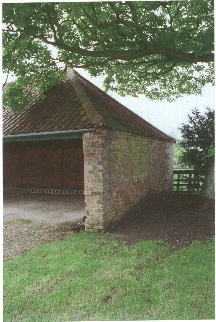
Pl. 6 North east corner of Building 1.
