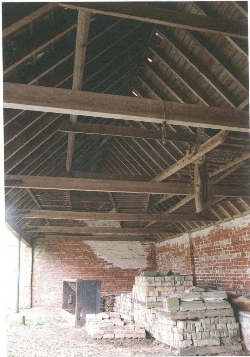
Pl. 37 Building 6. general view looking east showing roof construction, note internal boarding on south (right) side of roof only.
