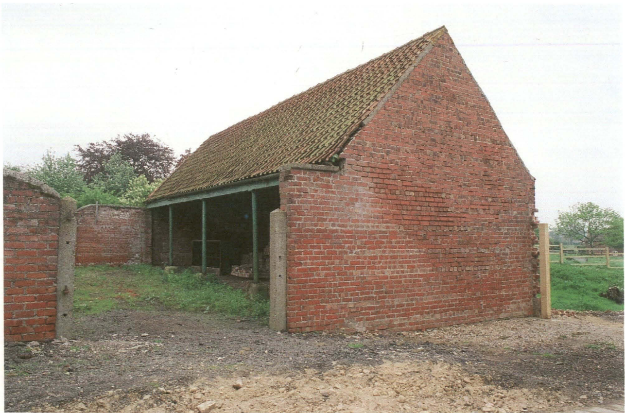
Pl. 30 Building 6, north and west elevations, looking south east.
