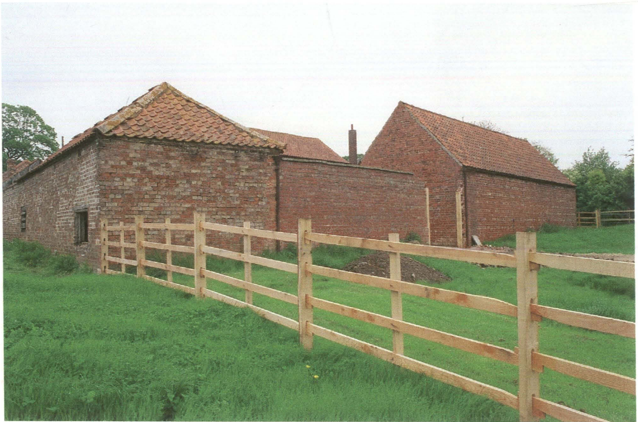
Pl. 29 General view looking north east with Building 5 to left, yard wall with inserted entrance attached to Building 6 to right.
