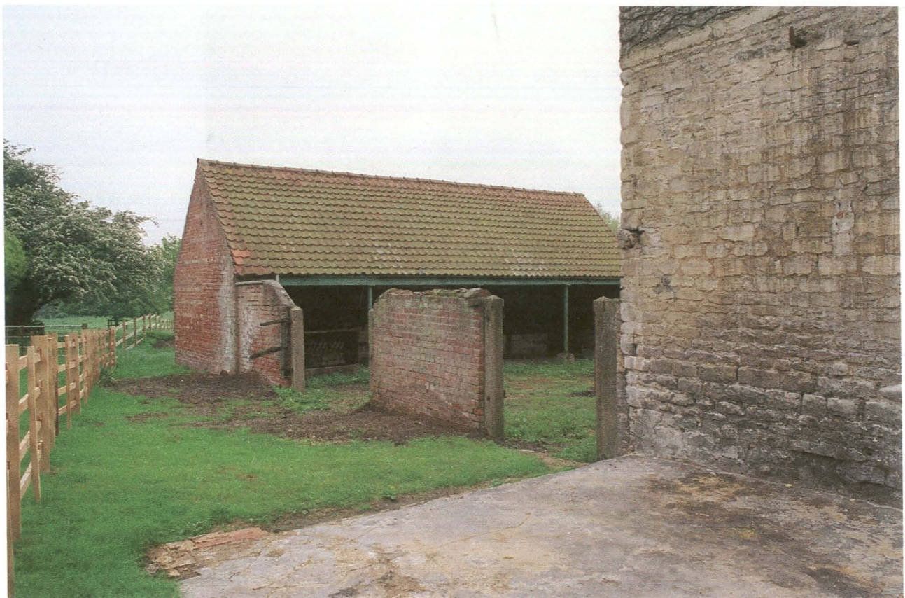
Pl. 31 Building 6, general view showing north and east elevations, with crewyard boundary wall and building 7 to right, looking south.
