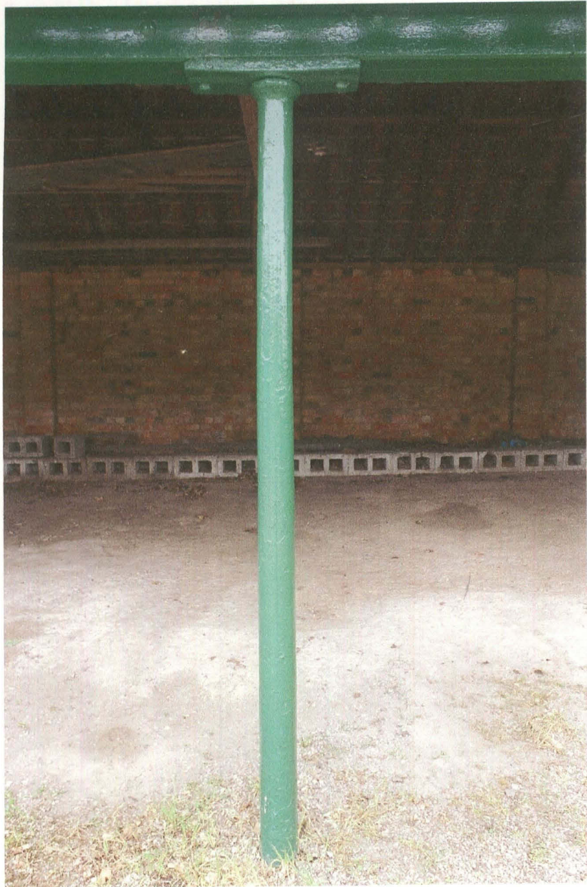
Pl. 5 Detail of cast iron column, Building 1.
