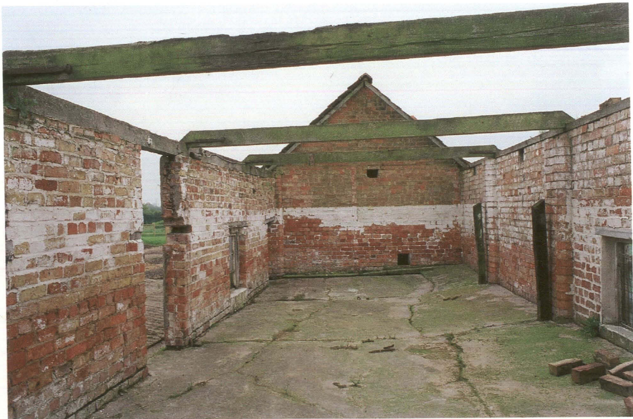
Pl. 22 Building 4 interior looking south.
