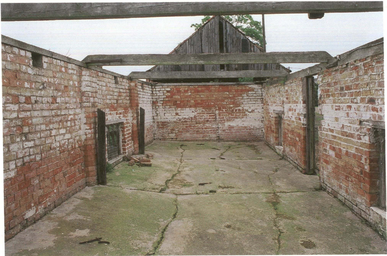
Pl. 21 Building 4 interior looking north, showing concrete floor and base of trusses strapped to eaves plate.
