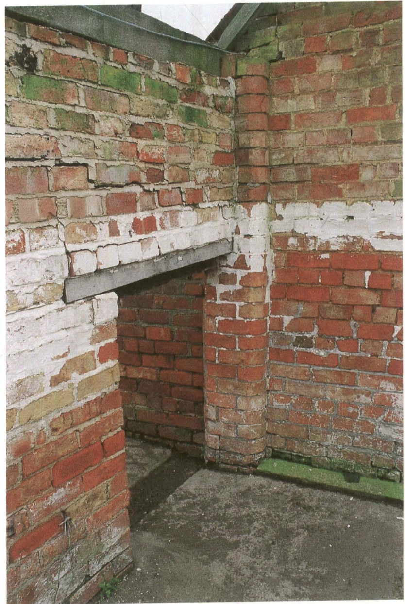
Pl. 24 Building 4. Chamfered pilaster at south east corner.
