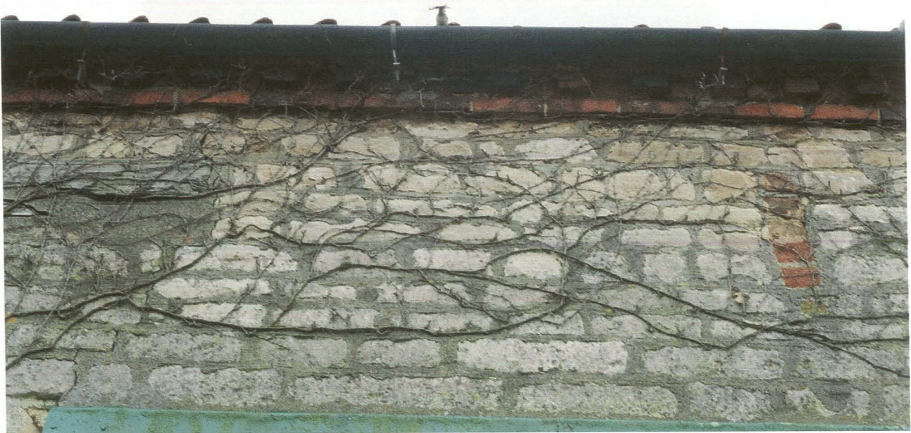
Pl. 43 Building 7, brick dentil detail at eaves height.
