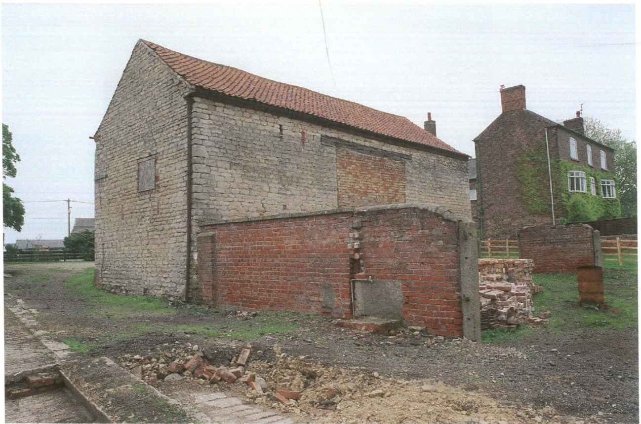
Pl. 39 Building 7, stone threshing barn, west and south elevations, looking north east.
