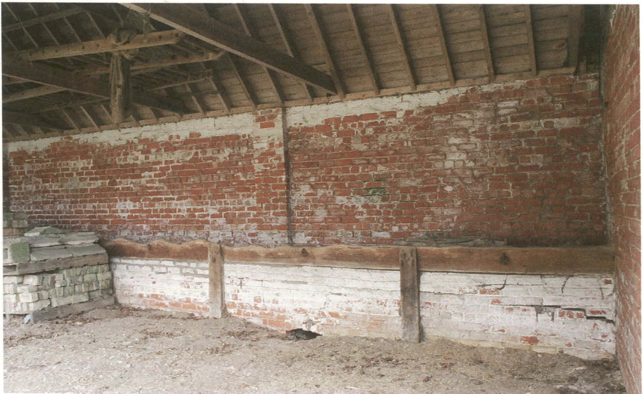
Pl. 34 Building 6. Feeding trough along south wall, with tethering rings attached to the board. Note brick pilaster marking the bay division.
