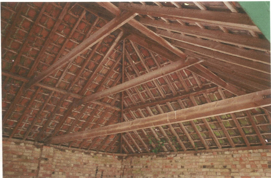
Pl. 8 Building 1, hipped gable and roof structure
