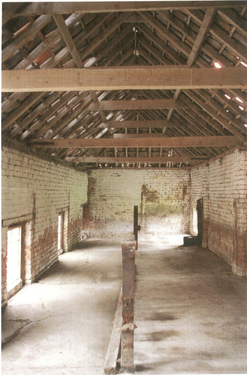
Pl. 27 Building 5 Interior looking south.
