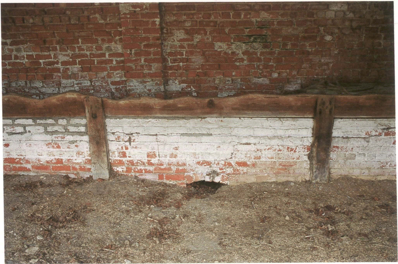
Pl. 35 Building 6. Detail of the drain beneath the feeding trough.
