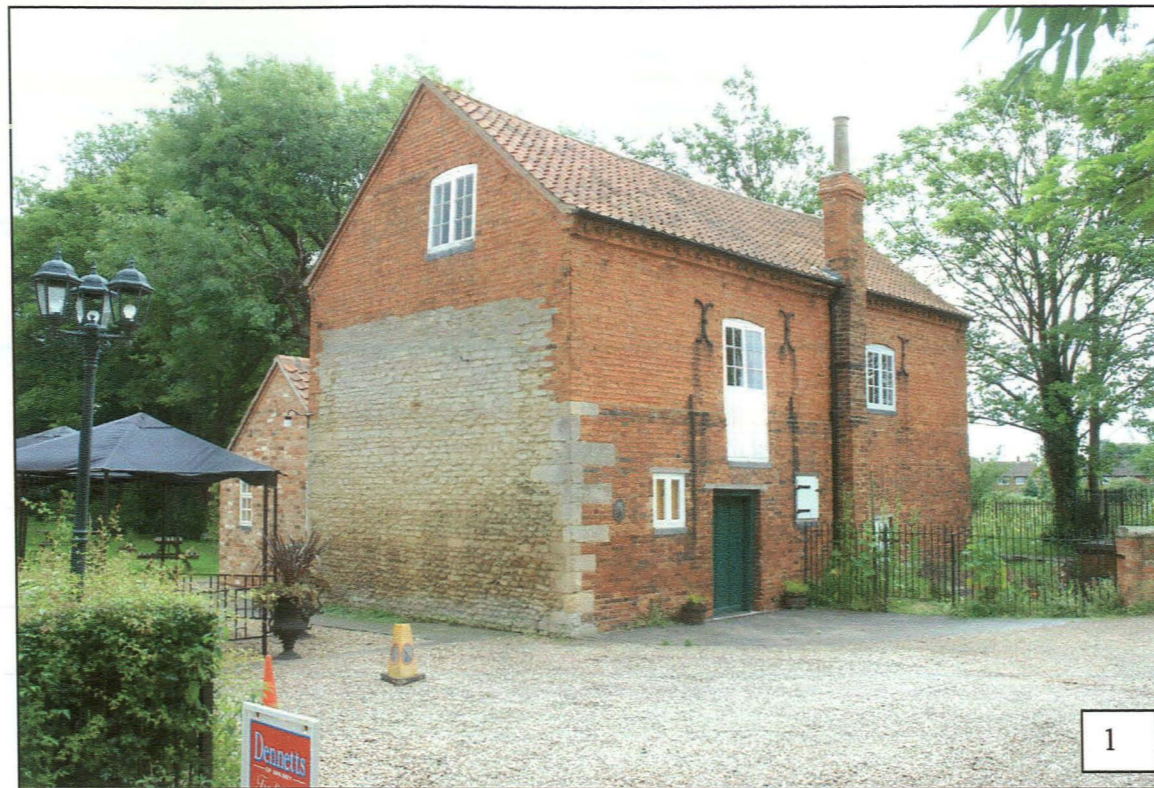
Plate 1: general view of the mill, looking southeast.
