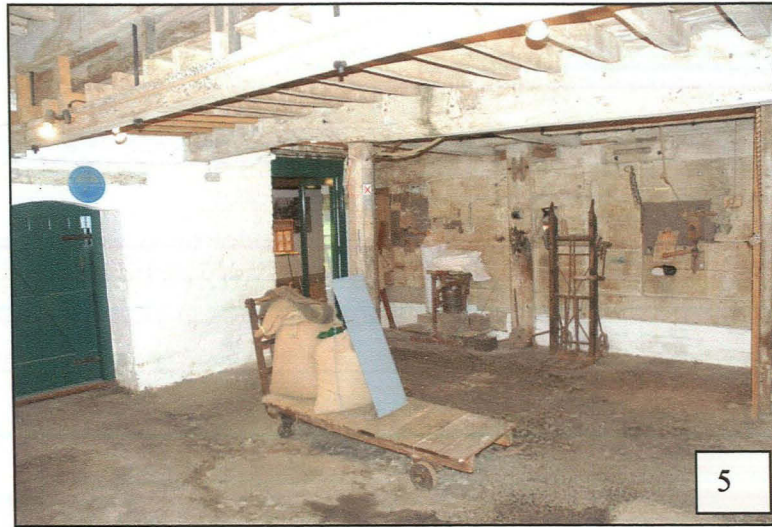
Plate 5: general view of Room 1, looking southeast. The timber partition from Room 3 with the flour chutes is visible on the facing wall.
