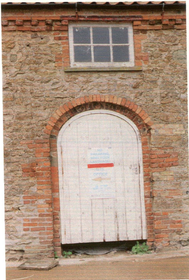
Plate 11: Barn (2), detail of exterior south elevation, showing original entrance and window above. Note the double pintle on the jamb, indicating that opening originally had a split stable door.
