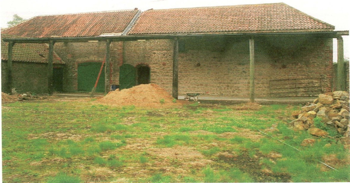
Plate 32: Exterior south elevation of Barn (3), with Dutch barn (7) adjoining.
