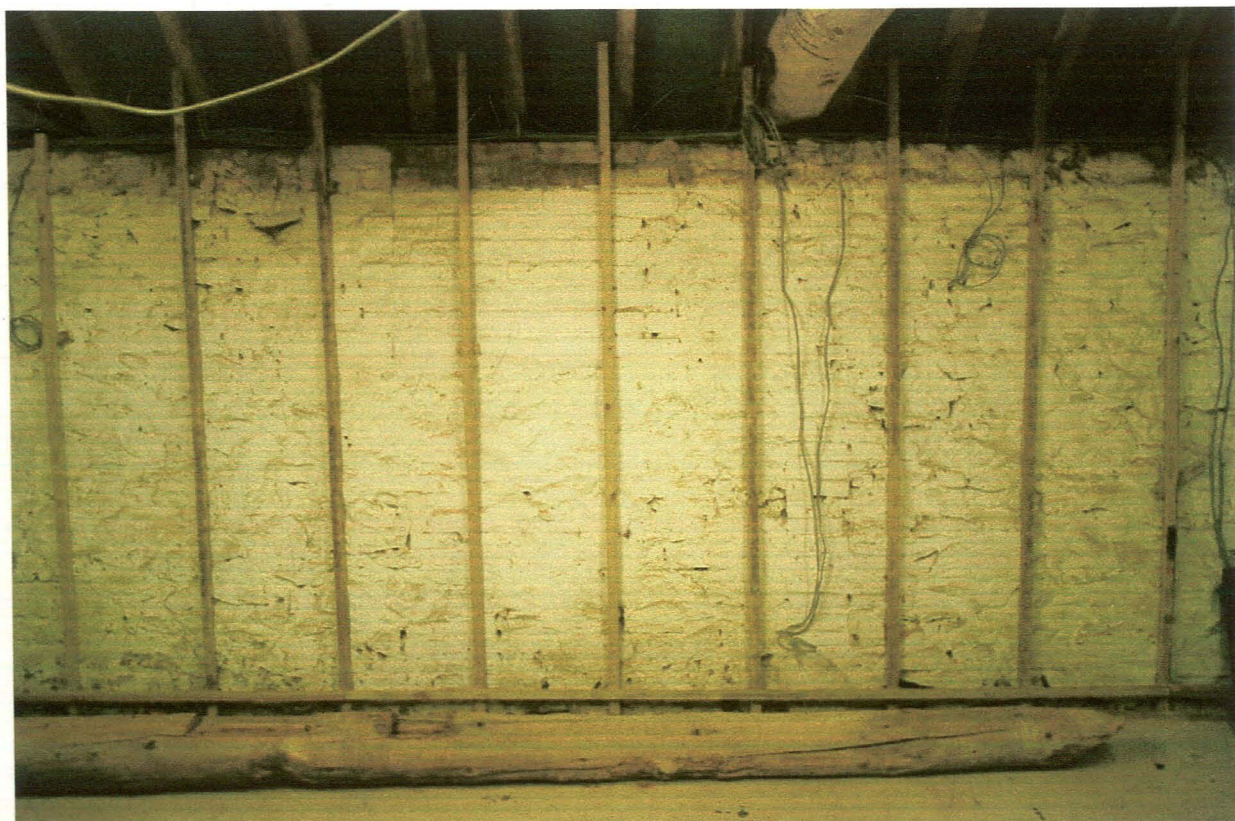
Plate 24: Internal west elevation of Stable block (4), showing blocked door.
