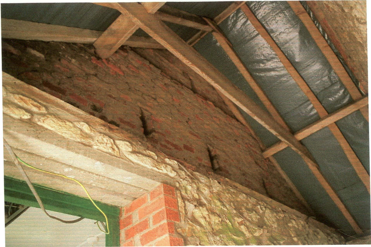
Plate 25: Stable block (4): detail of north gable wall, showing ventilation slits.
