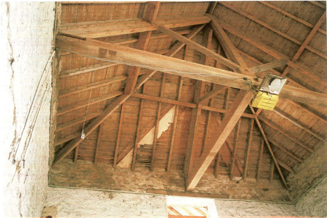
Plate 5: Interior of Barn (1), showing hipped roof at west end.
