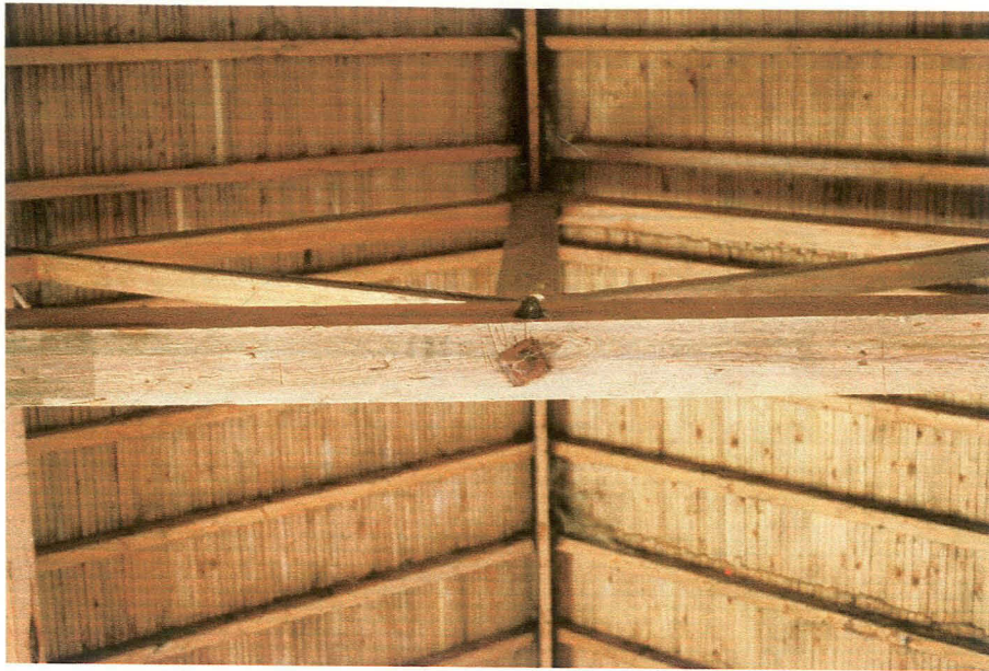
Plate 7: Barn (1) - detail showing batch mark on underside of crossbeam.
