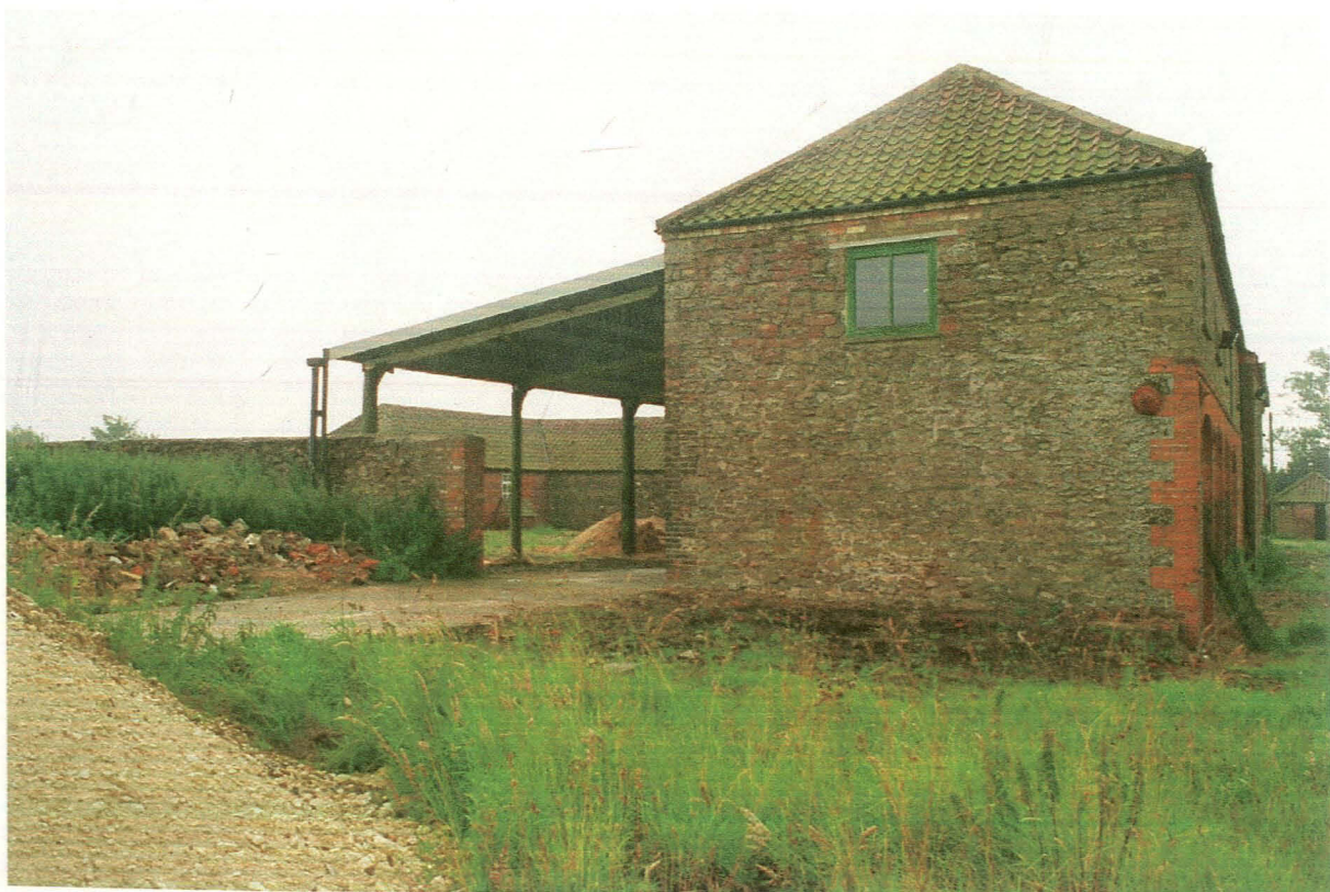
Plate 16: Exterior east elevation of Barn (3).
