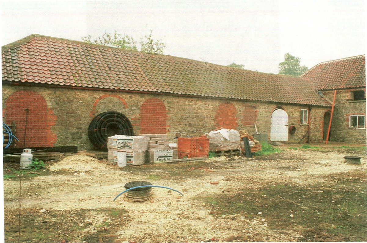
Plate 19: East elevation of Stable block (4).
