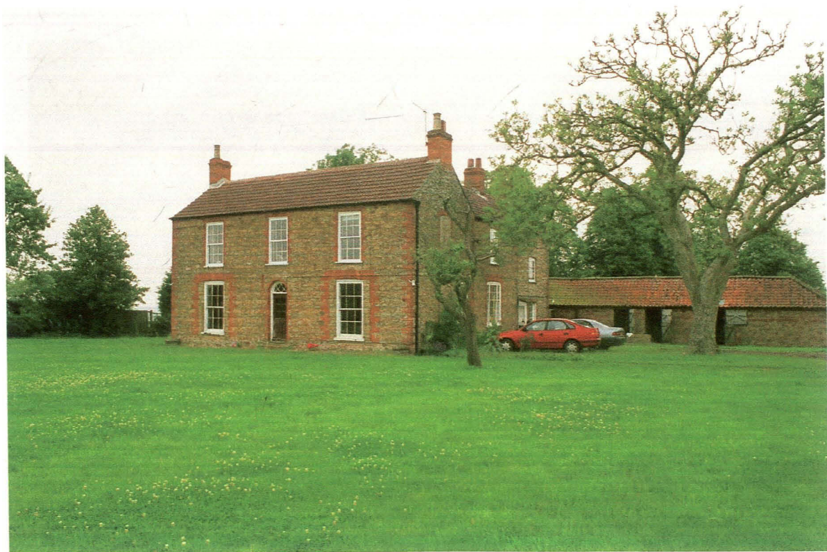
Plate 2: Exterior south elevation of Cow Pasture Farm, looking north.
