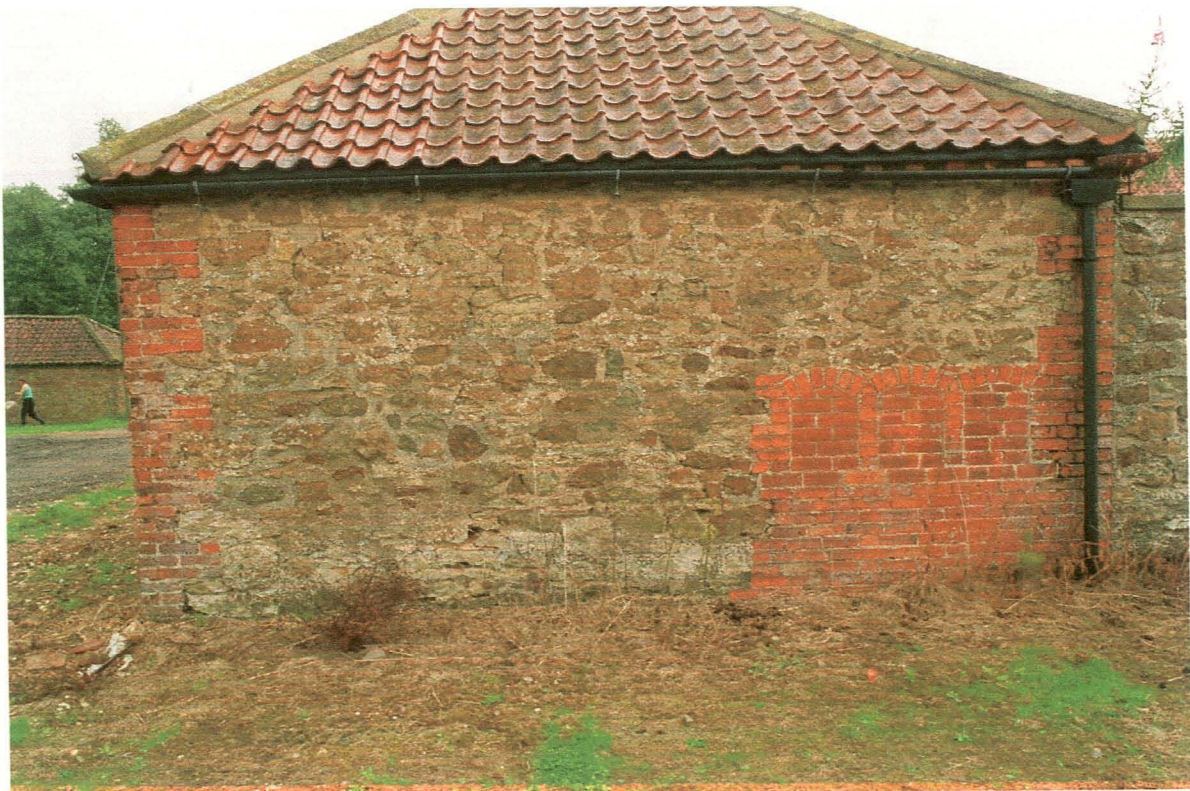
Plate 20: South elevation of Stable block (4). Note blocked niches.
