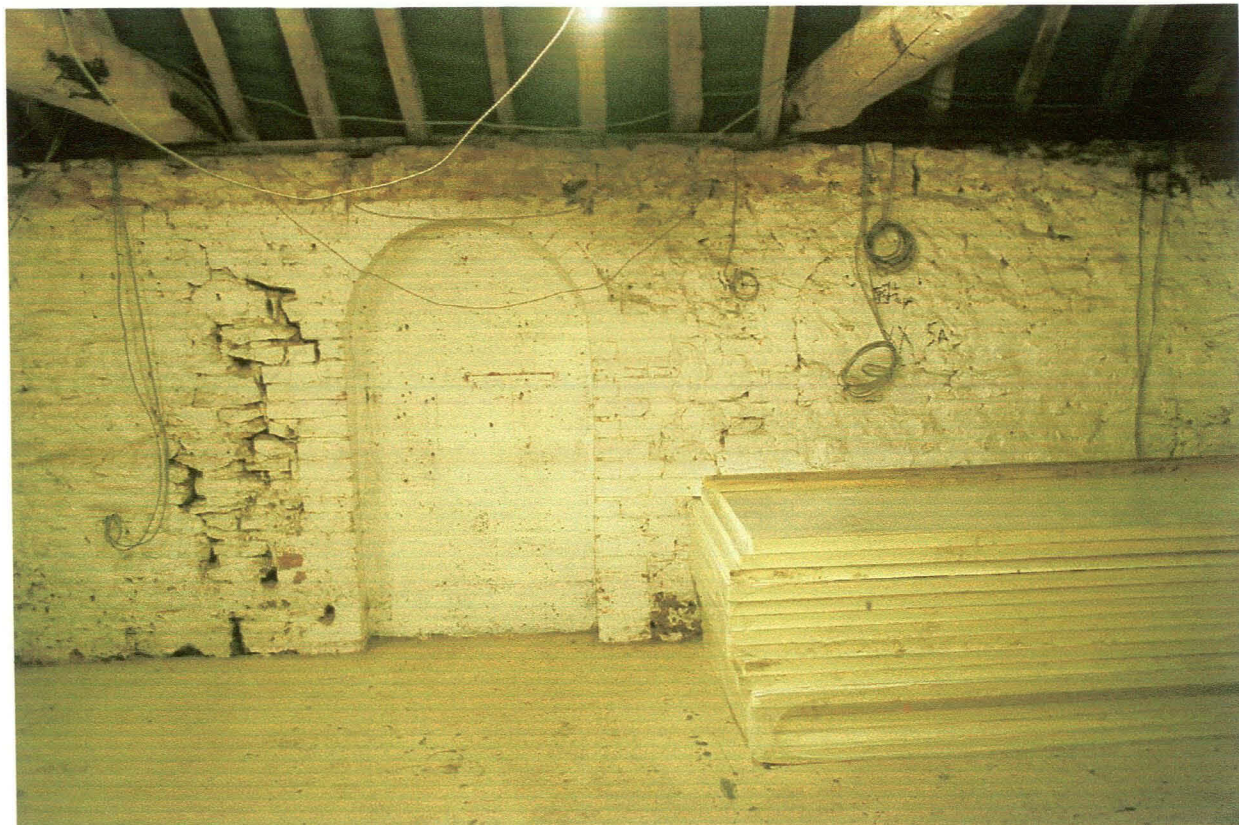
Plate 23: Internal east elevation of Stable block (4), showing blocked door.
