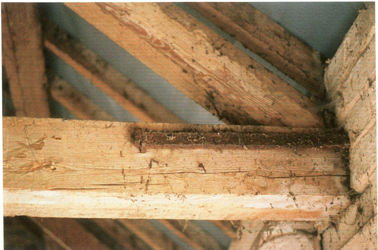
Plate 18: Barn (3): detail of iron strap used to secure tiebeam to wall.
