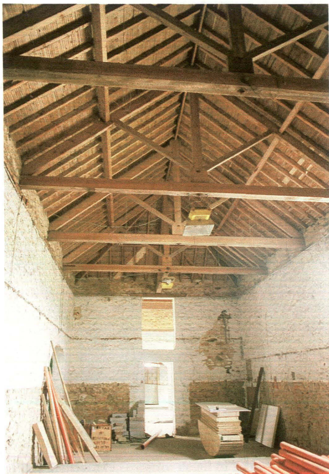
Plate 6: Interior of Barn (1) looking west.
