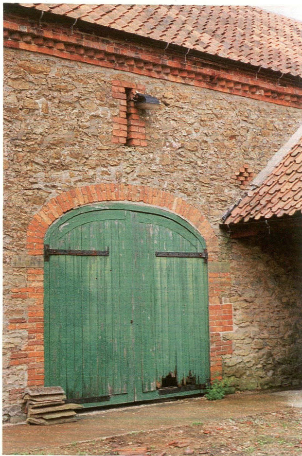
Plate 8: Barn (1) exterior detail of south elevation, showing entrance, ventilation slit above and diaper-shaped ventilation holes, partially obscured by later roof of Cattle shed (5).
