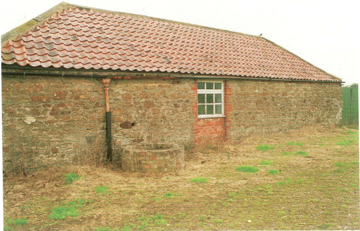
Plate 31: South elevation of southern boundary wall, incorporated into Store/office (6).
