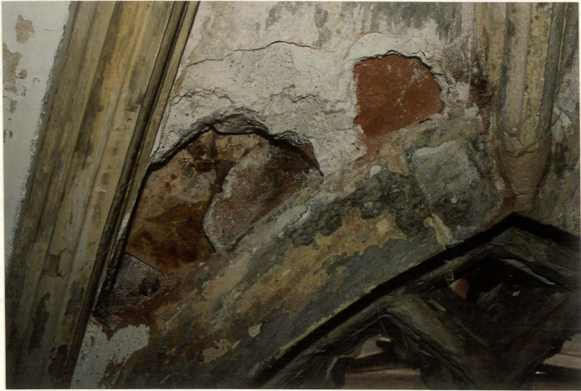
23. Brick infill and plaster over window head at N3.
