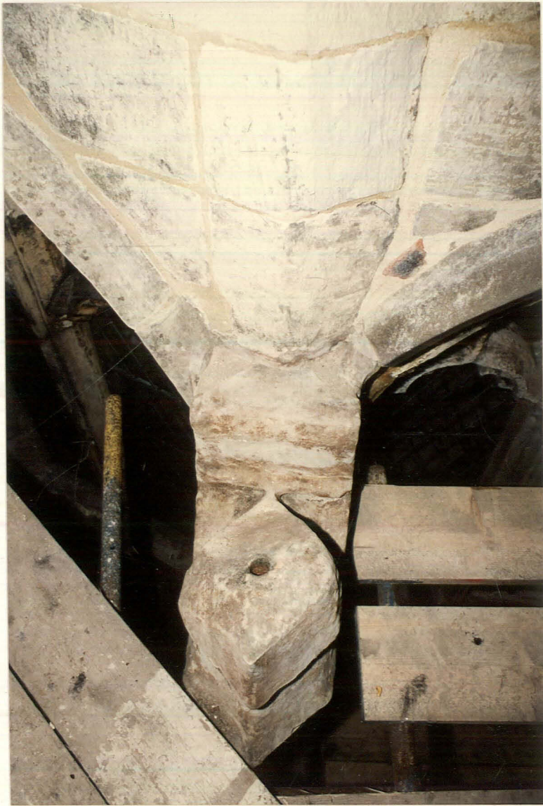
1. Buttress D pinnacle seat and hood springer housing block.
