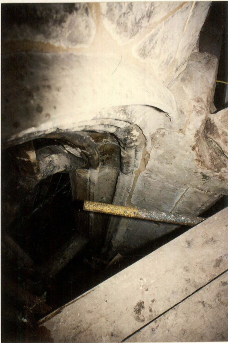
9. X4 window, standard jamb moulding.
