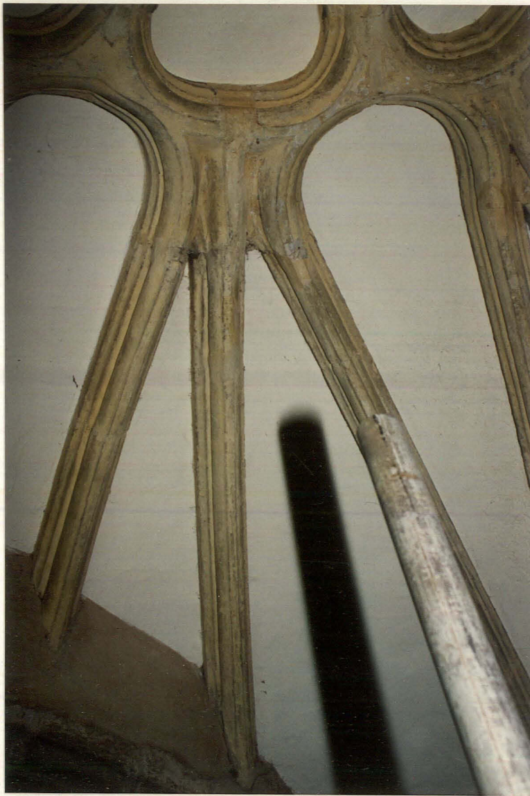
19. Vault, showing 'junction blocks' between inner and outer cells.
