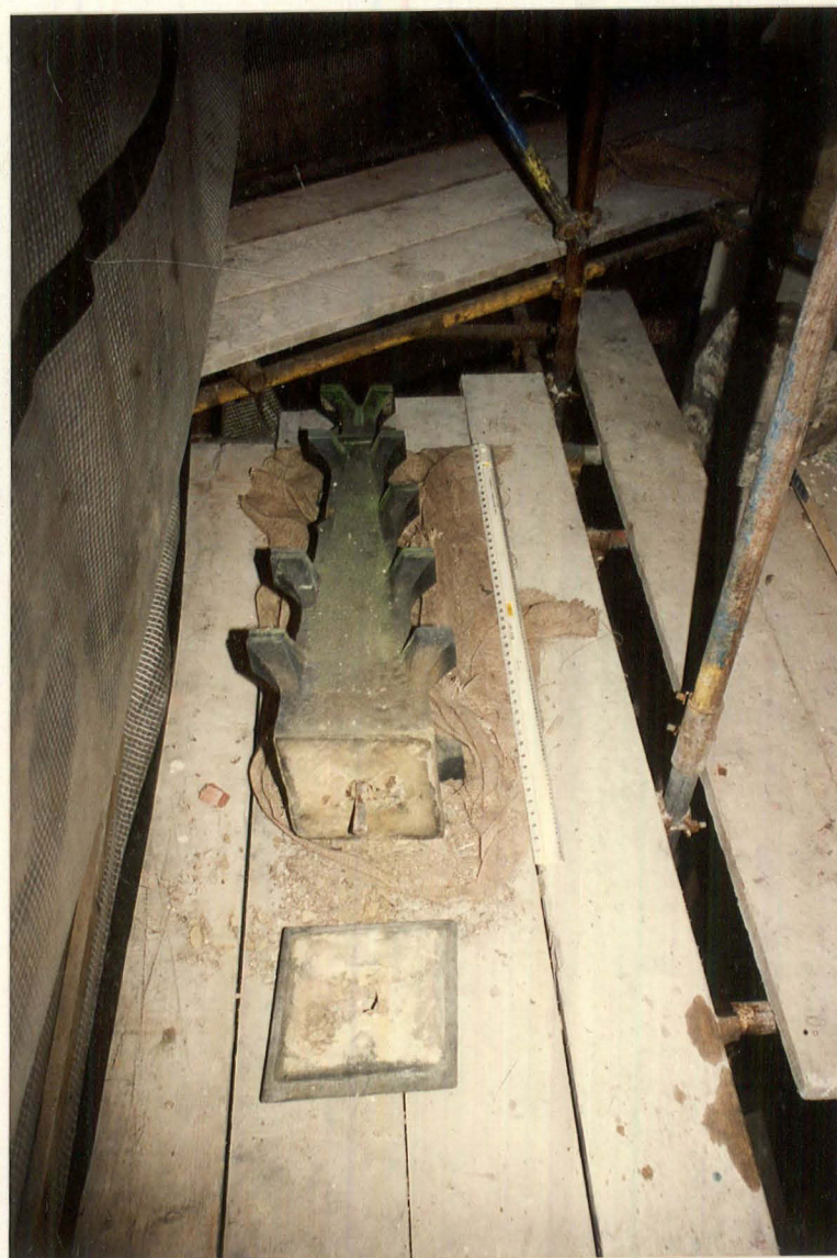
7. Buttress A cap from east, showing springer housing block.
