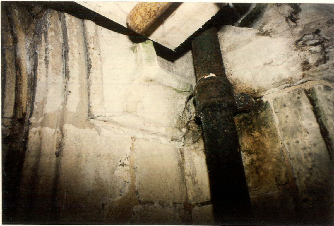
30. X5: Hood-mould terminal 527.
