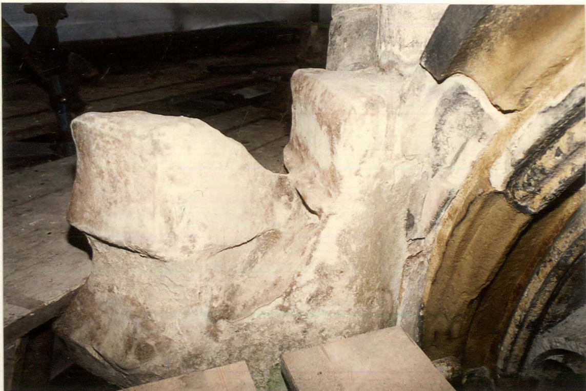
2. Buttress D cap from south, showing original hood springer.
