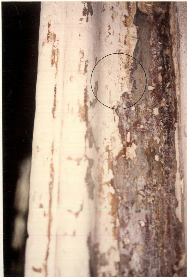
32. Masons marks (type 7) on shaft/jamb block 1233.
