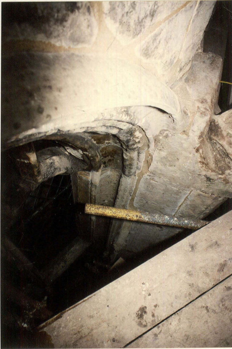
9. X4 window, standard jamb moulding.
