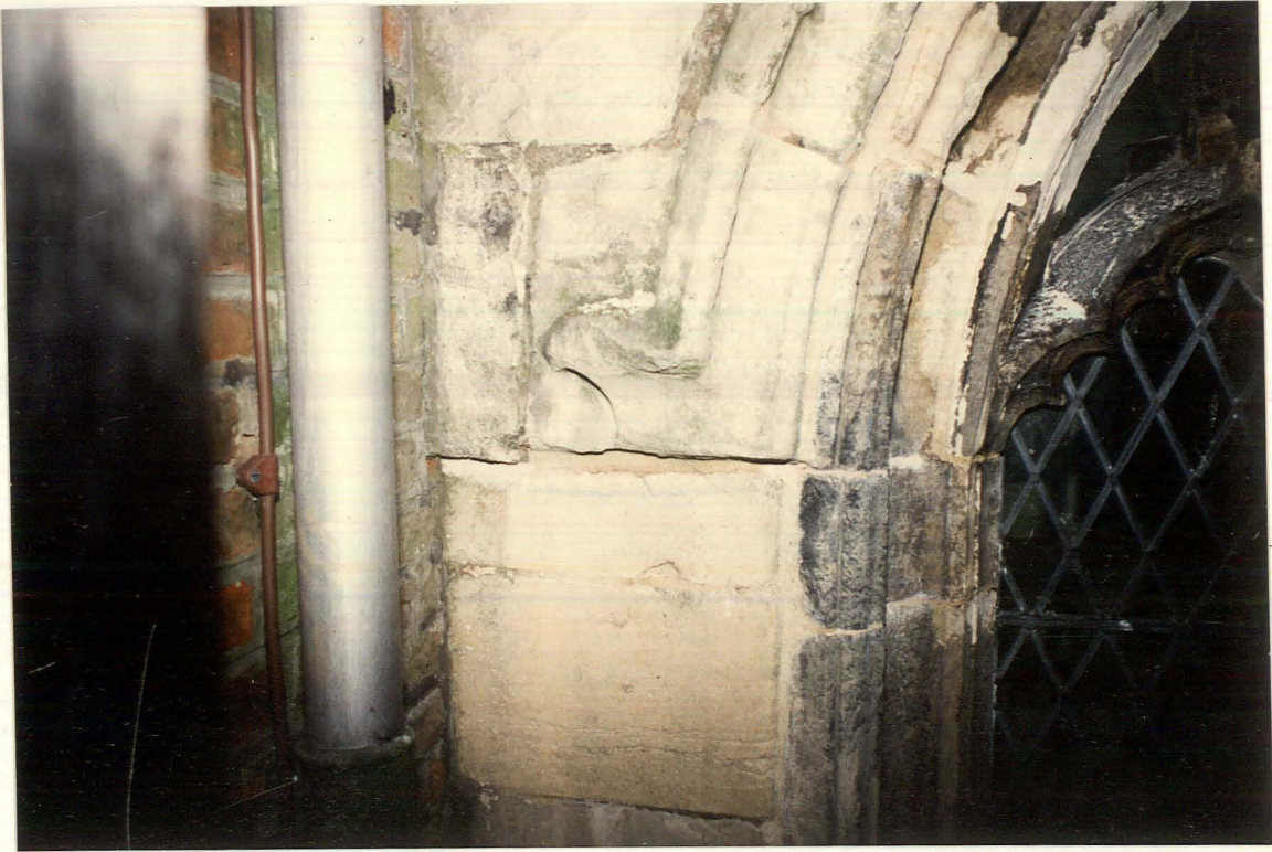
29. X1: Hood-mould terminal 465.
