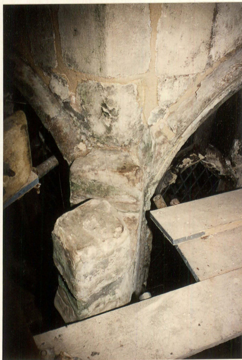
7. Buttress A cap from east, showing springer housing block.
