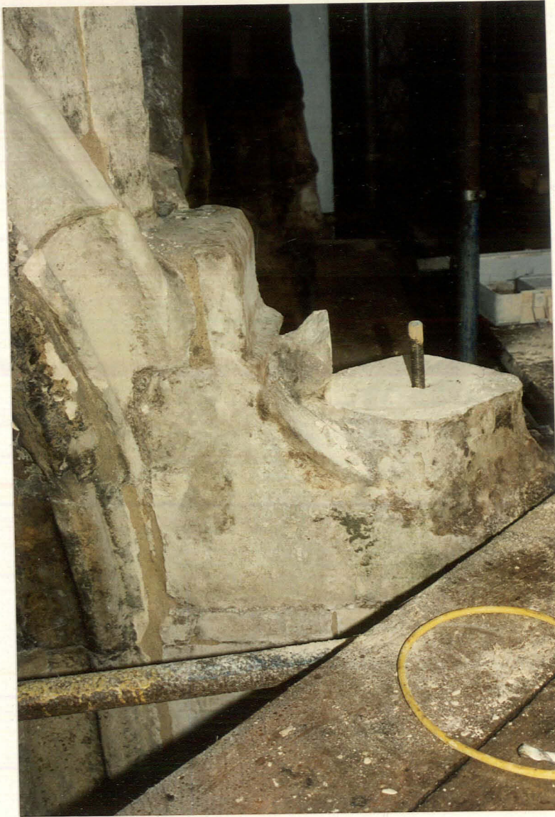
3. Buttress D cap from north, showing (background) original hood springer angle.
