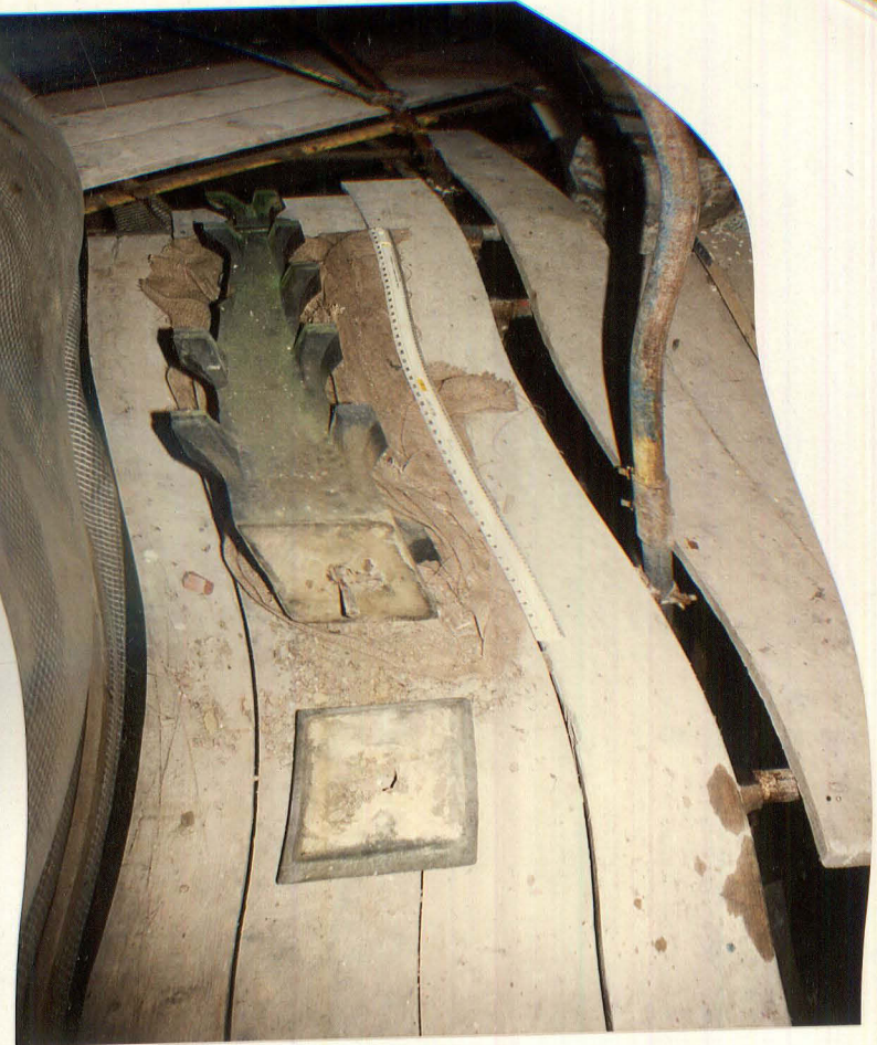
7. Buttress A cap from east, showing springer housing block.
