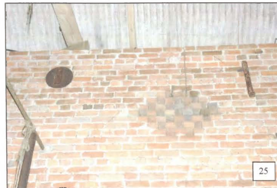
Directly opposite the ground floor doorway in the north wall, a similar door was present on the south side. This comprised a pair of ledged and diagonally braced plank stable-type doors, which originally gave access to the northern crewyard.
