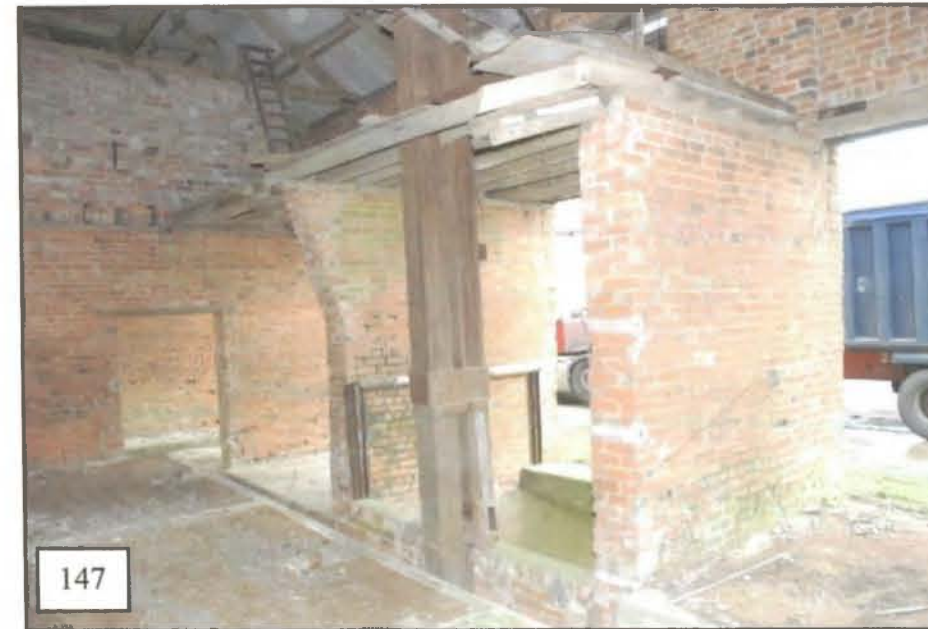
At first floor level, a large grain hopper was constructed over the passage from the yard, with chutes to allow loading of wagons. An overhead grain transport system was also present to transfer the grain from here to the tanked-out area in the western part of the building.
