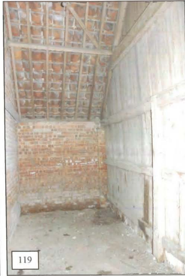
A timber partition, of vertical 7" tongue and grooved planks, separates the eastern bay from the rest of the building. The partition is fixed to the west side of a collar above and a tie-beam lower down, the tie beam being braced with a central 5" square vertical post, which has further horizontal braces both to the wall and to the post of the open-frontage. A three-light window of overlapping panes is present towards the north end of this partition.
