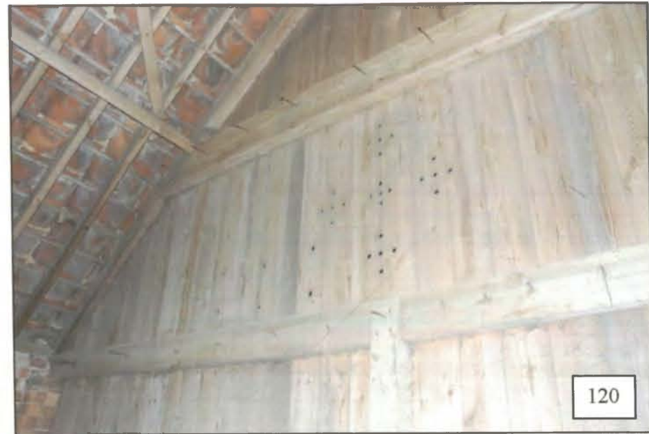
A timber partition, of vertical 7" tongue and grooved planks, separates the eastern bay from the rest of the building. The partition is fixed to the west side of a collar above and a tie-beam lower down, the tie beam being braced with a central 5" square vertical post, which has further horizontal braces both to the wall and to the post of the open-frontage. A three-light window of overlapping panes is present towards the north end of this partition.
