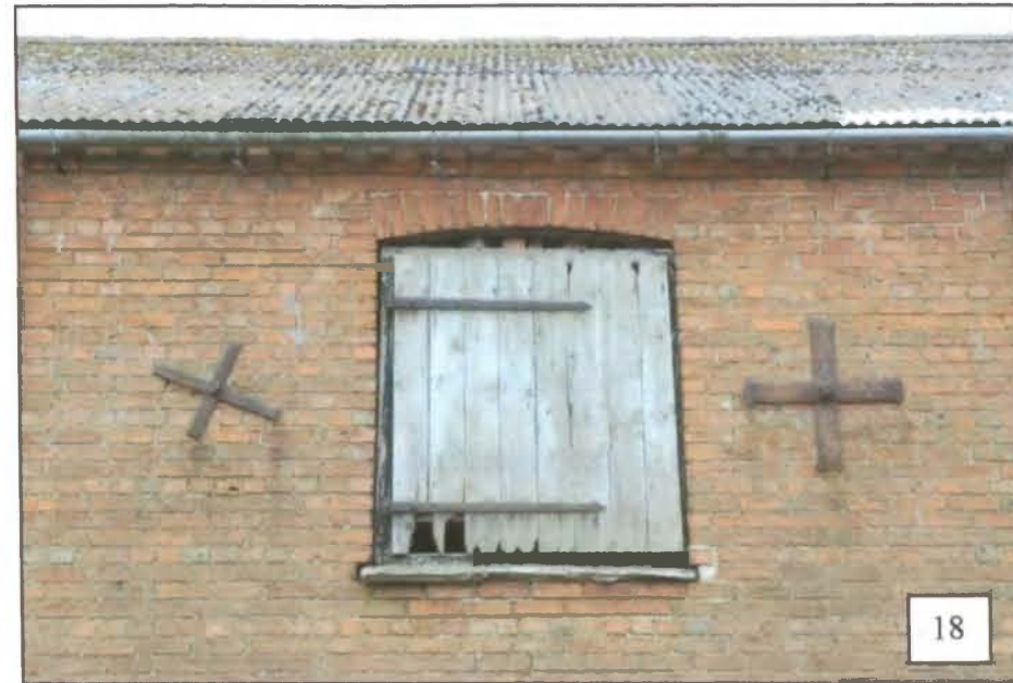
The western part of Building A does retain some original features: on the north side, the large stable-type door at ground level is of ledged and diagonally braced beaded plank construction, with long strap hinges. The first-floor ledged and diagonally braced plank loading door is in an original position, but may itself be a replacement.
