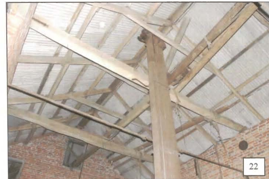
The roof, although now reclad in corrugated asbestos cement panels, retains the heavy timbers of its original construction. It is of collar rafter construction with chamfered collars, a ridgeboard and staggered butt-purlins, their pegged tenons projecting through the rafters. In the western part, which has lost the stiffening effect of its first floor, four three-part iron tie-rods span the structure, centrally suspended from the nearest tie-beam or collar.
