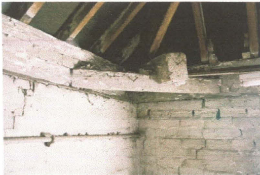
Dragon bracing at the north-east corner
