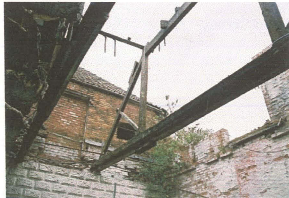
Building 2 -North Truss
