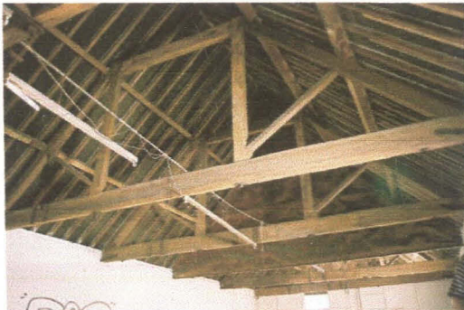
Queen Post Roof Trusses
