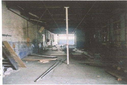
Building 1, ground floor looking south
