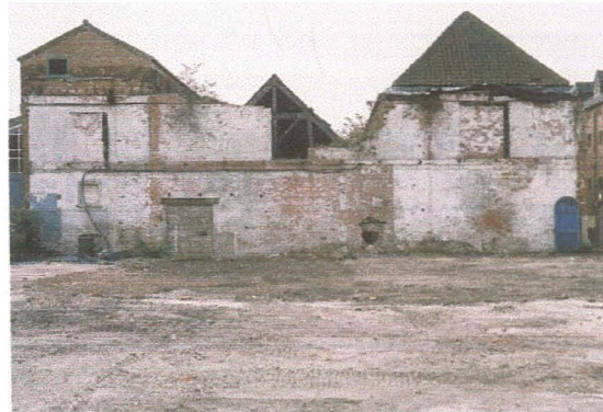
The North elevation
