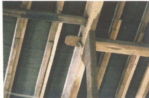
Detail of butt purlins
