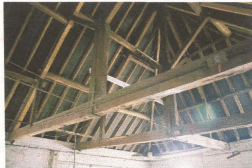
King Post roof trusses at the south end
