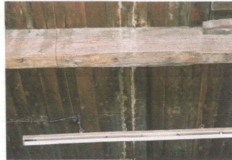
Building 1 Beam with simple stopped chamfer either side of spine beam (removed). Owing to the length of the building, the spine beam must have been composite and supported at intervals by verticals
