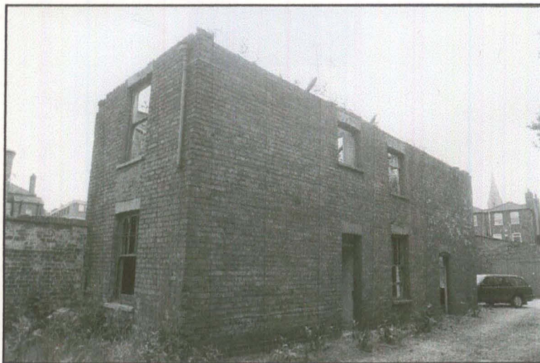
The Foreman's House looking north-east
