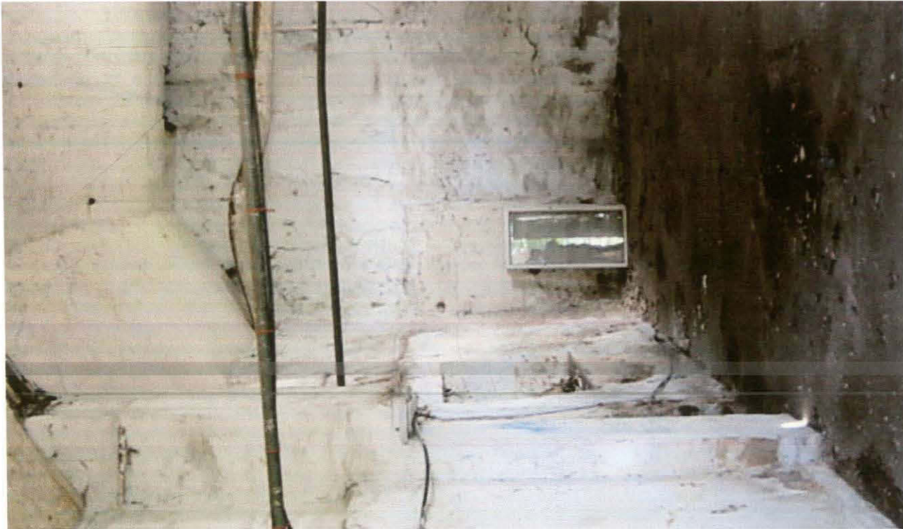
12. Garage - View from entrance, showing the white painted/rendered walls, lath & plaster ceiling & timber tie.
