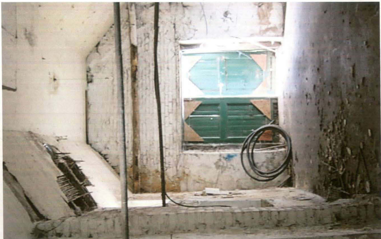
11. Garage - View towards entrance showing the white painted brick walls, lath & plaster ceiling and timber tie.
