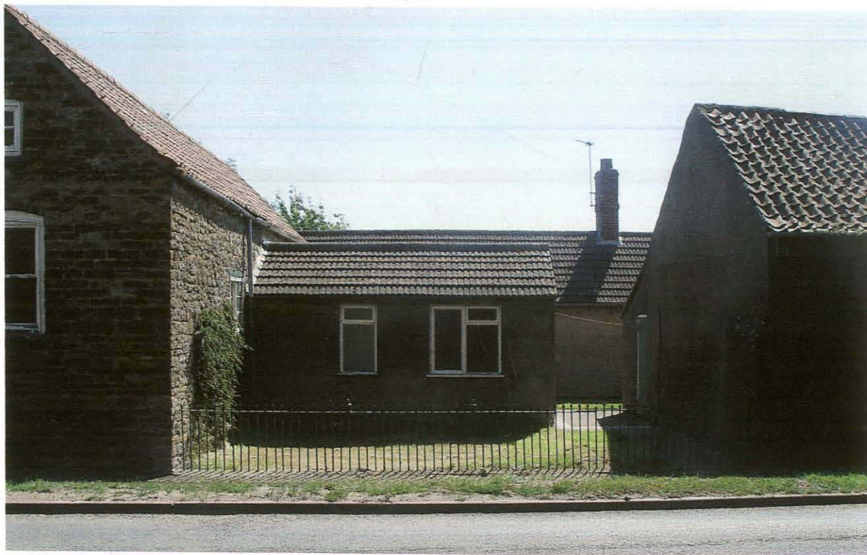
5. Grooms Cottage - Western Elevation looking from Lincoln Road. Note - 1960's rendered bathroom extension.
