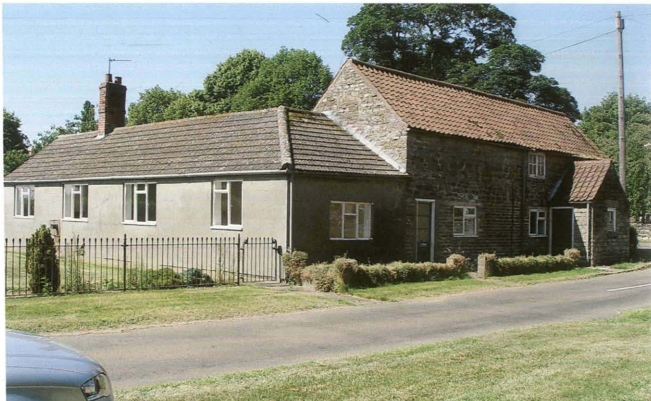
1. Grooms Cottage - Eastern & Northern Elevations looking from Cammeringham Hill. Note - 1960's rendered extension on the Eastern Elevation.
