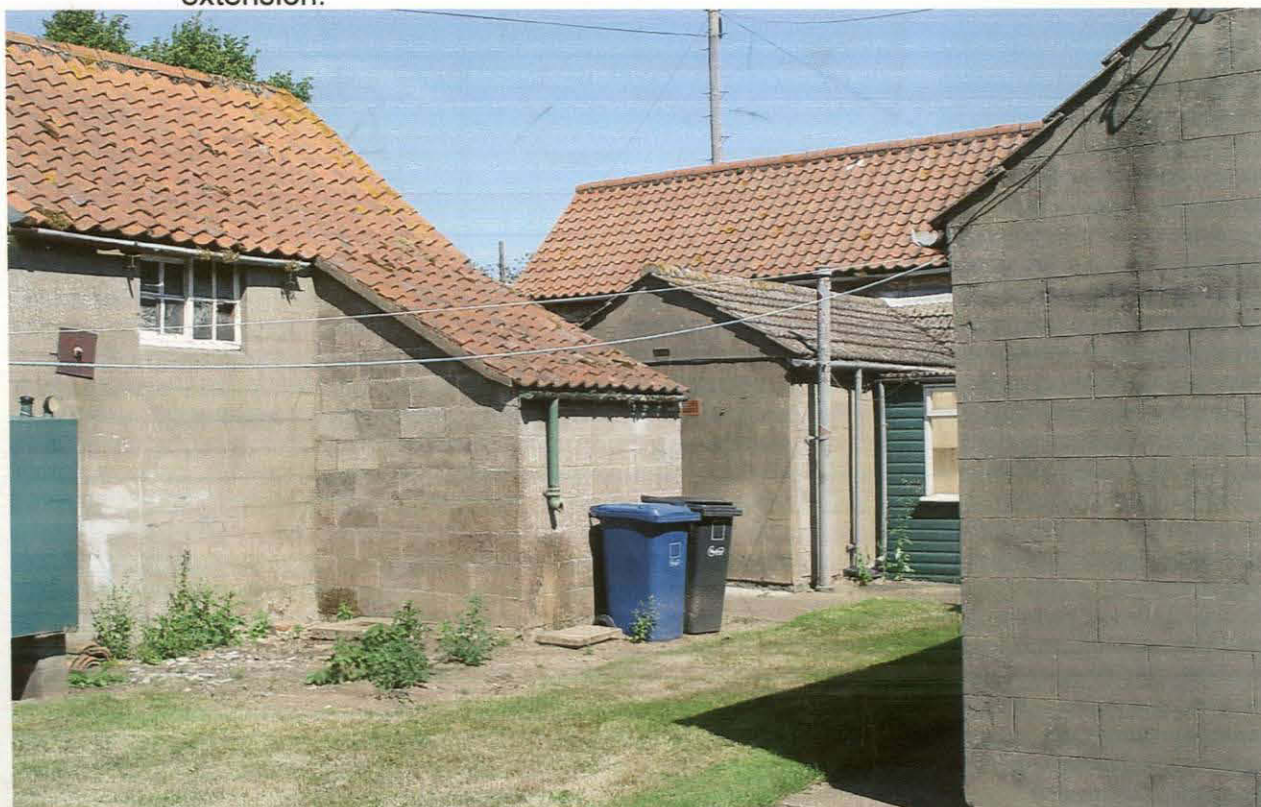
10. Garage - Northern end of Eastern Elevation of Grade II listed Garage showing late 19th century additions which were used as a coalhouse.
