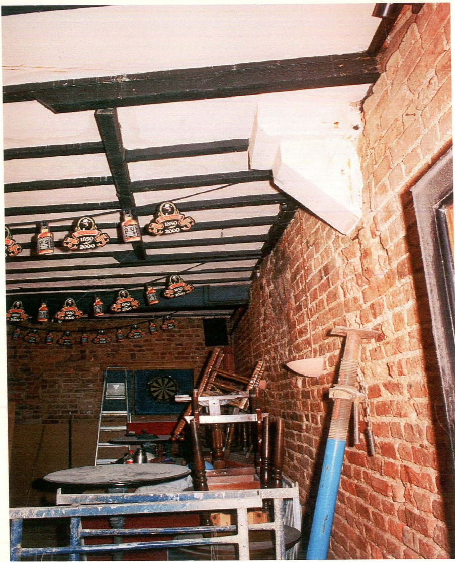
Pl. 9 West wall of bar, looking south showing corbel supporting hearth above. Note blocked door in south wall at far end of room.
