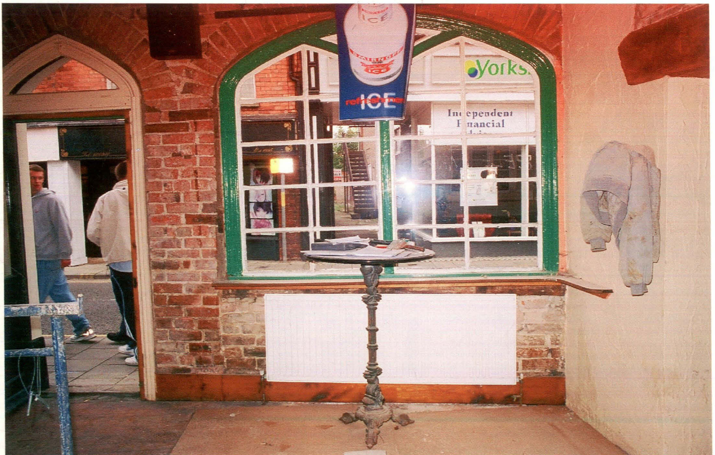
Pl. 8 North wall of bar, showing entrance onto Mercer Row and window with blocking beneath.
