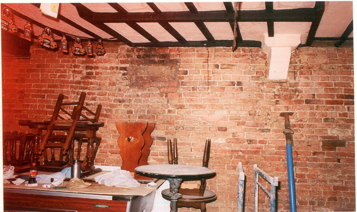
Pl. 10 West wall of bar, looking west showing corbel supporting hearth (right) and disturbed Brickwork (left) marking position of second corbel.
