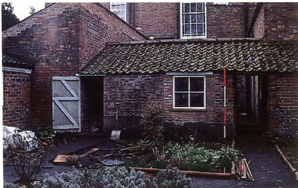
Pl. 1 Exterior of recorded building. Looking south.
