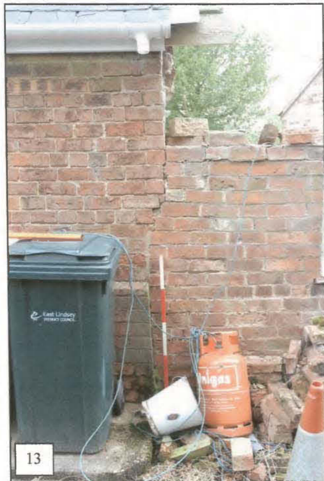
The joint between the brickwork of Lizzies House and the eastern wing of 'Greenhaven' clearly demonstrated that Lizzies House had received its brick cladding before the construction of the neighbouring property. At the east end of the south elevation, several squared limestone blocks were present at foundation level.
