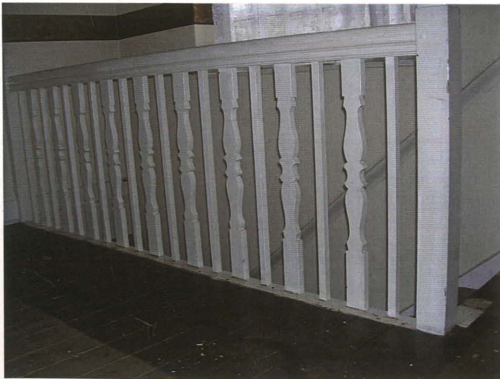
Pl. 44 Detail of the stair showing the flat-sectioned balusters
