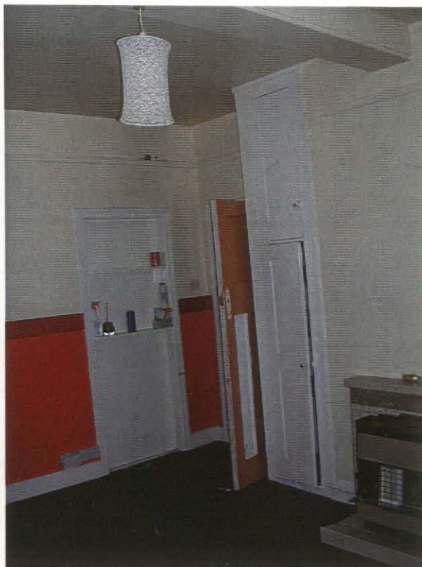
Pl. 36 Blocked door to kitchen (shelved) in west wall of landlord's living room
