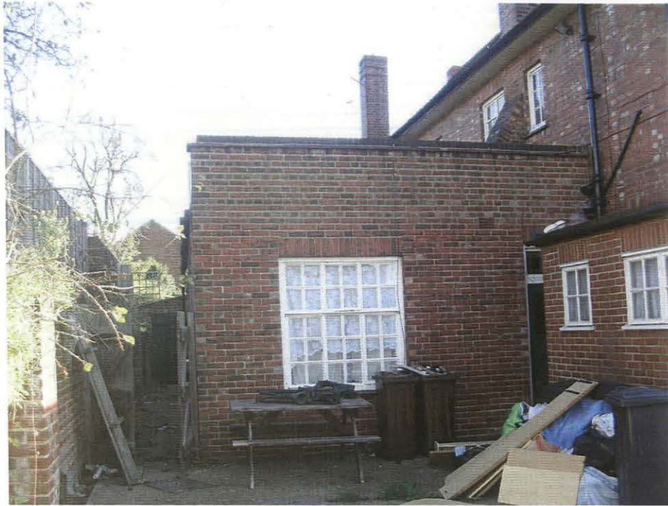
Pl. 13 West elevation of single storey block on north side of pub. Note added parapet marked by change in mortar colour.
