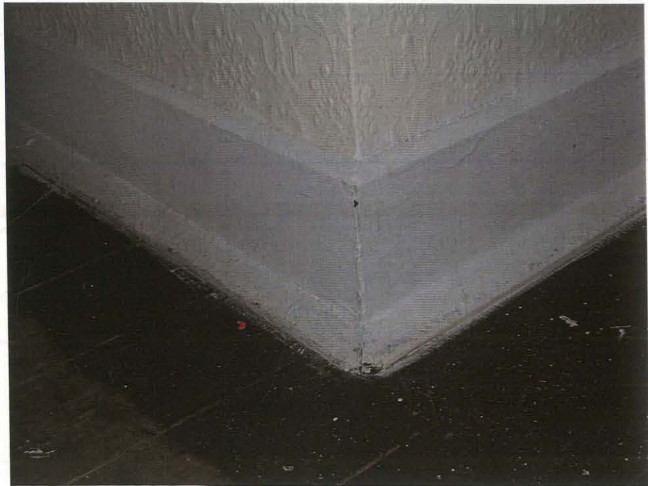
Pl. 45 Detail showing skirting board
