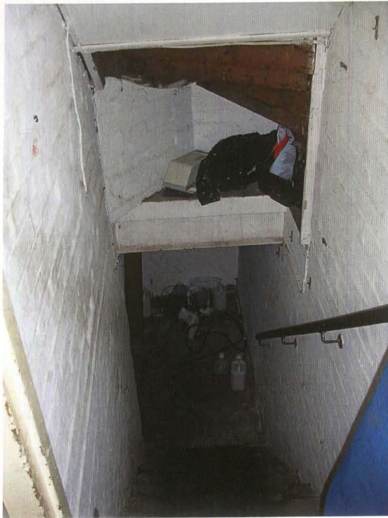
Pl. 37 Steps to cellar, looking west.
