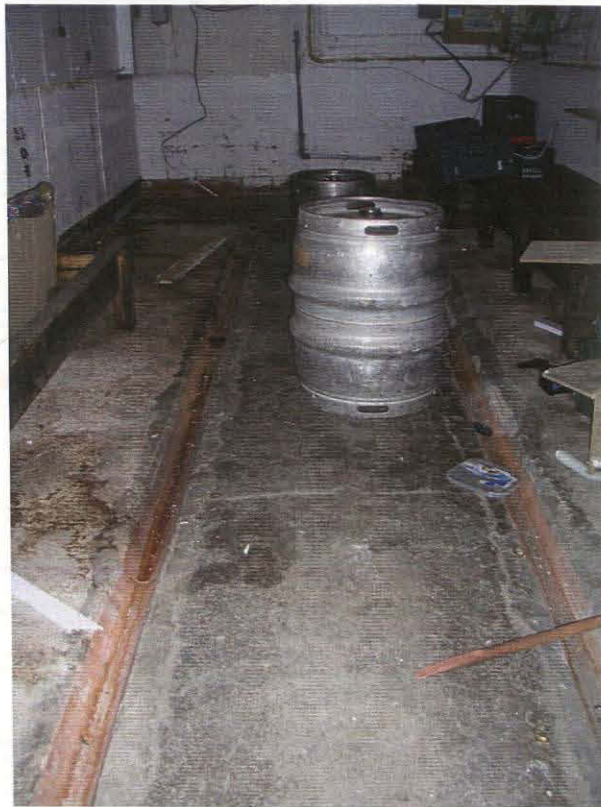
Pl. 39 The cellar south half, looking east.. Note drainage gullies in floor
