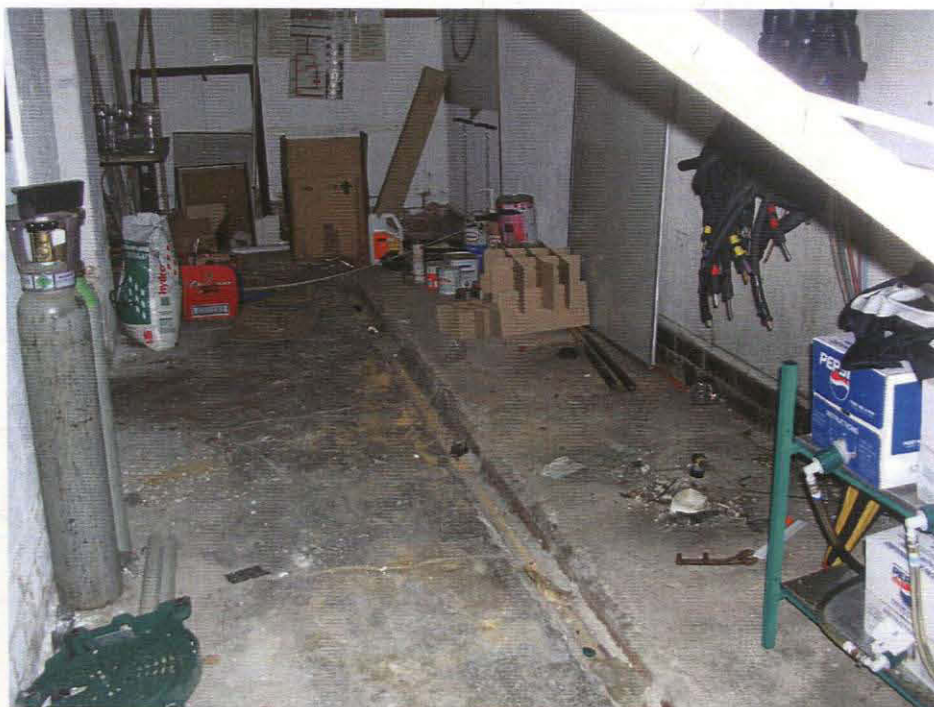
Pl. 40 The cellar, north half, looking east
