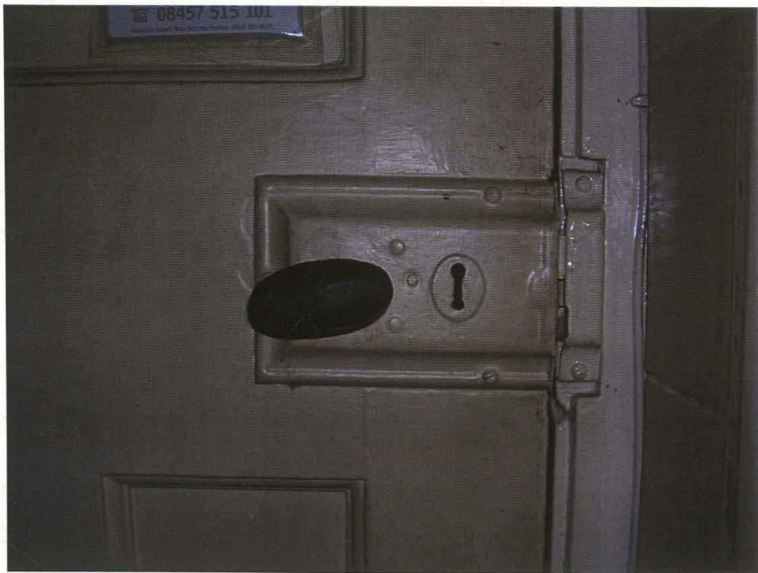
Pl. 16 Original handle and lock on door to rear lobby
