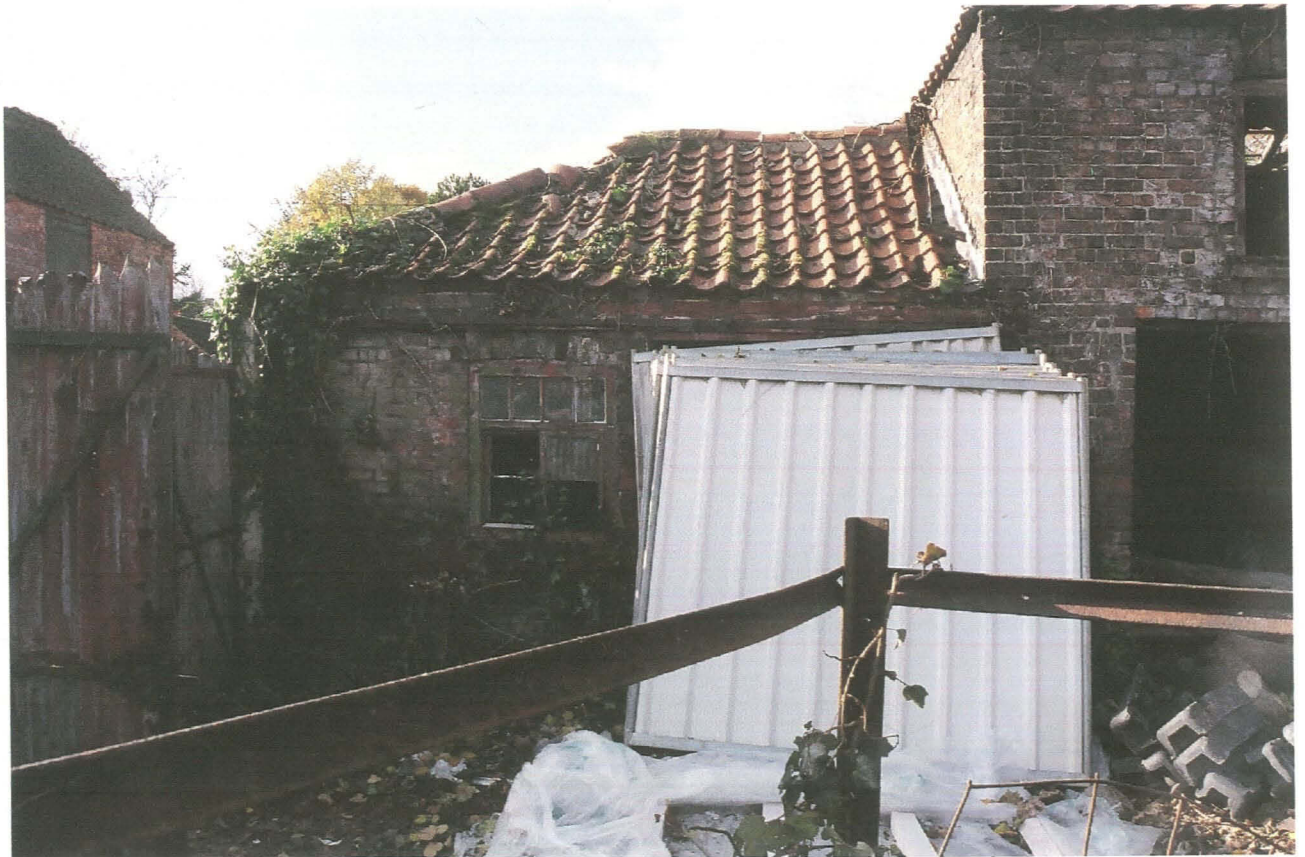
PI. 6 Building 3, east elevation.
