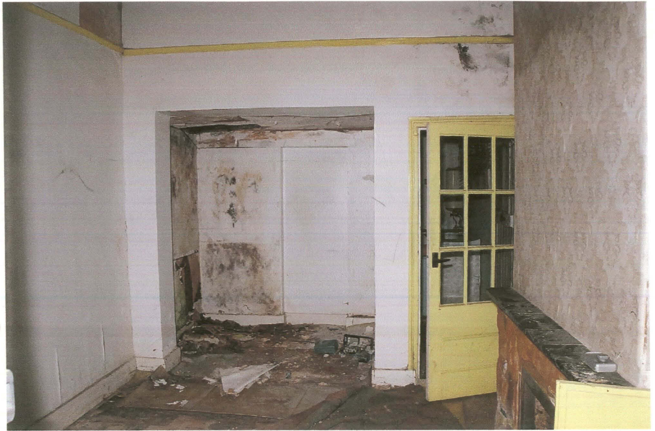
PI. 27 Building 9, ground floor interior, looking south.
