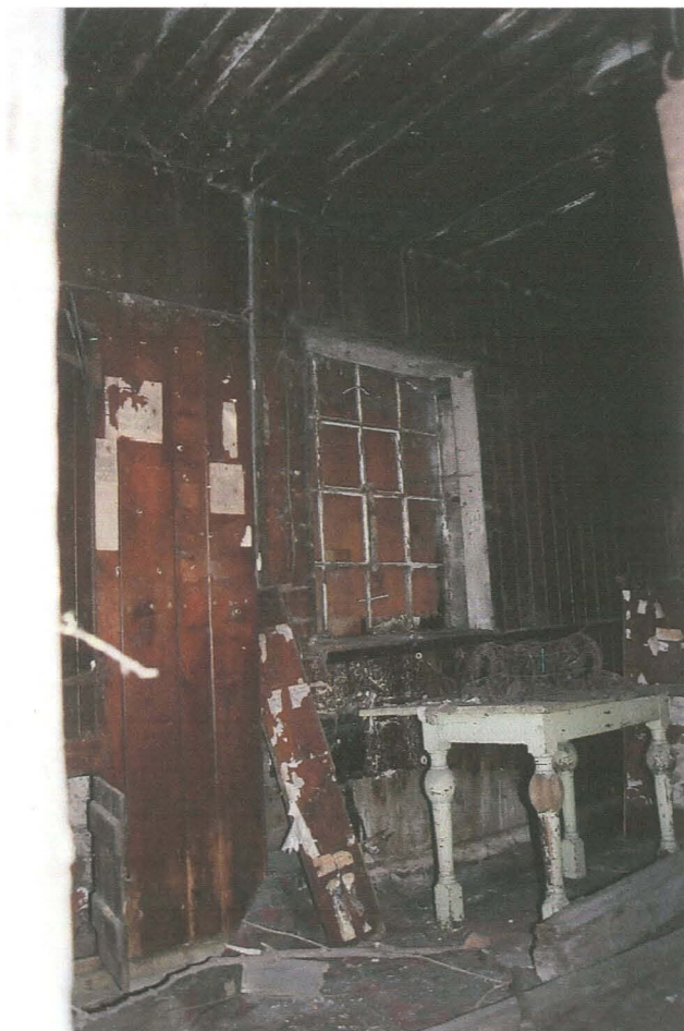
PI. 8 Building 3, interior view looking south showing blocked window and tongue and groove panelling.
