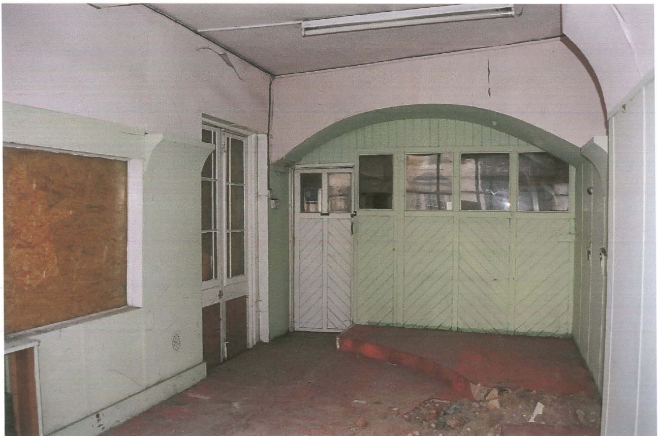
PI. 34 Building 11. Ground floor, east room, showing hardboard cladding concealing brick arch, with French windows in east elevation. Looking south.
