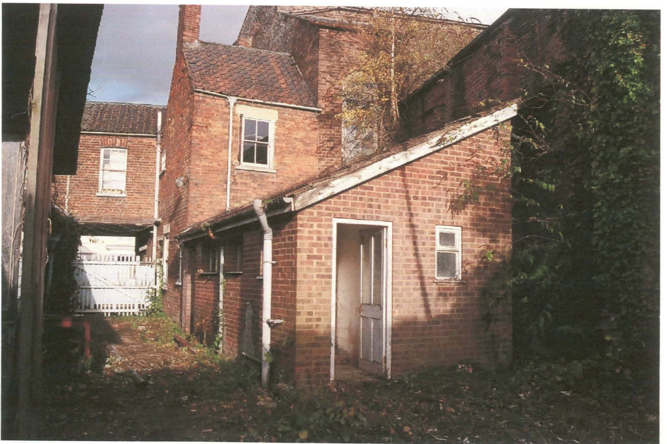
PI. 20 Building 7, view north.
