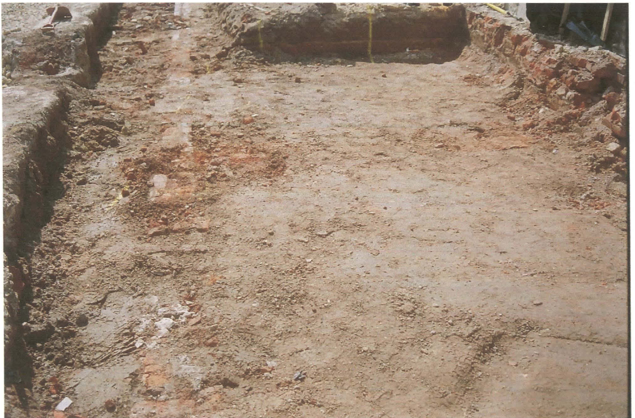
PI. 46 Reduced surface below No. 13 Market Street, showing the brick internal wall foundation, formerly a front wall (looking south).
