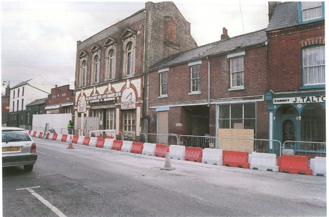
PI. 31 Building 11, north elevation overlooking Market Street.
