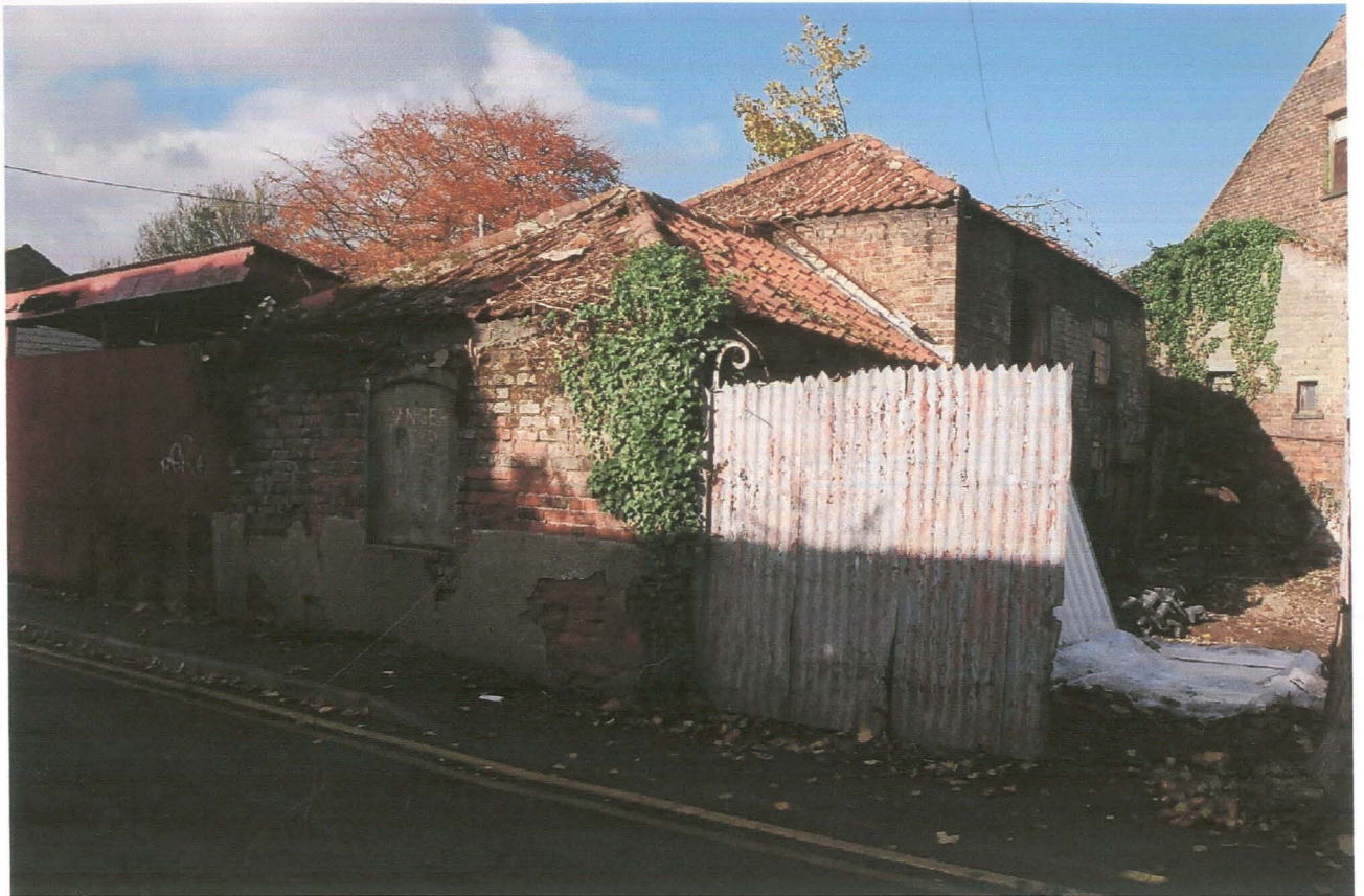
PI. 7 Building 3, south elevation, showing blocked window.
