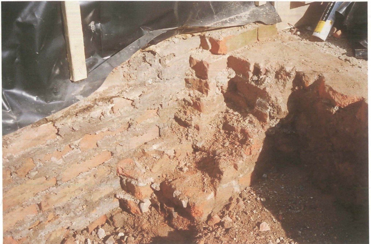
PI. 45 Brick foundations for western wall of No. 13 Market Street, abutted by later wall of No. 15 Market Street (looking west).
