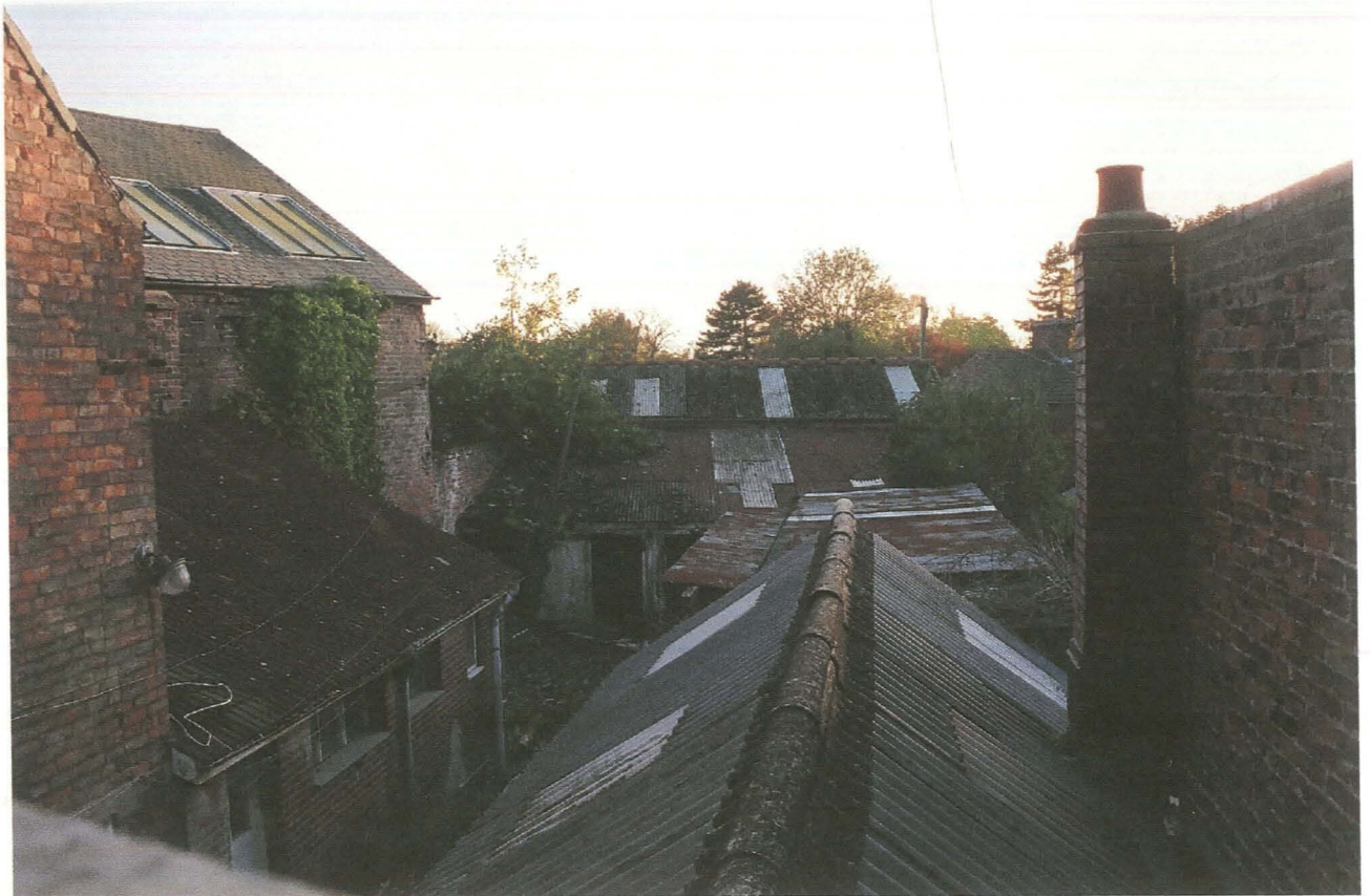
PI. 13 General view of west courtyard looking south towards workshops (Buildings 5 and 6).
