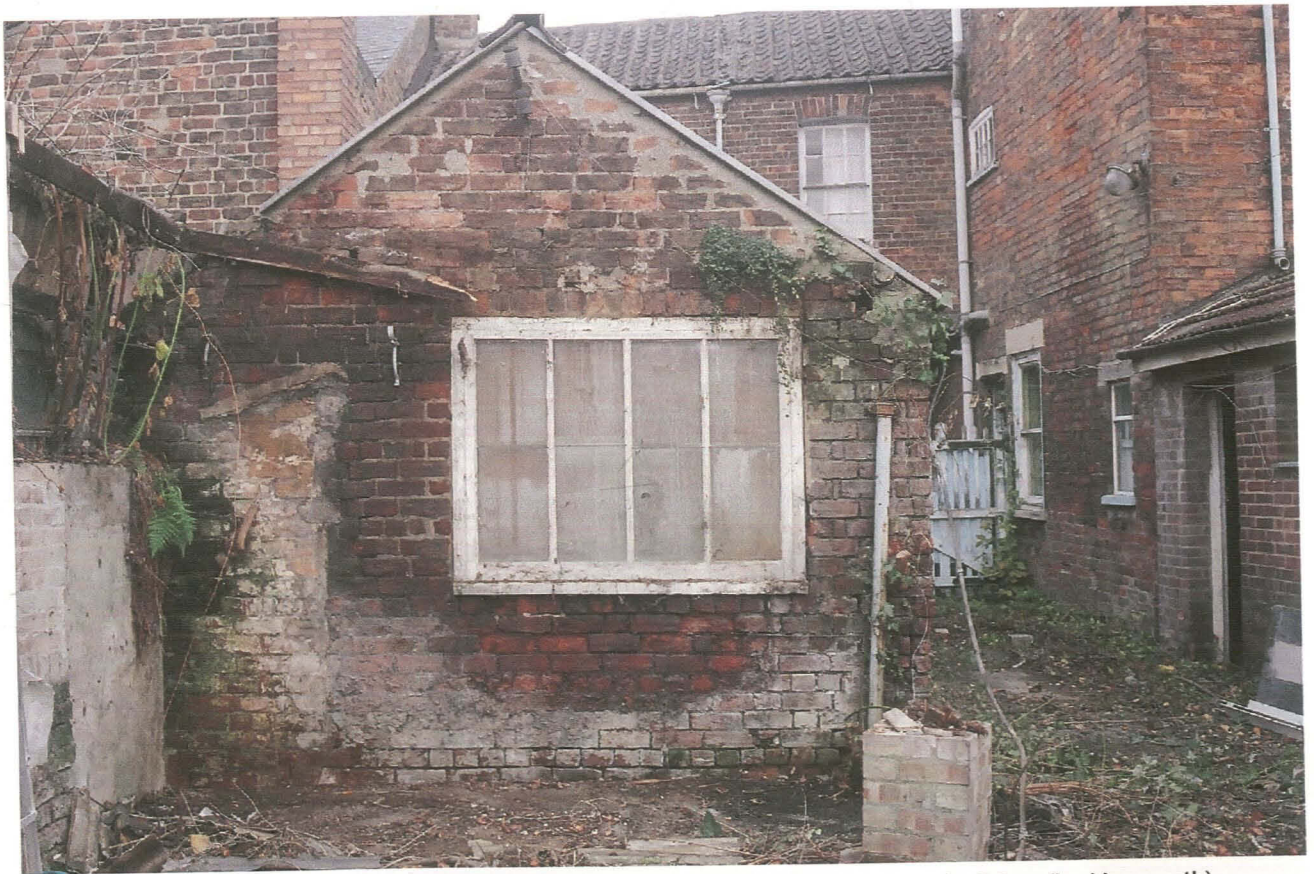
PI. 50 Rear wall of No. 13 Market Street, showing scar of demolished lean-to building (looking north).
