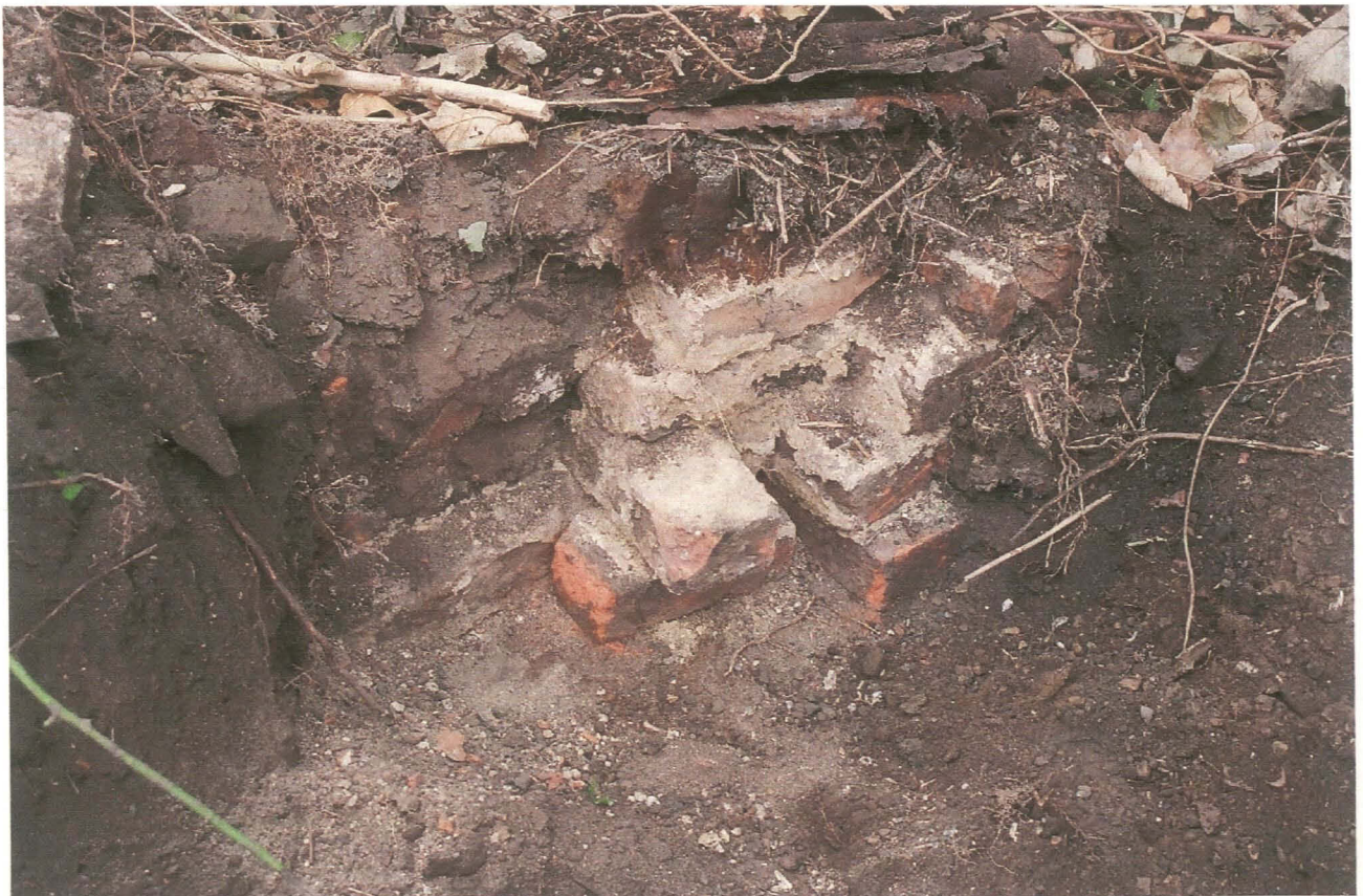
PI. 54 Buried wall foundation to rear of No. 7 Market Street.
