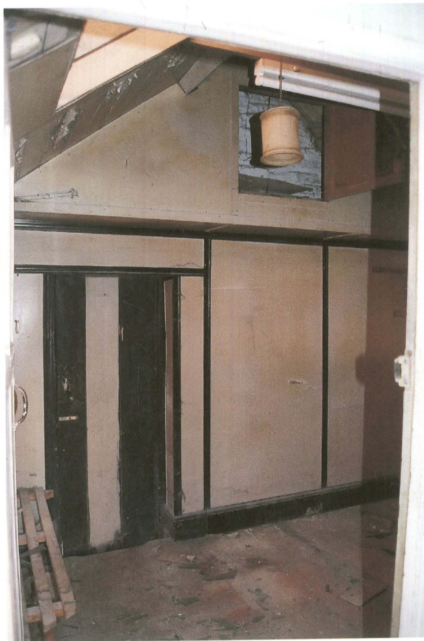
PI. 25 Building 10, interior, looking south, with door leading to Building 8.
