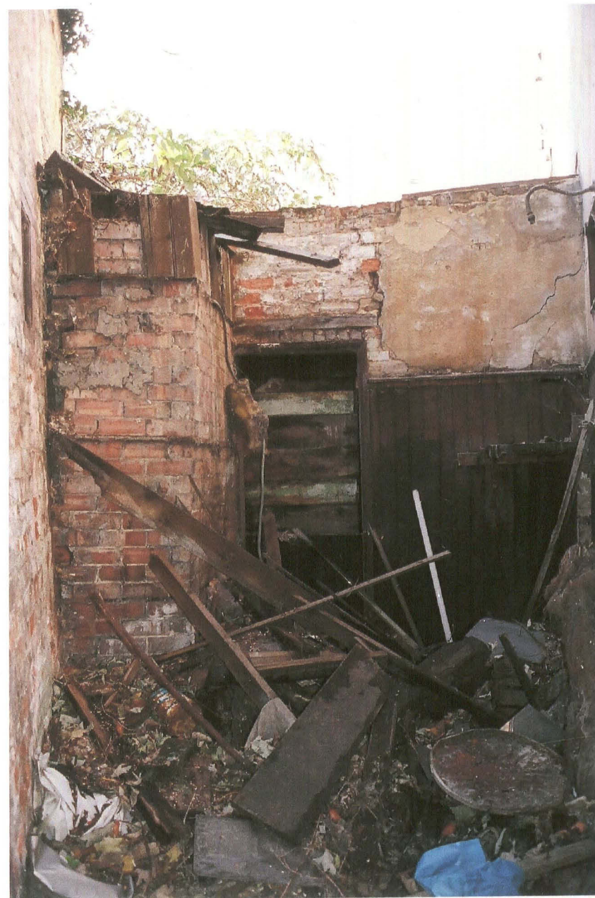
PI. 12 Building 4, room 4a with inserted 20 th century toilet, access from room 4b.
