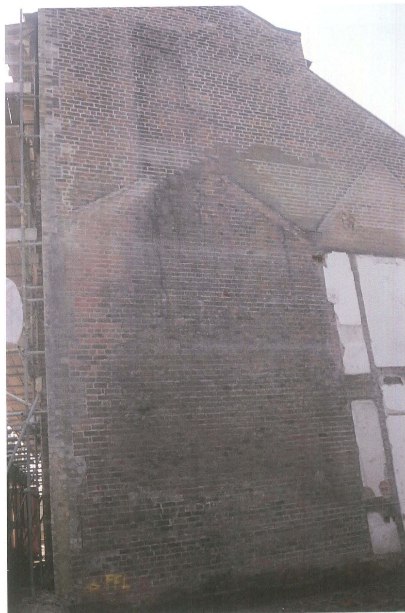
Pl. 40 Western gable end of the Market House, showing the outline of the demolished No. 11 Market Street (looking east).
