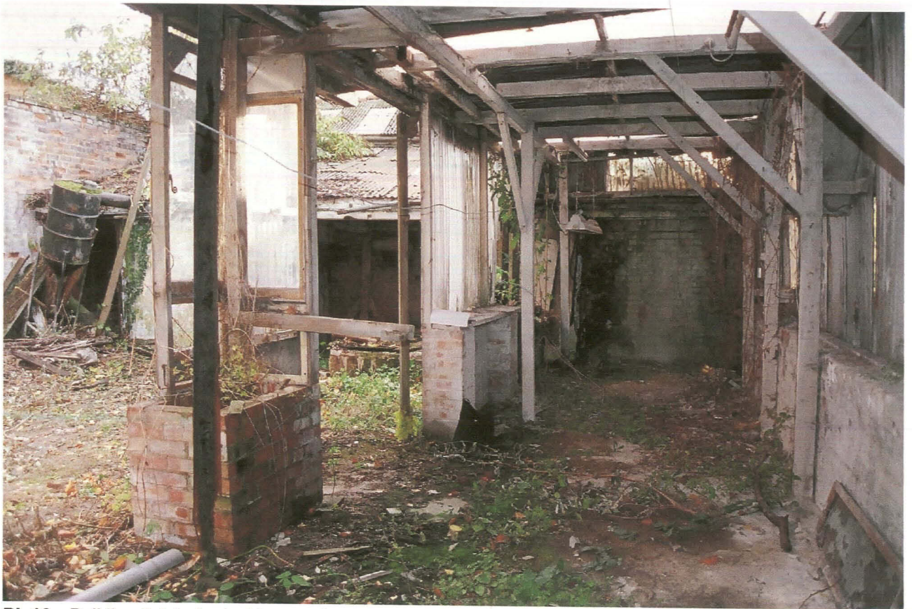
PI. 19 Building 6, interior looking south, showing modern brick plinths along east wall.
