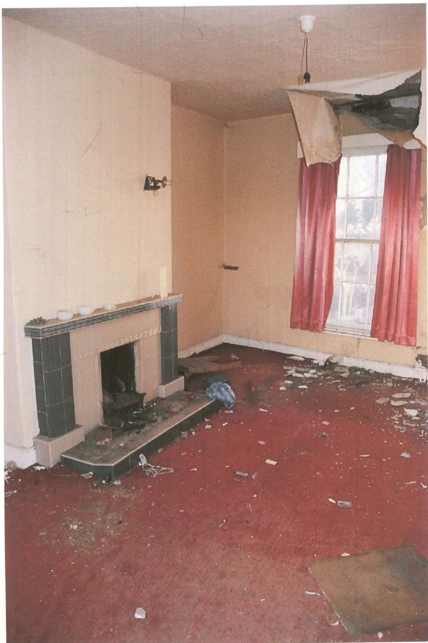
Pl. 39 Building 11, west bedroom, looking north-west.
