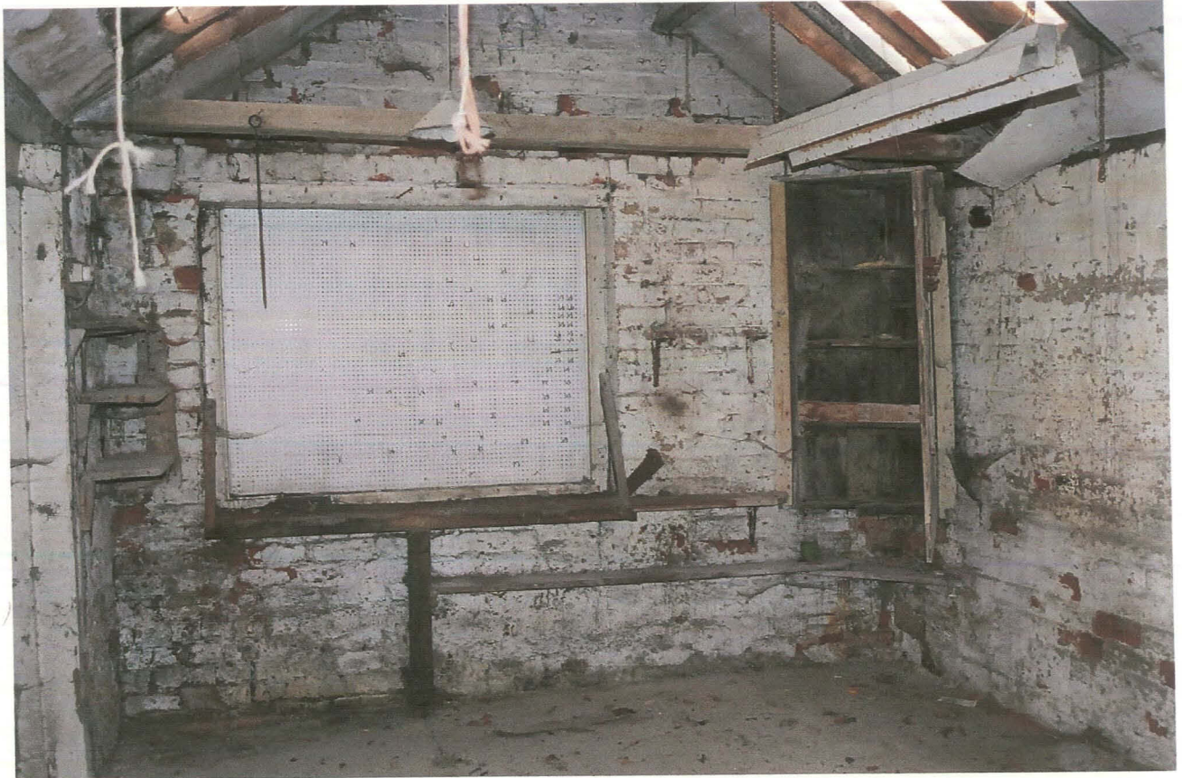
PI. 23 Building 8, interior, looking south, showing corner cupboard.
