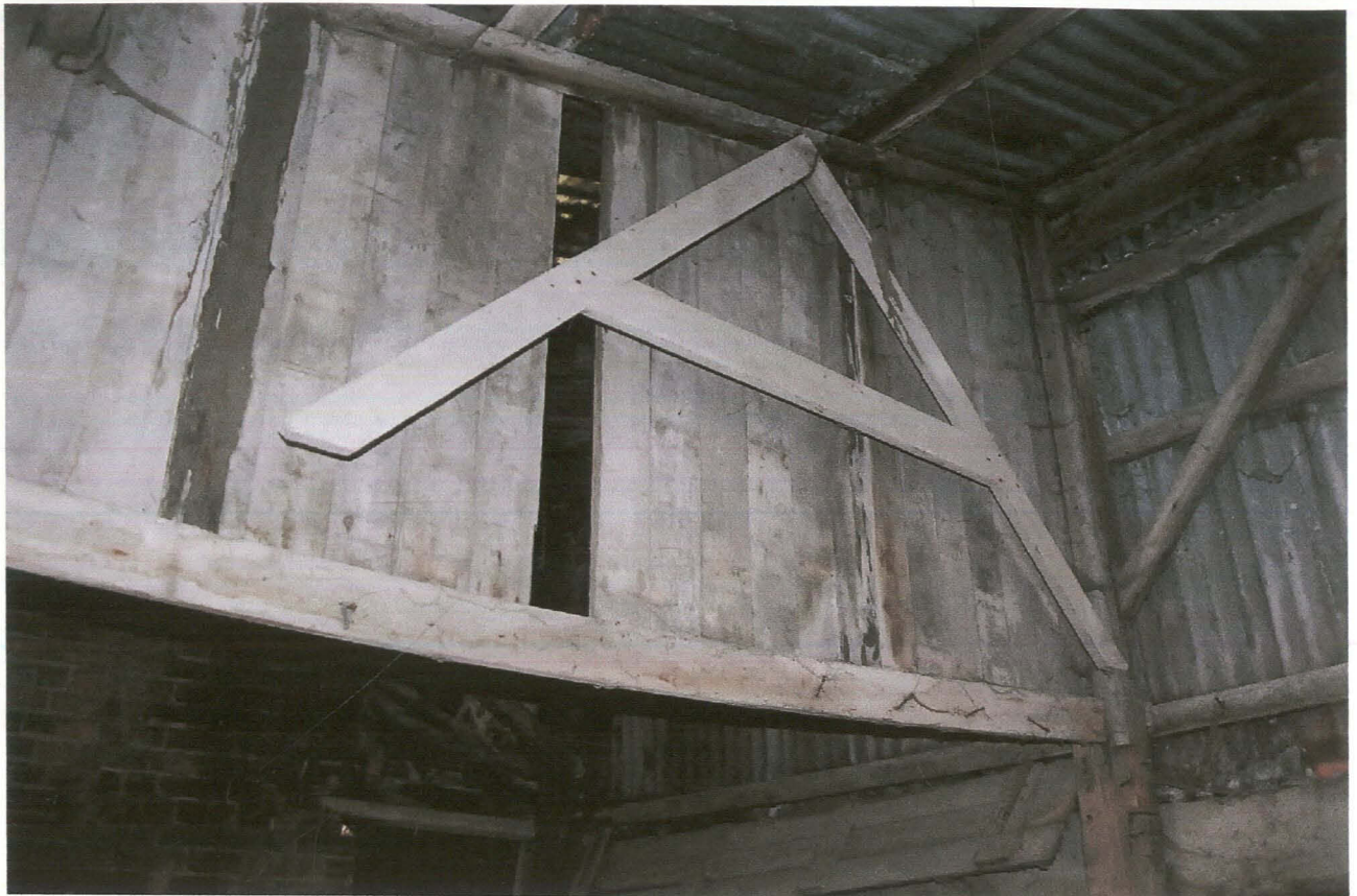
PI. 15 Interior partition wall of Building 5, with A-square template hanging on the wall.
