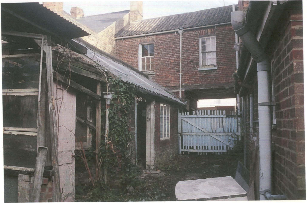
PI. 21 Building 8, to north of Building 6 in foreground, looking north.
