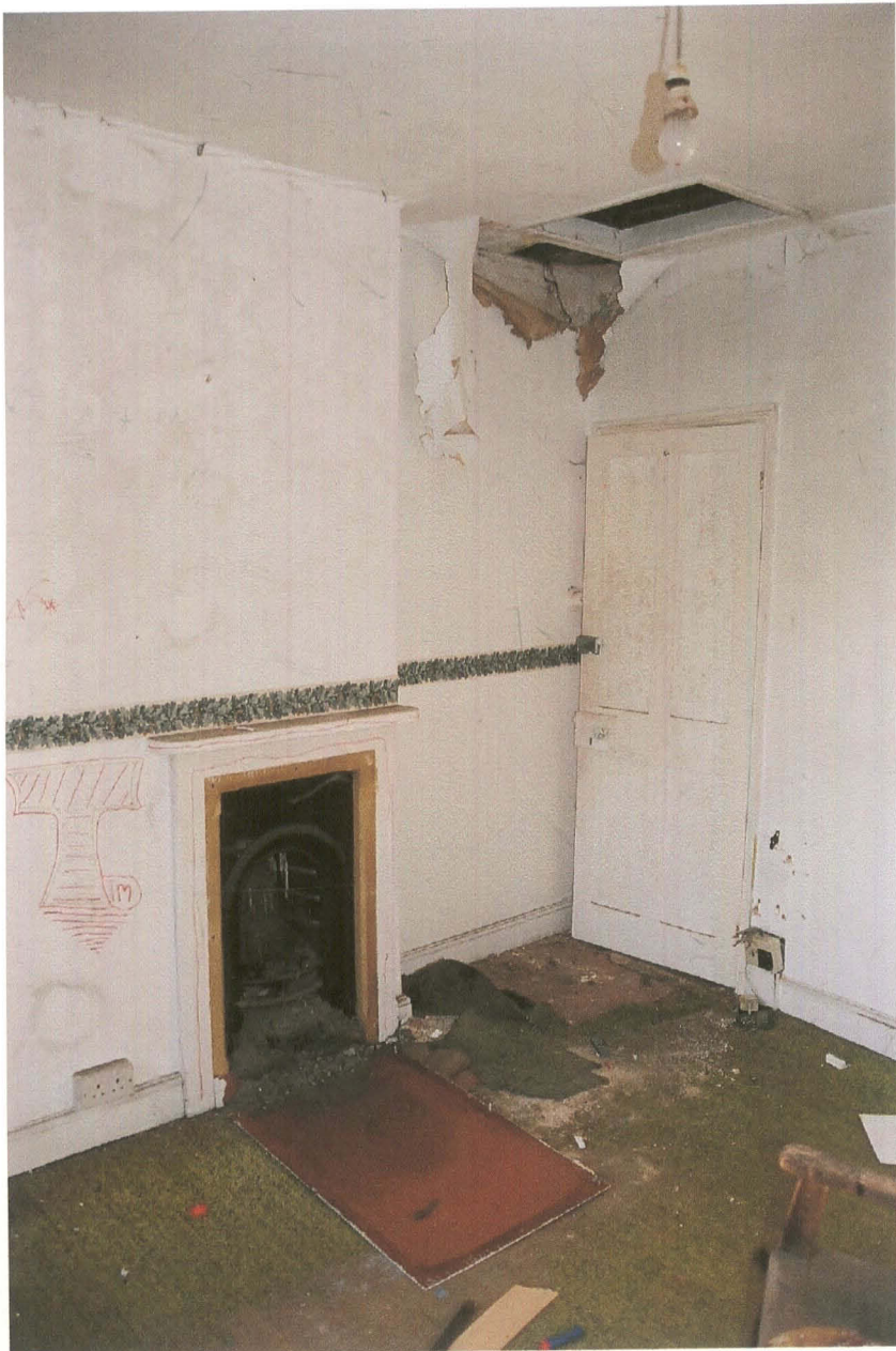
PI. 29 Building 9, first floor bedroom, looking west.
