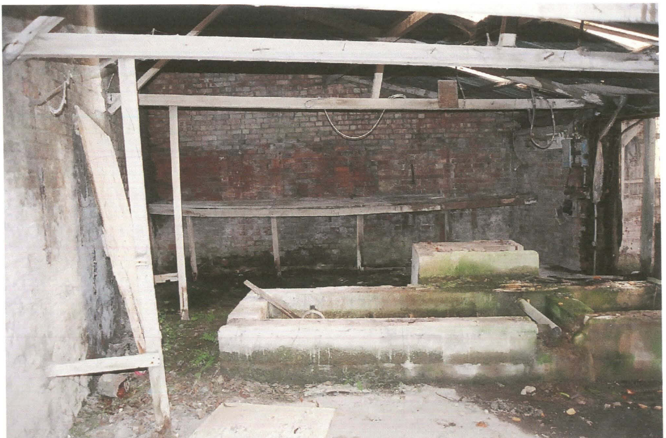
PI. 14 Interior view of Building 5 showing breeze block saw mill, with bench along east wall.
