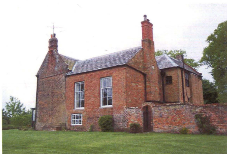
Figure 16 General arrangement from north-east showing phased construction and abutting garden wall.
