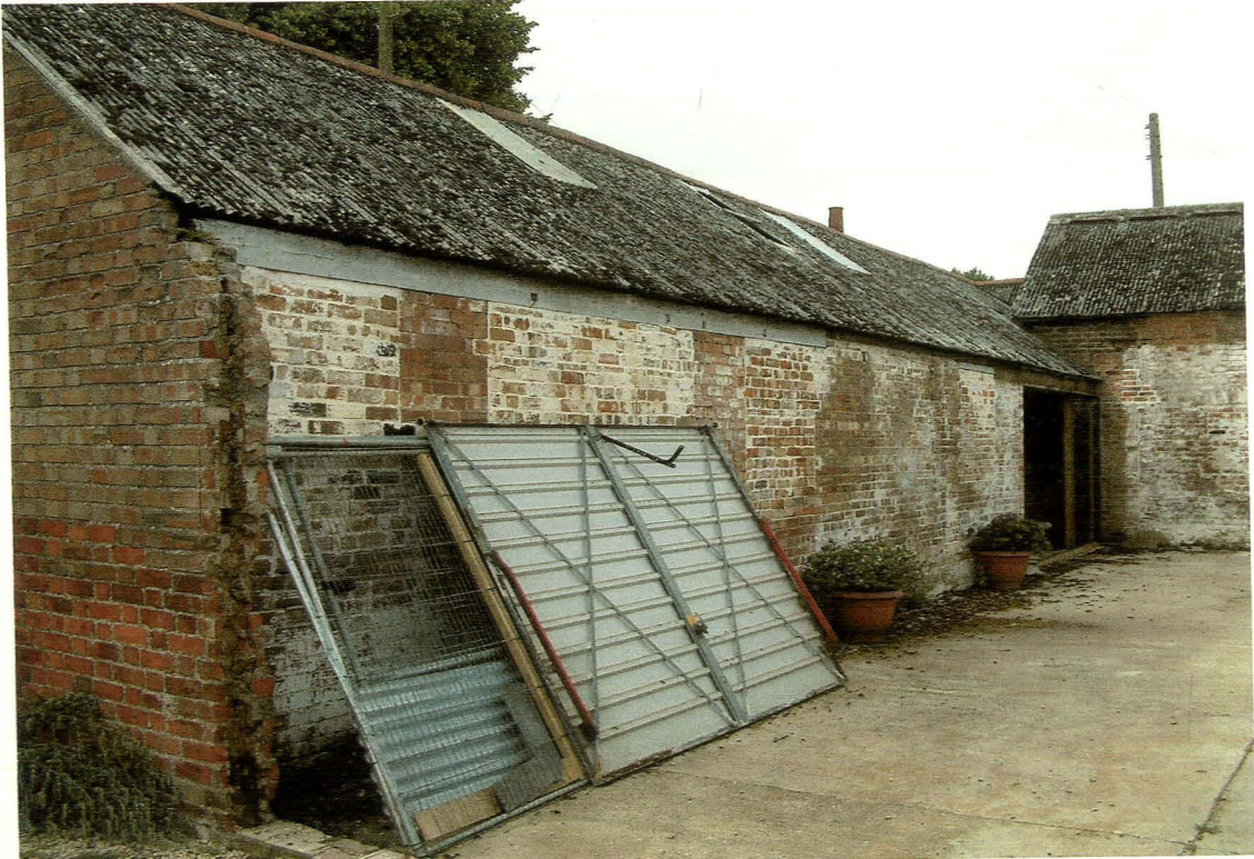
Plate 8. Outbuilding 1 looking east.
