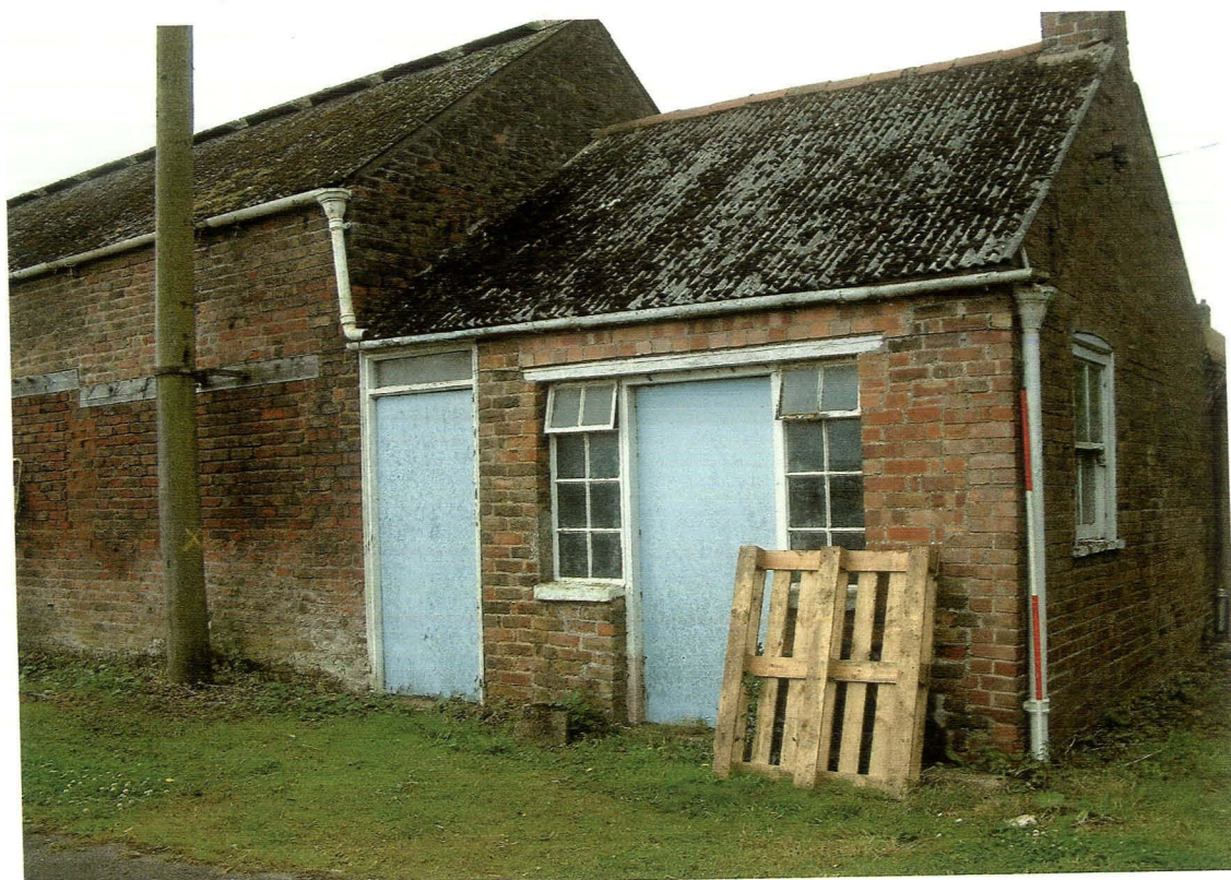
Plate 3. Small staff cottage on northern end of outbuilding 2.
