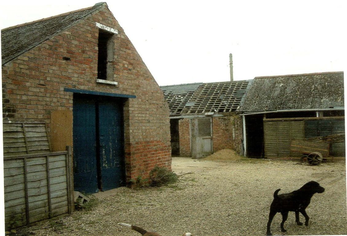
Plate 7. Gable end of outbuilding 1 looking south.
