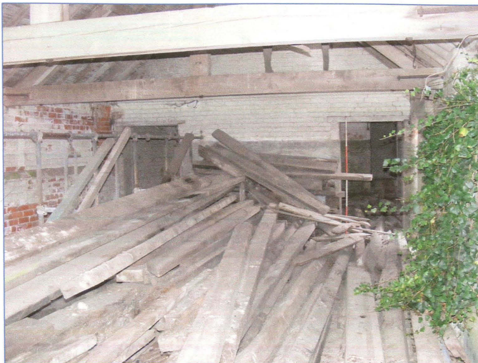
Plate 23 (Shot 25): Interior of Room B2, looking north-north-west from the south-east corner. The steel frame of the milking stalls is visible to the left of the shot, adjacent to a walkway running along the length of the building.
