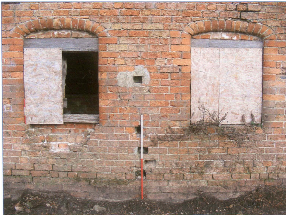
Plate 6 (Shot 14): Detail of basket arch windows in south of elevation of possible stable and granary building (Room A1). Looking north-north-west
