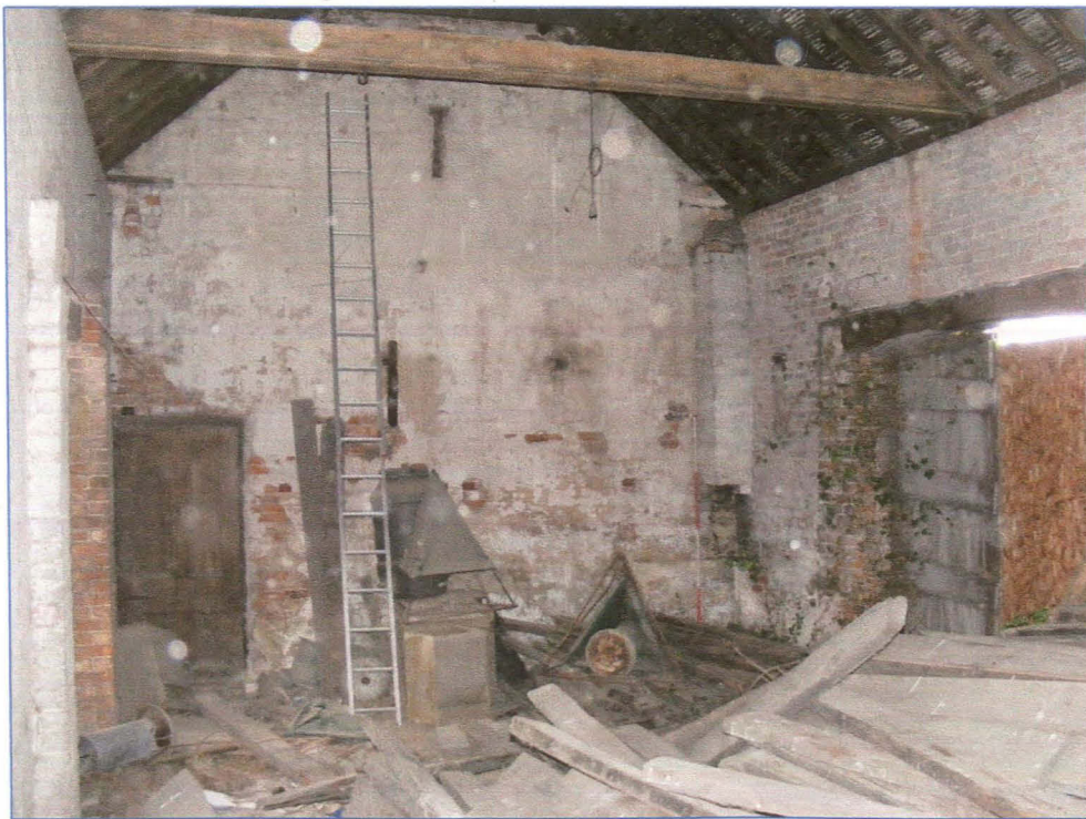
Plate 14 (Shot 30): Interior of threshing barn (A4), looking west from the south-east corner. The chimney is visible in the north-west corner of the building, as well as a blocked ventilation slit above the roof line in the west wall.
