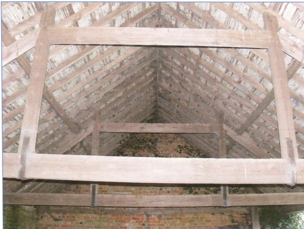
Plate 2 (Shot 3): Roof structure of the cartshed, looking west-north-west
