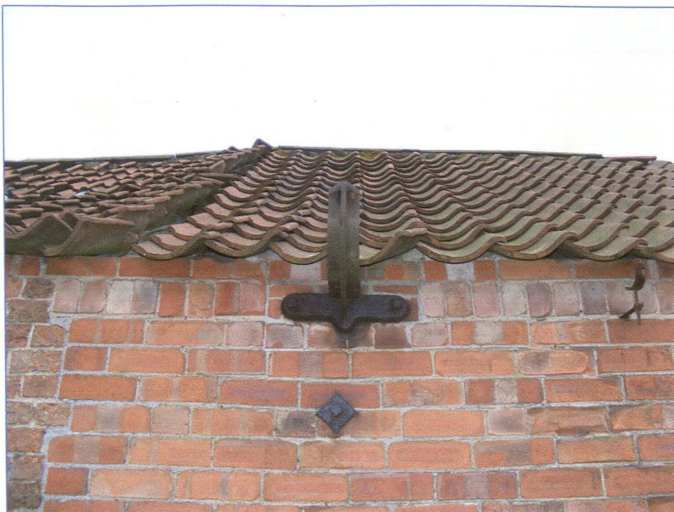
Plate 17 (Shot 44): Detail of cast-iron gutter bracket on west elevation of Block B, looking east-north-east. Another smaller, probably later bracket is visible to the right of shot
