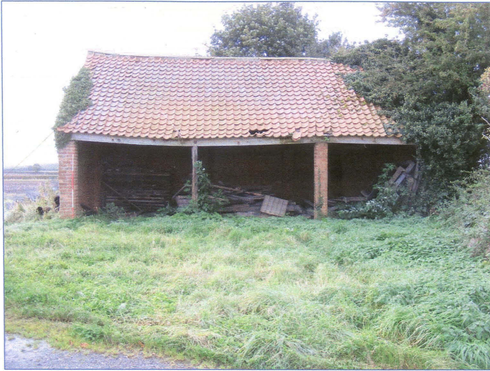
Plate 1 (Shot 1): North elevation of the cartshed, looking south-south-east
