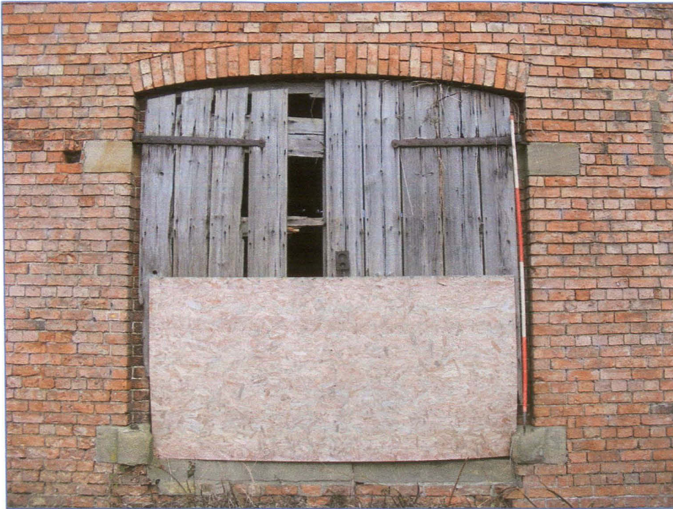
Plate 11 (Shot 18): Double doors in south elevation of threshing barn (A4). The stone mortise blocks are still in situ, and the stone blocks with metal strap hinges are also visible. To the right of the shot is a blocked ventilation slit. Looking north-north-west.
