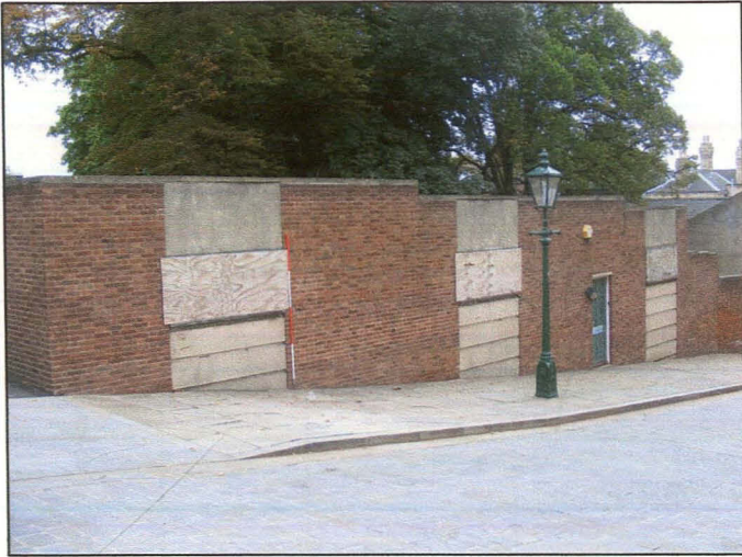
Plate 10 (Shot 11): West elevation of administrative bungalow, looking south-east from Danesgate. This shot illustrates the three levels on which the building has been built, and also shows the banded rustication below the windows
