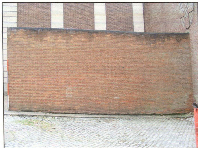
Plate 2 (Shot 3): West elevation of the Coin Gallery, looking east from Danesgate
