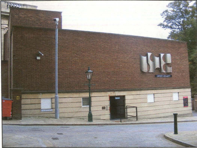
Plate 4 (Shot 4): West elevation of the Curtois Gallery, looking east-north-east. The door allows access to the basement.
