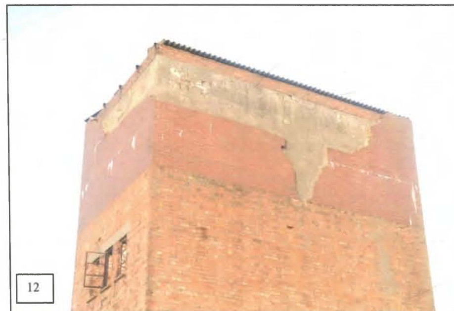
The concrete water tank was clad in a single skin of glazed bricks, giving it a redder colour than the rest of the brickwork. This brick skin had partially fallen away on the south and west sides of the building, but some remedial work had been undertaken in cement to prevent further water penetration.
