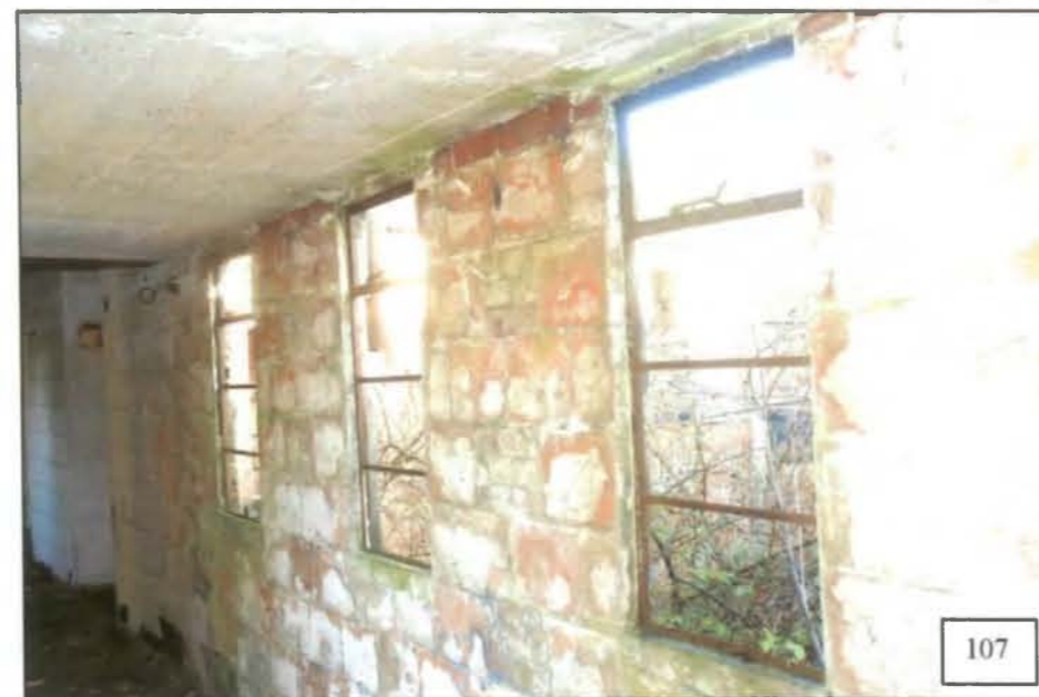
Within each of these porch structures, a pair of double doors (no longer extant) gave access to the linking corridor. On the opposite side of the corridor, a group of three metal-framed four-light windows, the uppermost a top-hung casement, lit the corridor.
