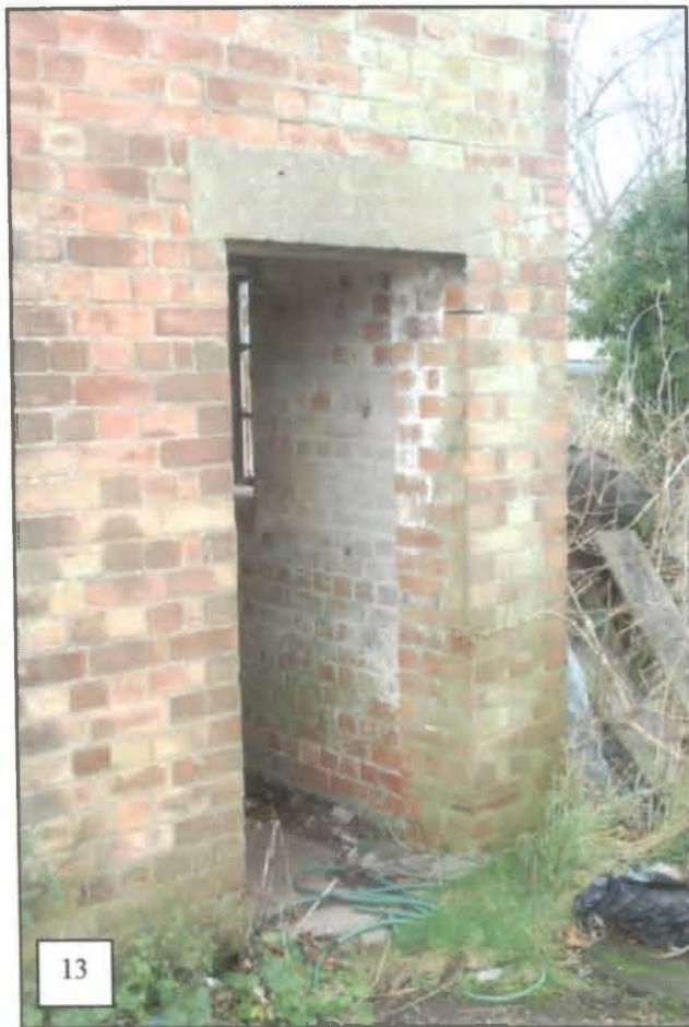
For safety reasons, only the ground floor of the water tower was accessed. The building was accessed through a door opening at the east corner of the south side. The interior was completely whitewashed. It was dominated by three vertical steel pipes: in the northwest and northeast corners these were 3 1/2 " in diameter and did not reach the ground, while the pipe in the southwest corner was 6 1/2 " in diameter and had the words 'Release Valve' painted on it with a downward pointing arrow.
