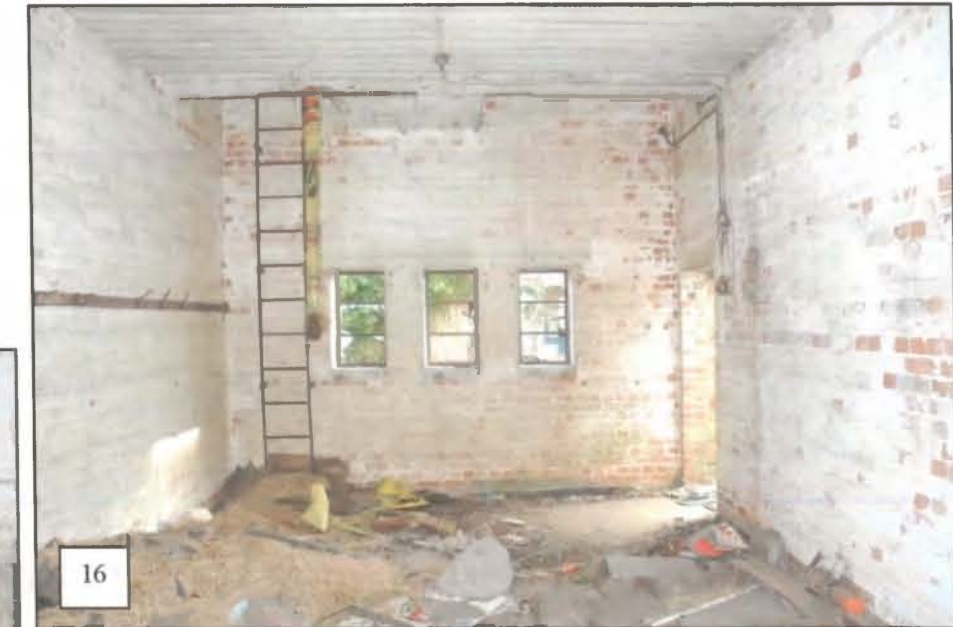
For safety reasons, only the ground floor of the water tower was accessed. The building was accessed through a door opening at the east corner of the south side. The interior was completely whitewashed. It was dominated by three vertical steel pipes: in the northwest and northeast corners these were 3 1/2 " in diameter and did not reach the ground, while the pipe in the southwest corner was 6 1/2 " in diameter and had the words 'Release Valve' painted on it with a downward pointing arrow.
