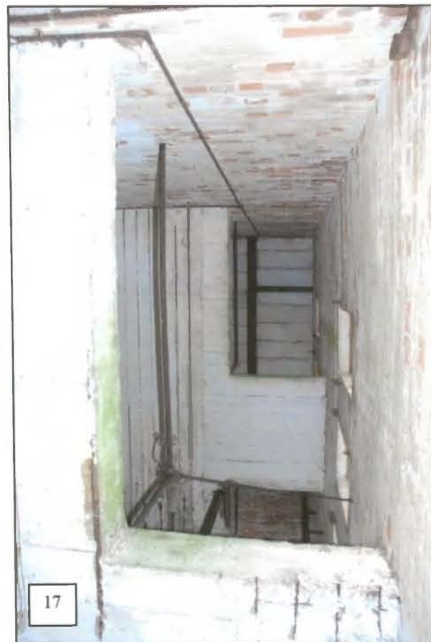
For safety reasons, only the ground floor of the water tower was accessed. The building was accessed through a door opening at the east corner of the south side. The interior was completely whitewashed. It was dominated by three vertical steel pipes: in the northwest and northeast corners these were 3 1/2 " in diameter and did not reach the ground, while the pipe in the southwest corner was 6 1/2 " in diameter and had the words 'Release Valve' painted on it with a downward pointing arrow.
