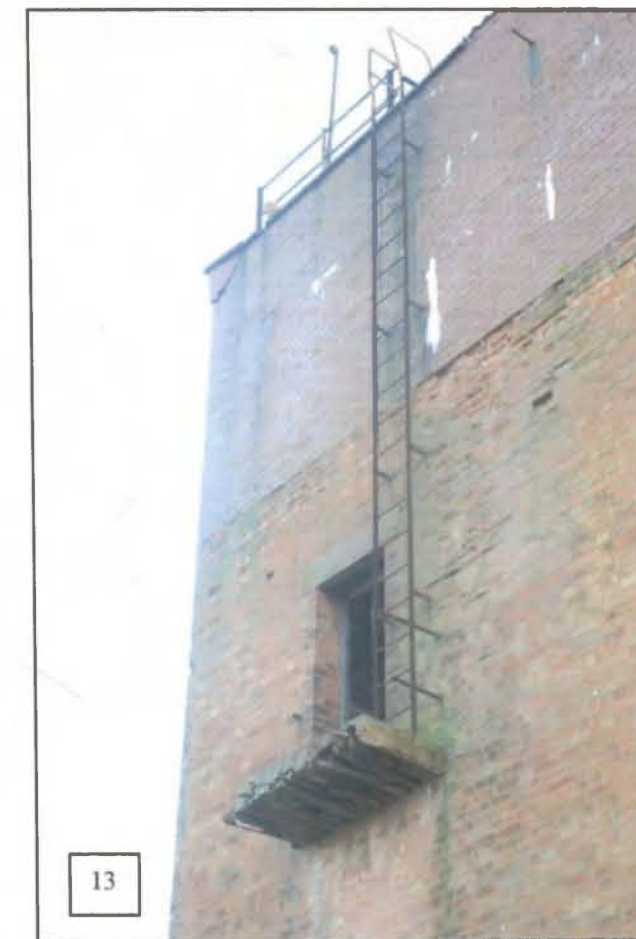
The concrete water tank was clad in a single skin of glazed bricks, giving it a redder colour than the rest of the brickwork. This brick skin had partially fallen away on the south and west sides of the building, but some remedial work had been undertaken in cement to prevent further water penetration.
