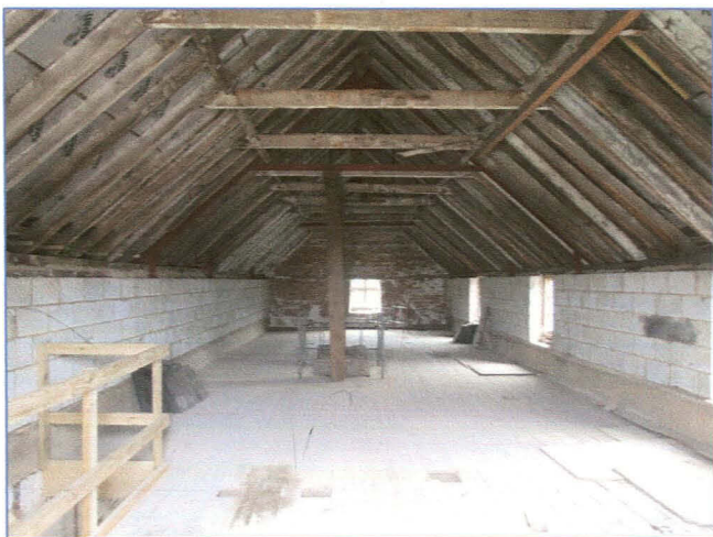
Plate 12: Second floor, looking south
