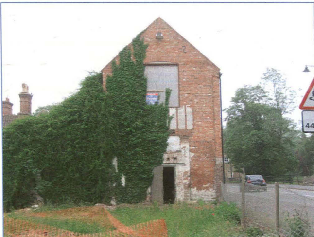
Plate 5: North elevation, looking south
