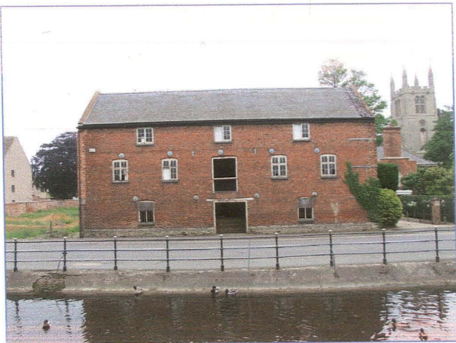
Plate 2: West elevation, looking east.
