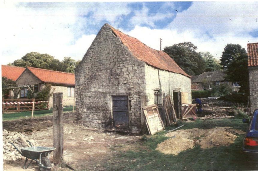
Plate 5 - View of the barns from the southwest
