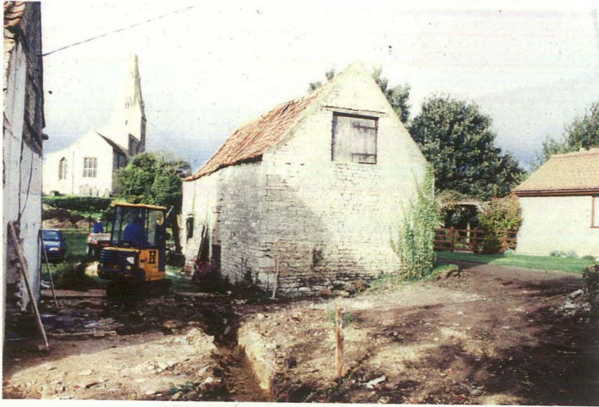
Plate 1 - View of the development, looking west
