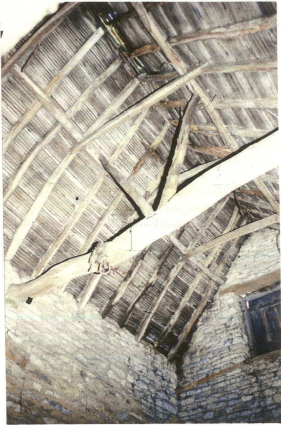
Plate 6 - View showing roof trusses in the eastern barn
