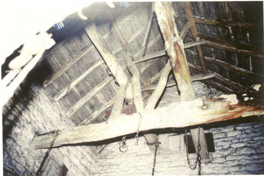
Plate 7 - View showing the roof trusses in the western barn
