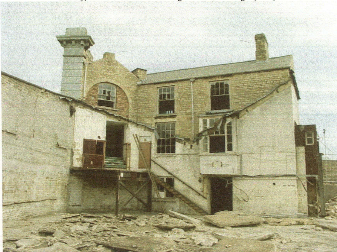
Pl. 3 Exterior of frontage building, looking NE. The diagonal arch is part of the original 1845 iron foundry, with later additional buildings attached to the right (south)
