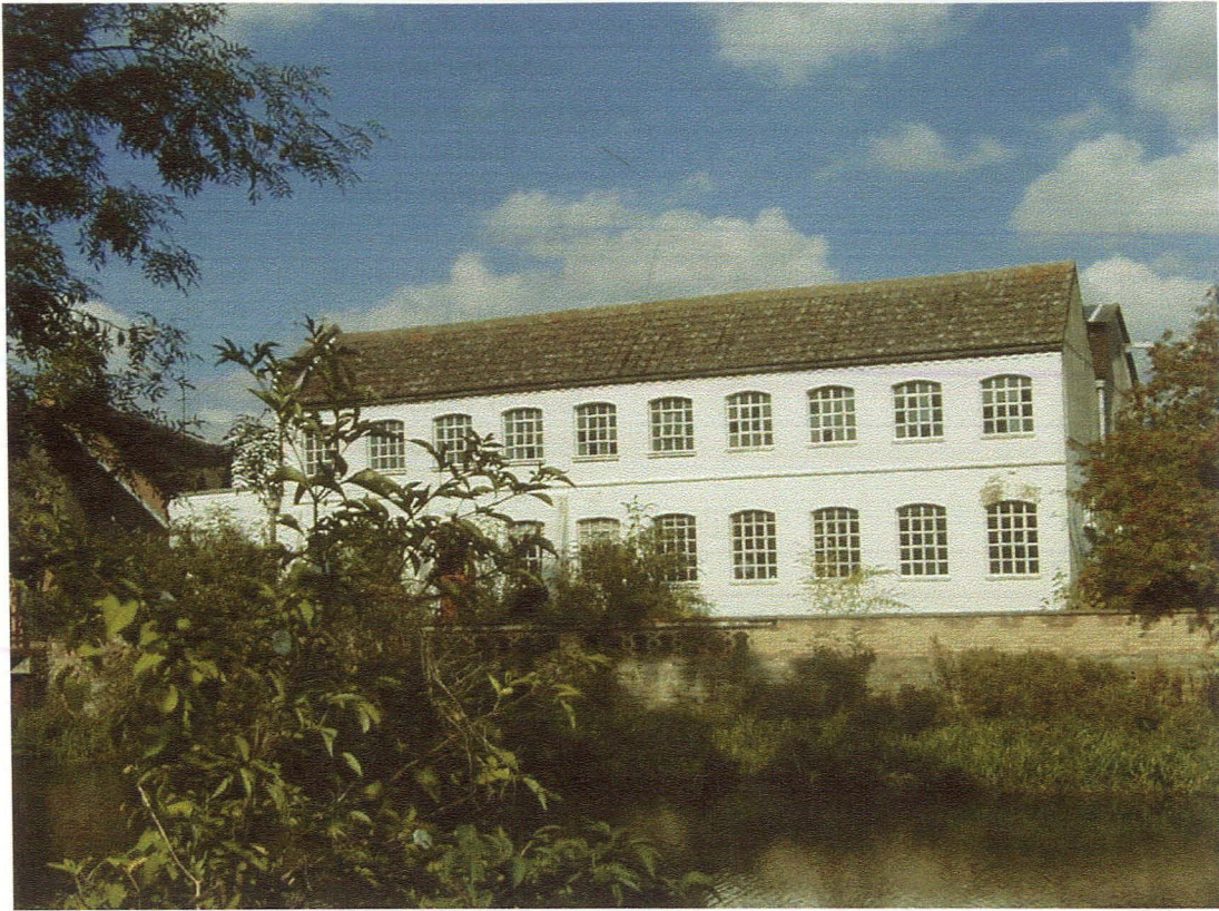
Pl. 2 Exterior of 1902 Stamford Electric Light Company building, looking N, also shows Blashfield terracotta balustrade
