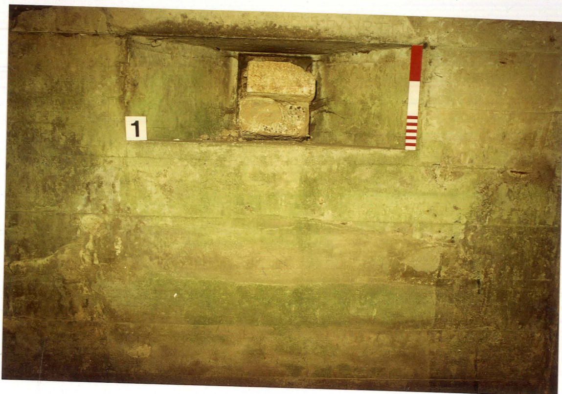
Pl. 18 Blocked gun embrasure, pillbox 1. Scale 0.3m.
