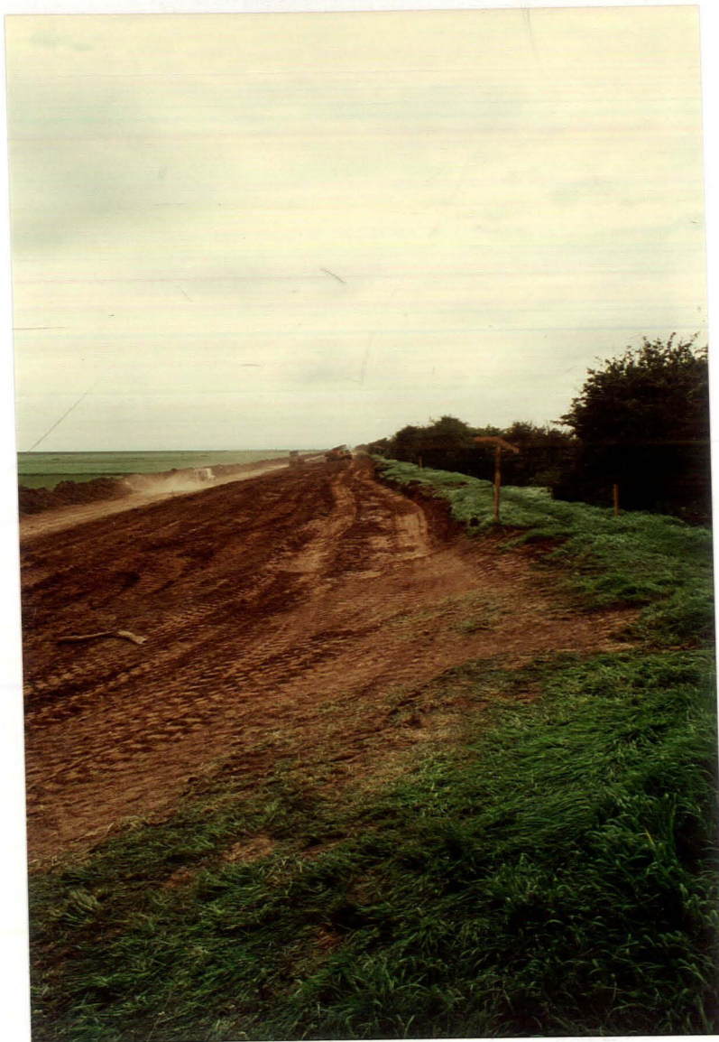
Pl. 9 Topsoil-stripping and reinforcement of the 1809 floodbank (looking west).
