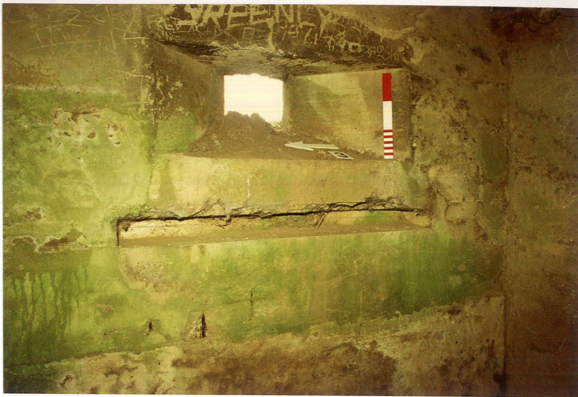
Pl. 26 Gun embrasure in the east wall of the southern room, pillbox 3. Scale 0.3m.
