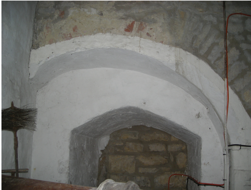
Plate 4 Recess cut through arcade in boiler room
