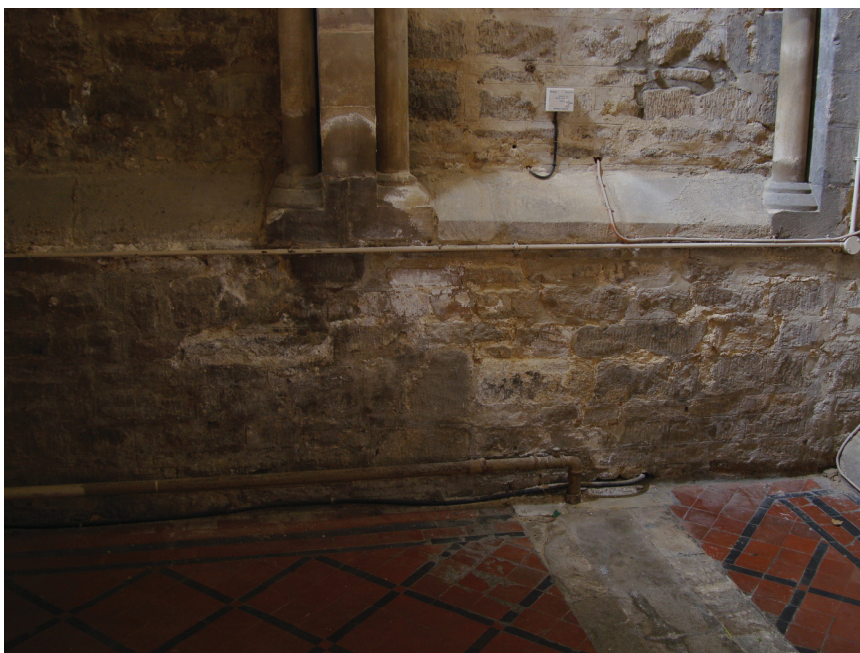
Plate 3 Detail of lower part of arcade, showing inserted chamfered sill and straight join
