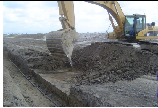
Figure 1 Machine removing overburden on north side of trench
