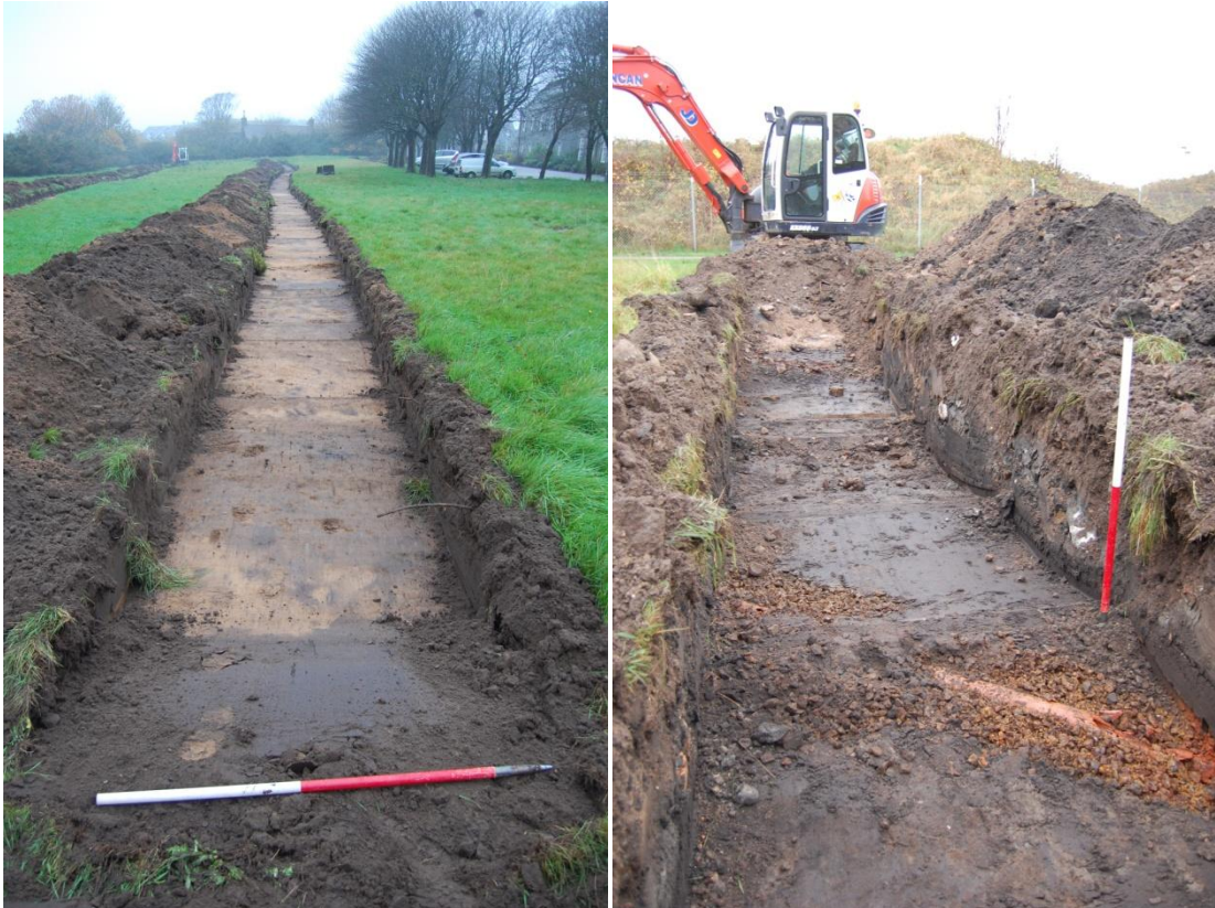
Ill 5 Trench 2 showing sand natural (left; facing W), Trench 4 showing ceramic land drain F3 (right; facing W)
