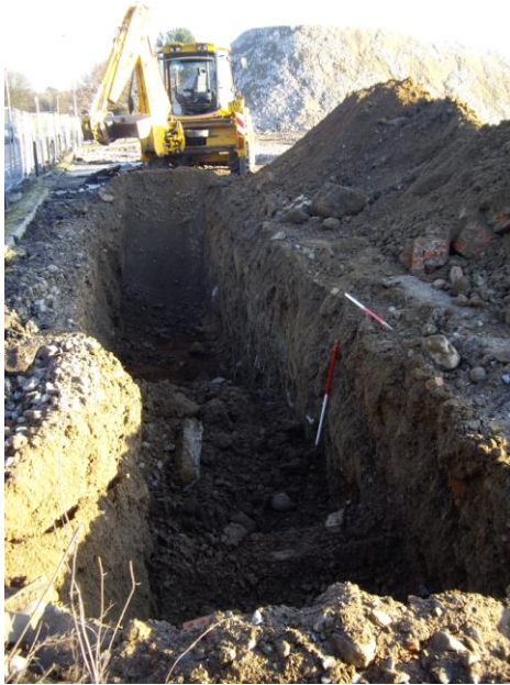
III 3 Photograph showing Trench 1, facing north-east
