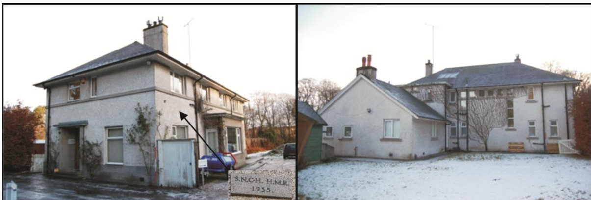
Figure 30 Area N2 Moir House (F63) from SW (left) from N (right)
