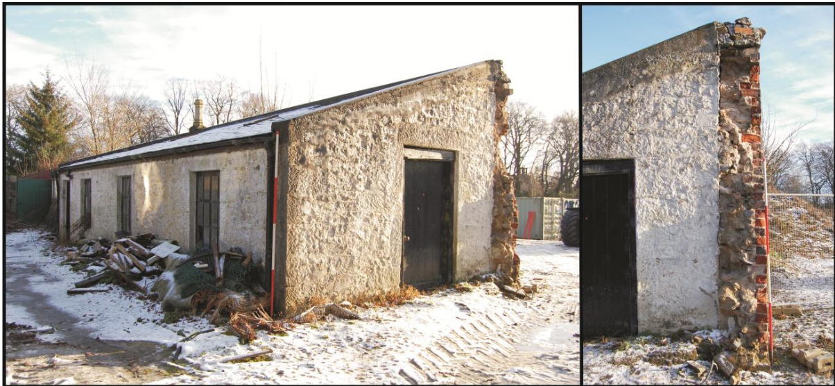
Figure 32 Area N2 Gardeners lean-to F59 (left) and detail of attachment to N garden wall F61 (right)
