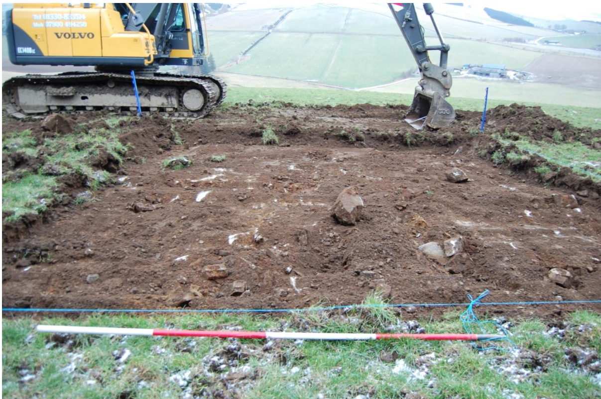
Illus 5 Trench for wind turbine, facing south-west
