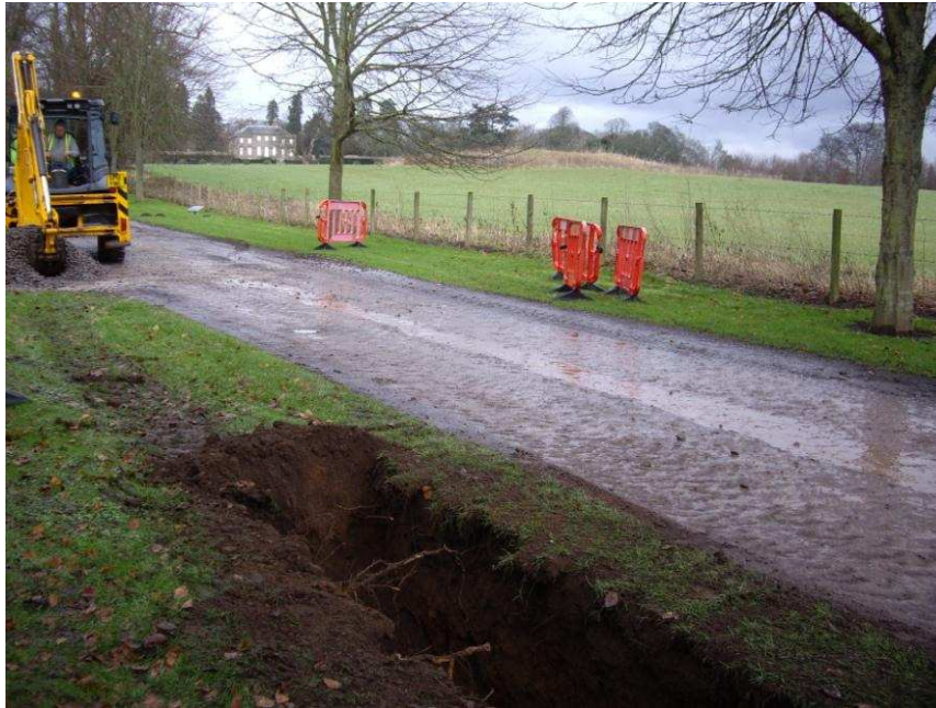
Illus 4 Trench 1 under excavation
