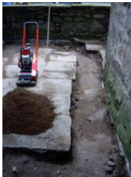
Illus 5: Backfilled Trench 2, facing south-east
