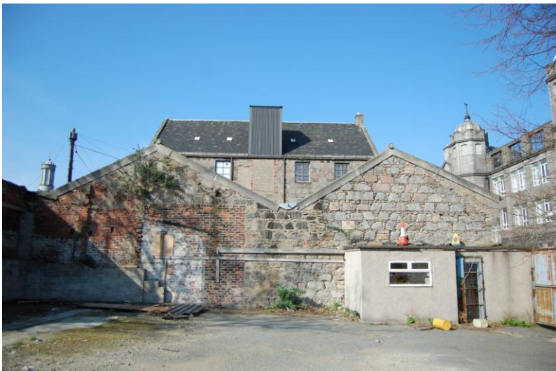
Illus 8 B5 East face of east extension
