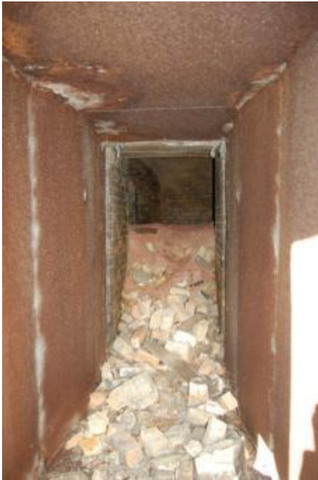
Illus 30 Vent between Boiler House B10 and chimney B11
