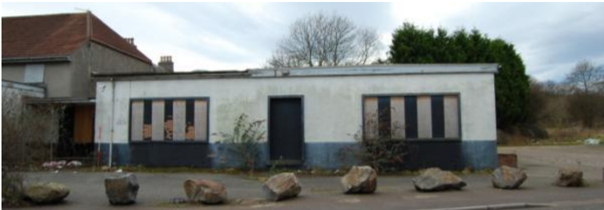
Illus 31 Building 16 from NE
