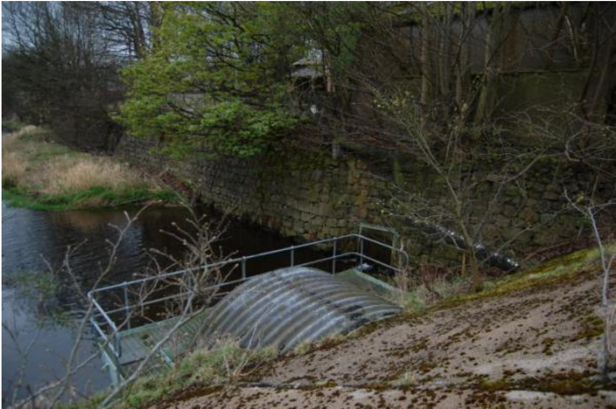
Illus 38 Lade 3 (centre) showing 23m wide lade feeding water back into the river Don and Lade L2 outflow (centre at base of stone embankment)
