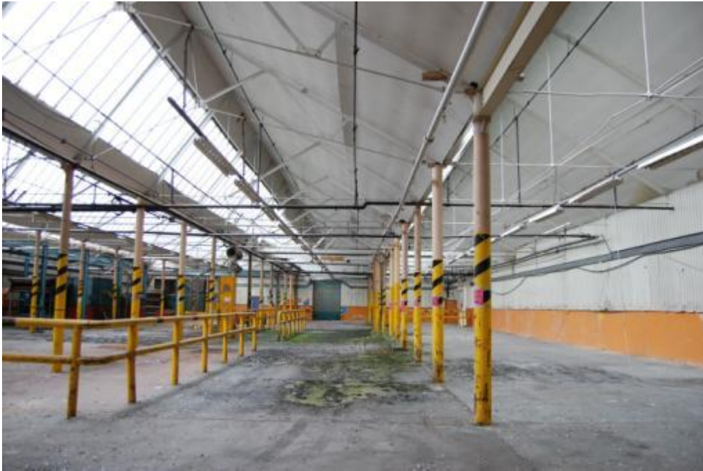
Illus 16 Interior of Building 4 facing east showing cast iron support pillars
