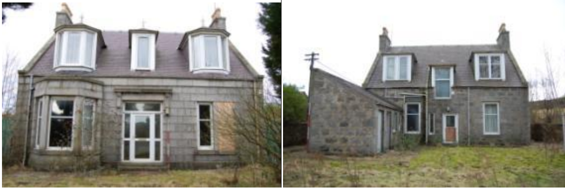
Illus 32 Building B17 (left) front SE facade; (right) rear NW face
