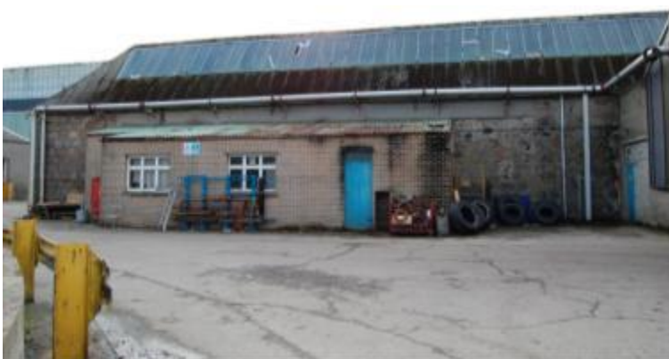
Illus 19 Building 5: North wall showing extension 5b.
