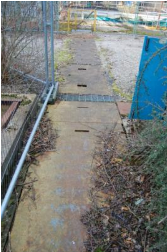
Illus 40 Culvert (L7) facing west
