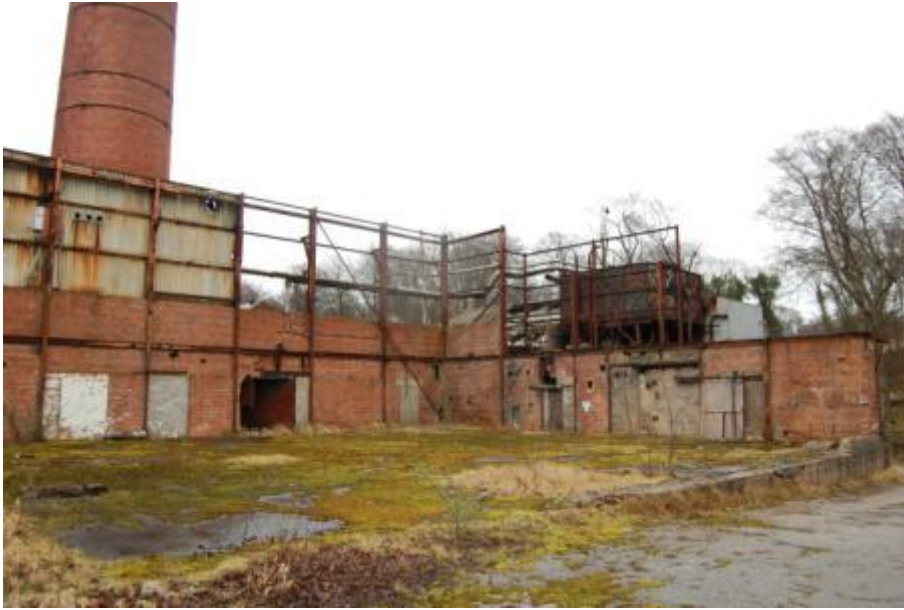
Illus 26 Chimney (B11) with B10 (foreground); facing NNW
