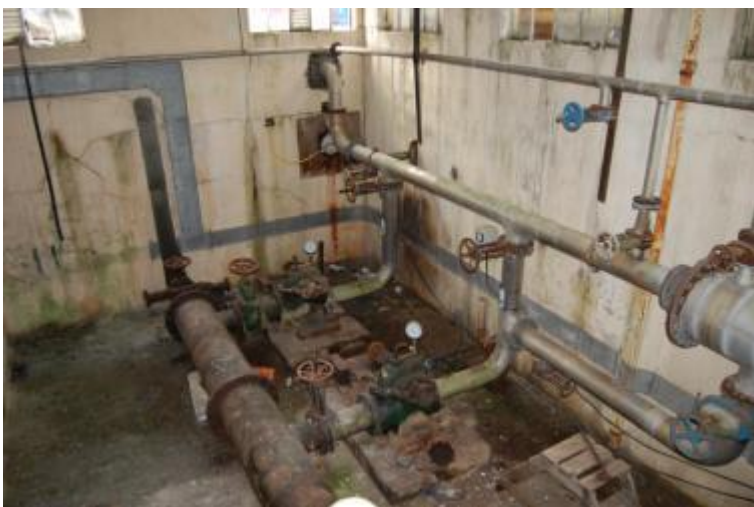
Illus 21 Building 6a pumping plant with mechanisms still in situ
