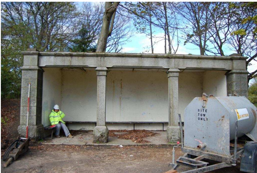
Illus 12 Stone shelter east facade; facing west
