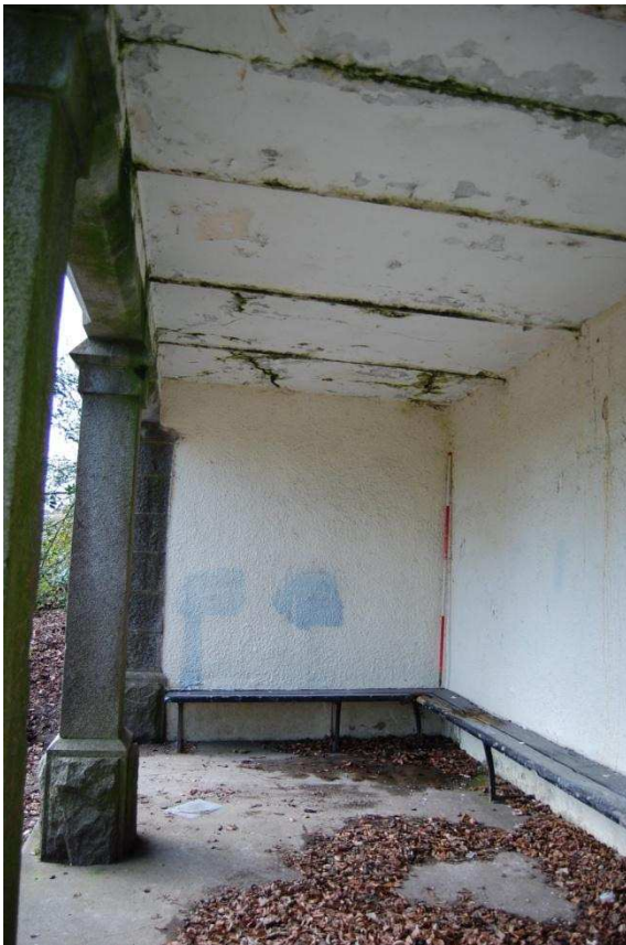
Illus 14 Stone shelter interior, facing south
