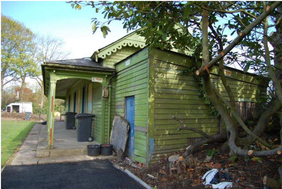
Illus 6 Pavilion facing SE
