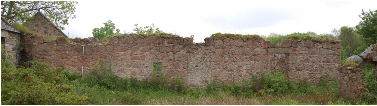
Illus 19 NW elevation of south wing showing wall junction F7 (left)
