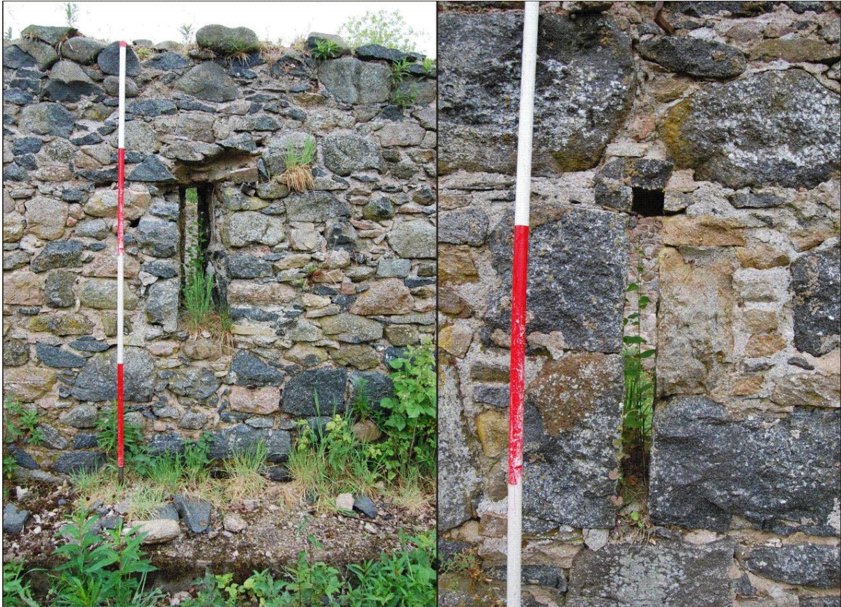
Illus 10 Window 11 interior (left) and exterior (right)
