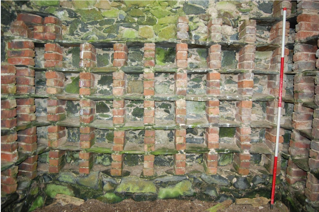
Illus 5 Brick and stone slate nesting boxes on the interior of the east wall
