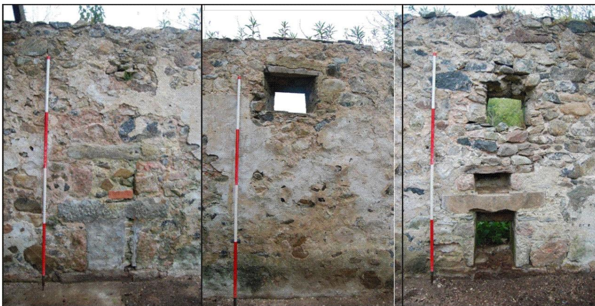
Illus 17 (left) Aperture 1 (top) 2 (bottom); (middle) Aperture 3 (right) Aperture 4 (above) 5 (centre) and 6 (below) with fine-grained sandstone lintel
