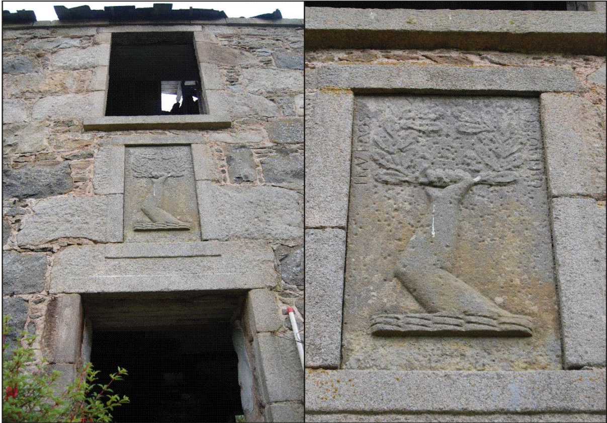
Illus 15 Room 6 Door 20 with Window 13 (above) and sandstone plaque
