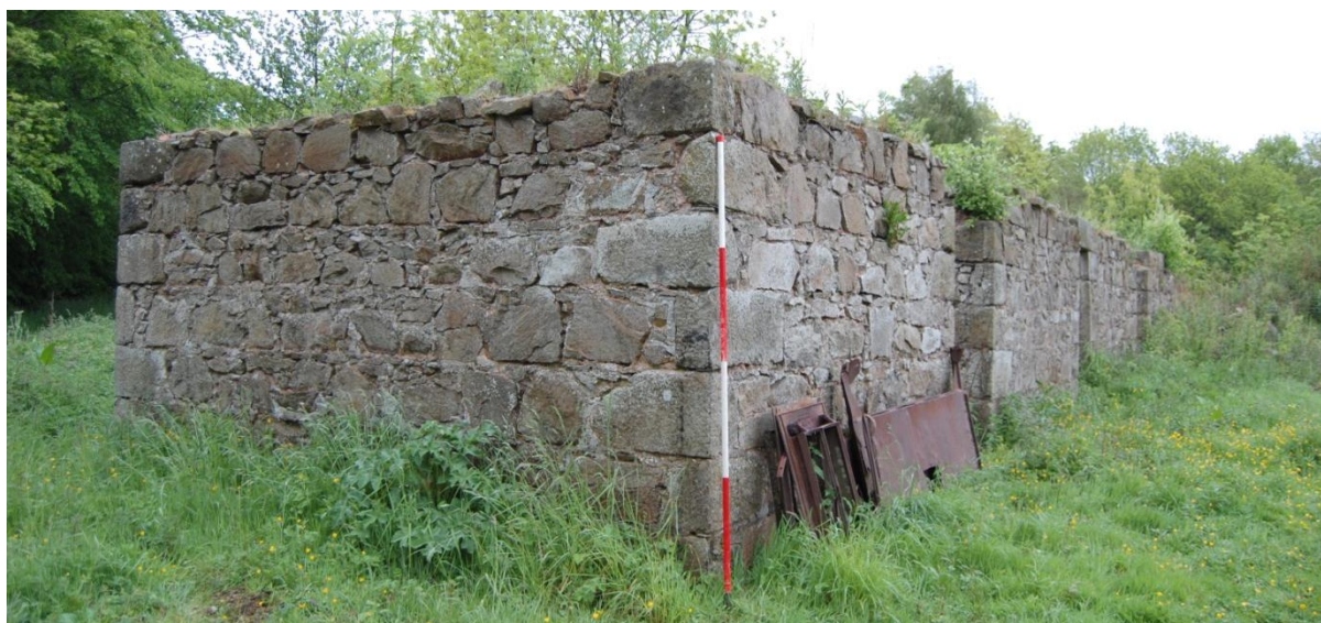
Illus 26 Room 1 (foreground), Room 2, Room 3
