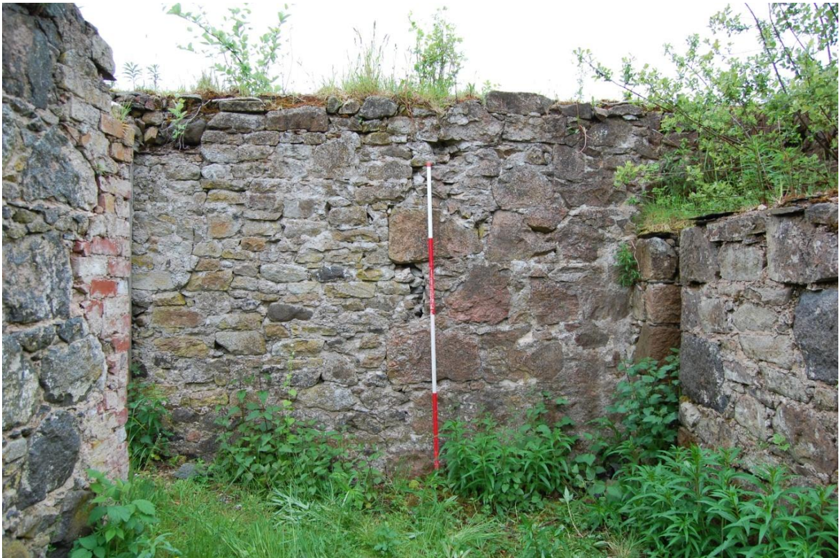
Illus 12 Room 4 south wall scar F6 between the pink quartz-rich granite (right) and grey granite fieldstones (left)
