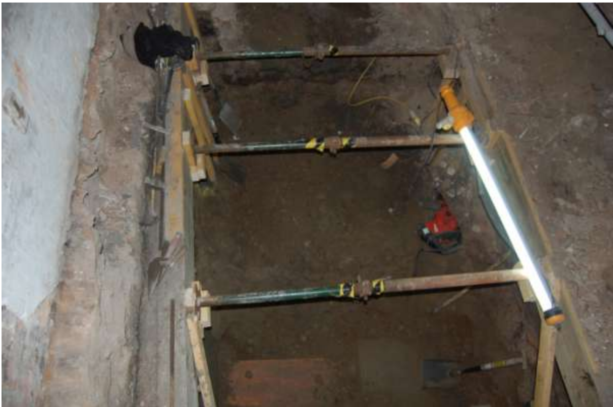
Illus 6 Trench for new lift shaft
