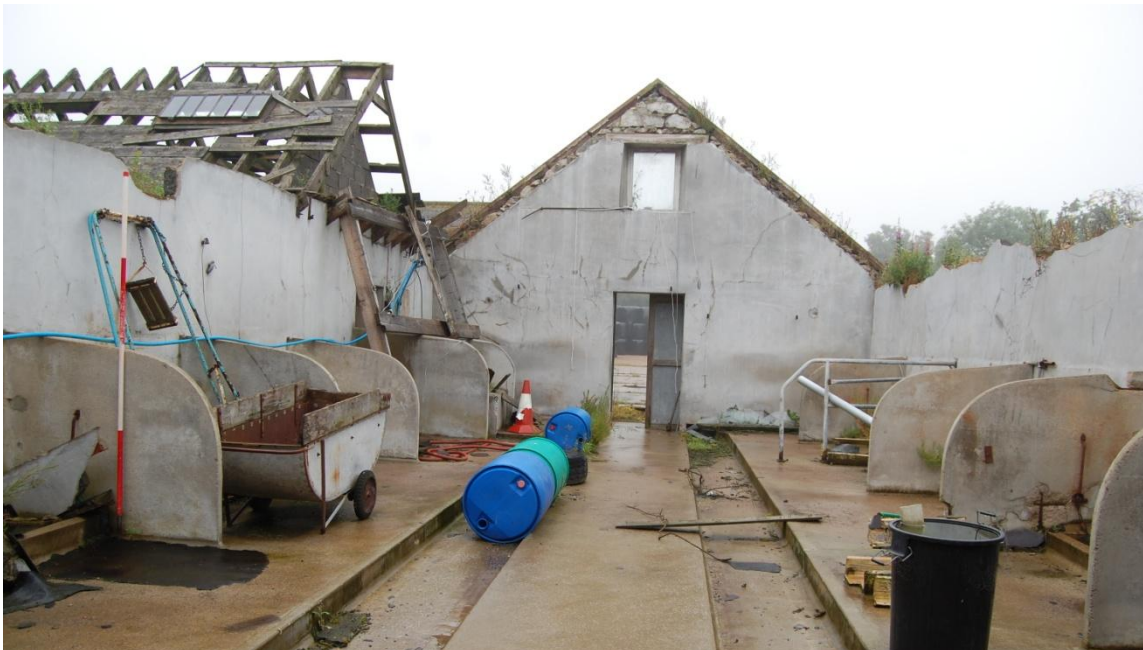
Illus 5 Room 1 showing reinforced concrete partitions, facing north
