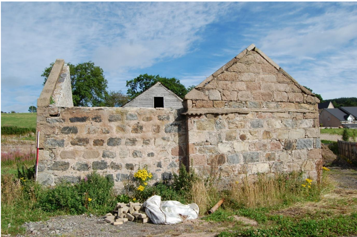
Illus 6 Phase 1 gable (left) constructed of large pink granite blocks, and Phase 2 (left). The Phase 1 gable had a door (F6) which was blocked in Phase 2
